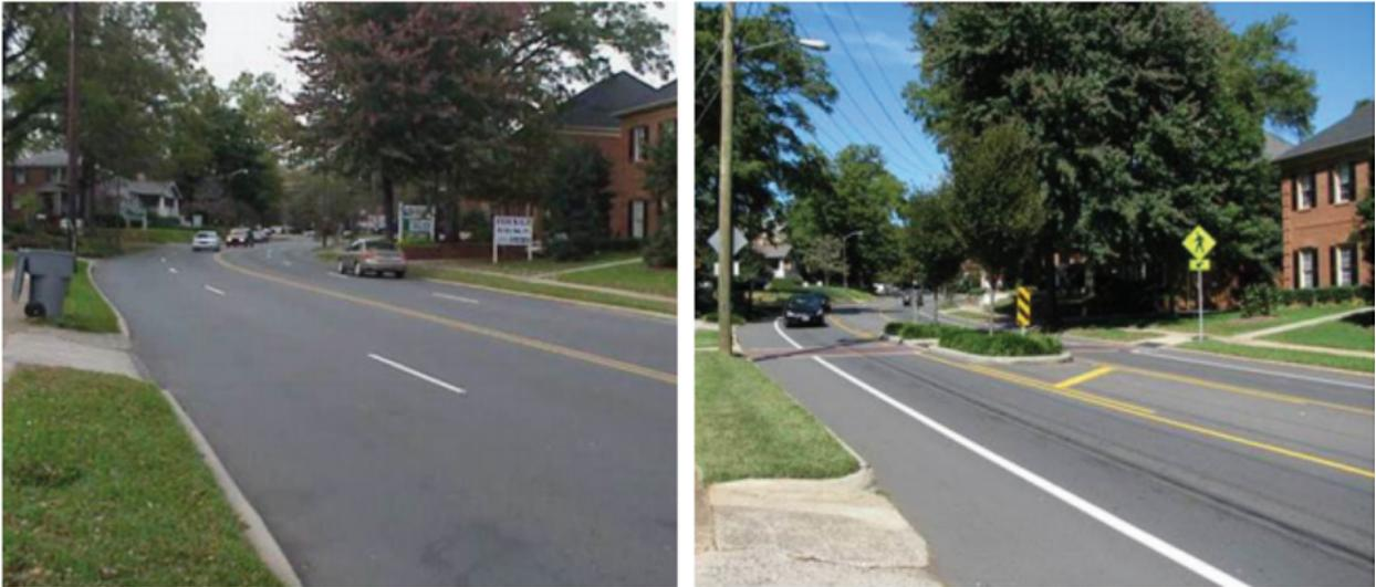
**Figure 5-3** Four-lane road in Charlotte, NC, changed to three-lane road with median turn lane to create space for bicycle lanes (Photos: Ken Tippette)
