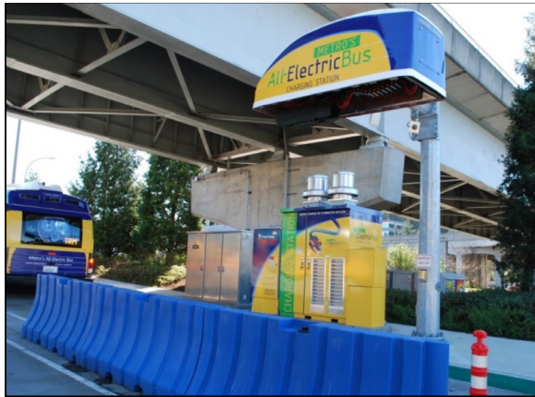
Figure 3-6 Fast-Charge Station at KC Metro Park-and- Ride
