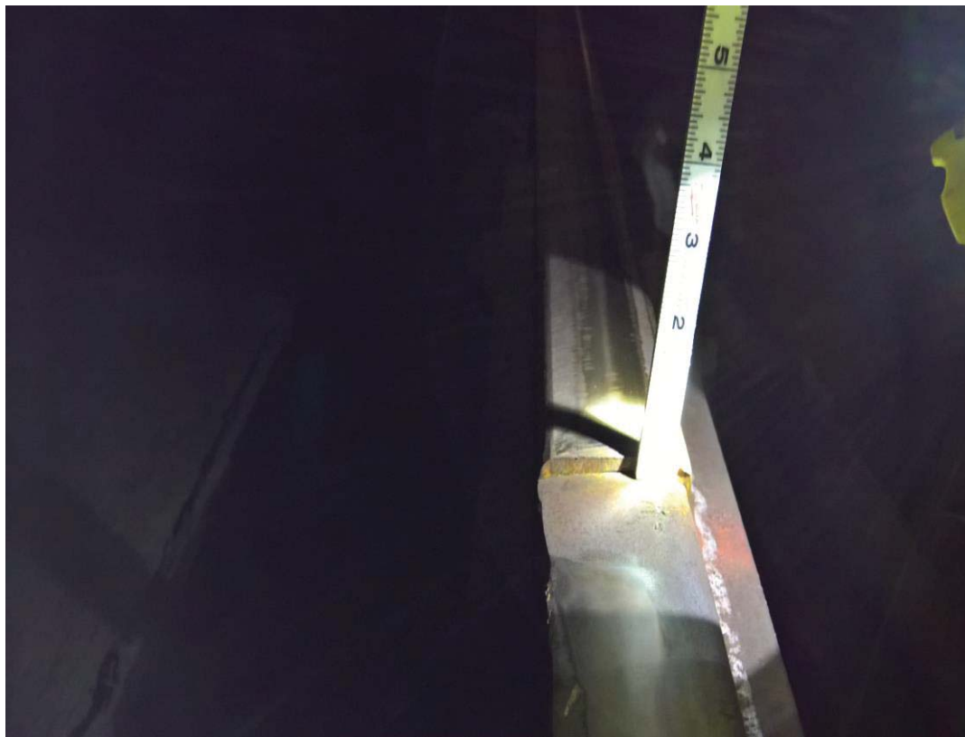
Photo 1: A2 232+75 tread mismatch measuring 3/16-inches.
