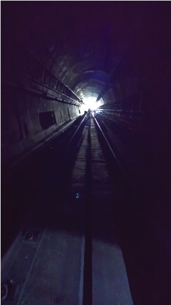
Figures 1 and 2: No working tunnel lights between B1 480+25 and working limits. The on-track equipment was providing the only lighting for workers.
