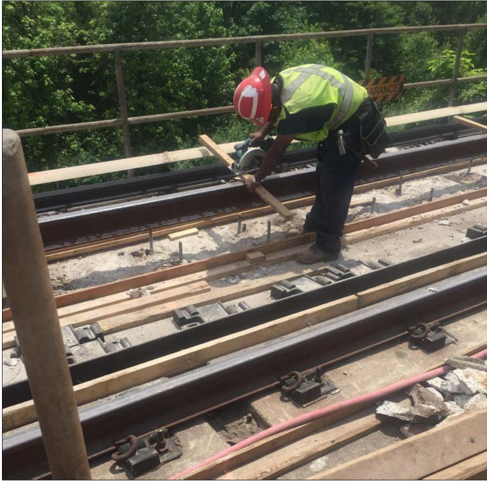
Surge 15 – Building forms for new grout pads between Cheverly and Landover Stations
