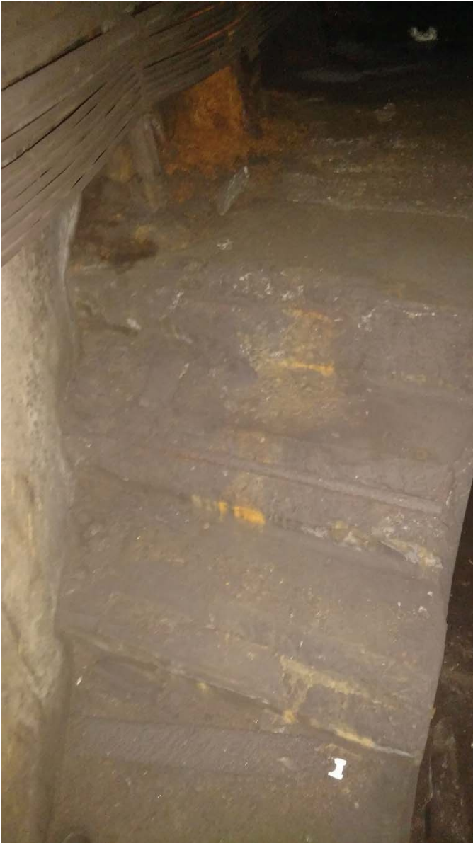
Figure 1: Safety Walk Stairs. Note exposed rebar, crumbled step and displaced step edge.
