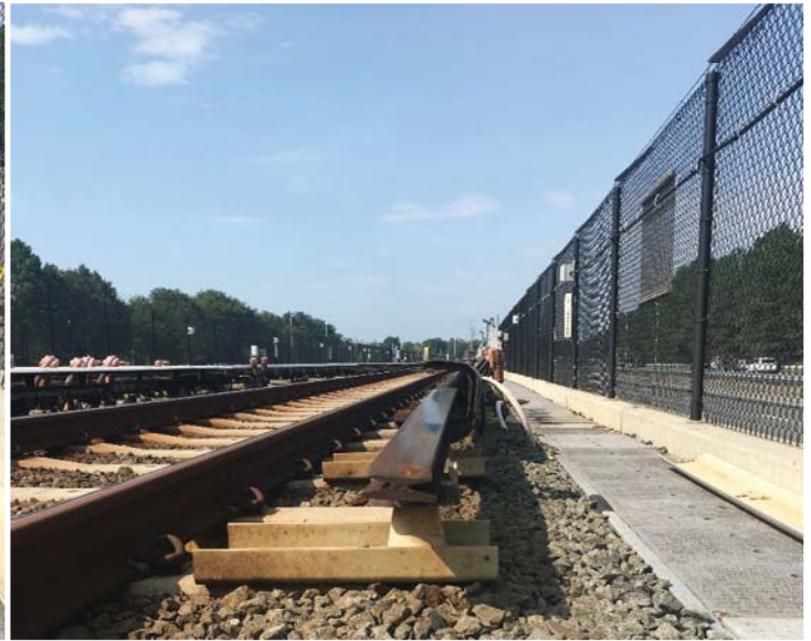
Figures 1 and 2: Missing cover board, evidence of collector shoes striking the nose of the end approach, and misaligned end approach at N2 1006+70.
