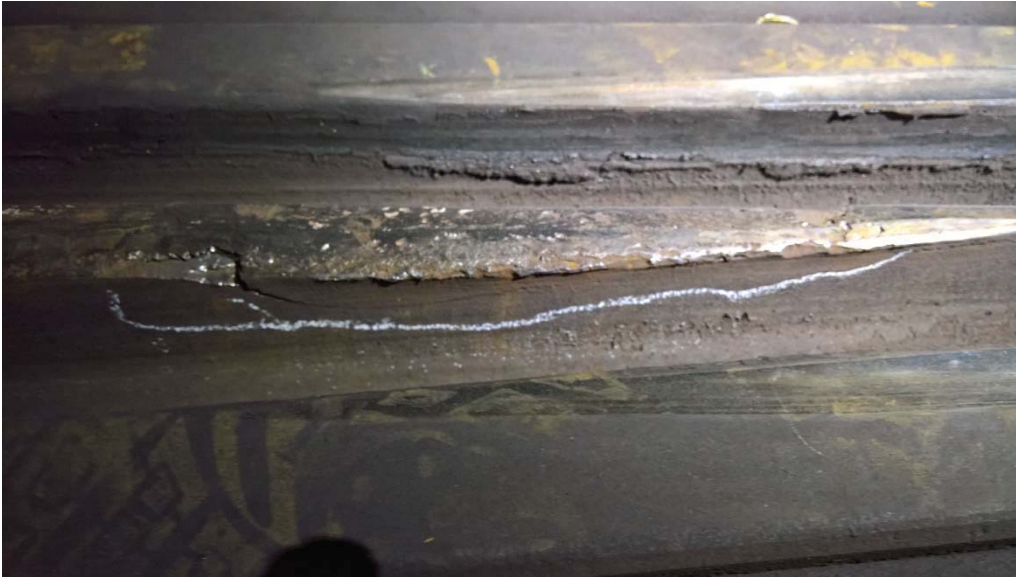
Figure 1: Cracked frog point at switch #3.
