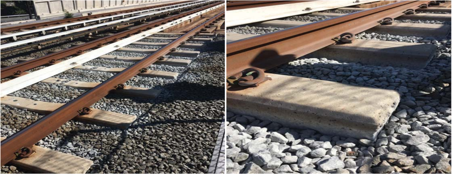
Figures 1 & 2: Churned ballast at the location with a 1 ½" uniform profile deviation. Ballast indents on the sides of the concrete crossties indicate the amount of dynamic movement under loaded operations.
