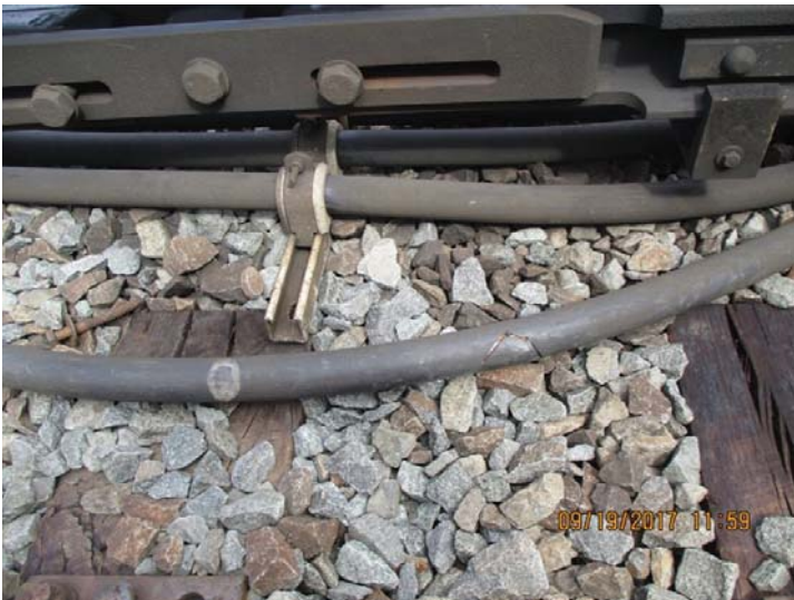
Figure 1: J1 607+00 - Expansion cable damaged and on gauge side of the third rail.
