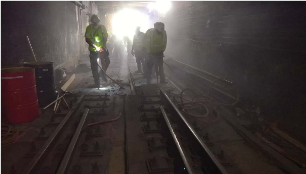
Figure 4: WMATA personnel demolishing grout pads.
