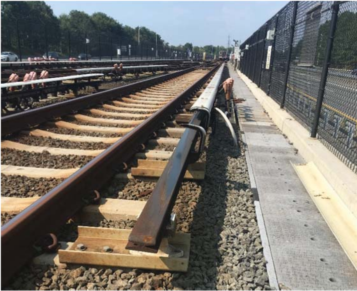
Figures 1 and 2: Missing cover board, evidence of collector shoes striking the nose of the end approach, and misaligned end approach at N2 1006+70.
