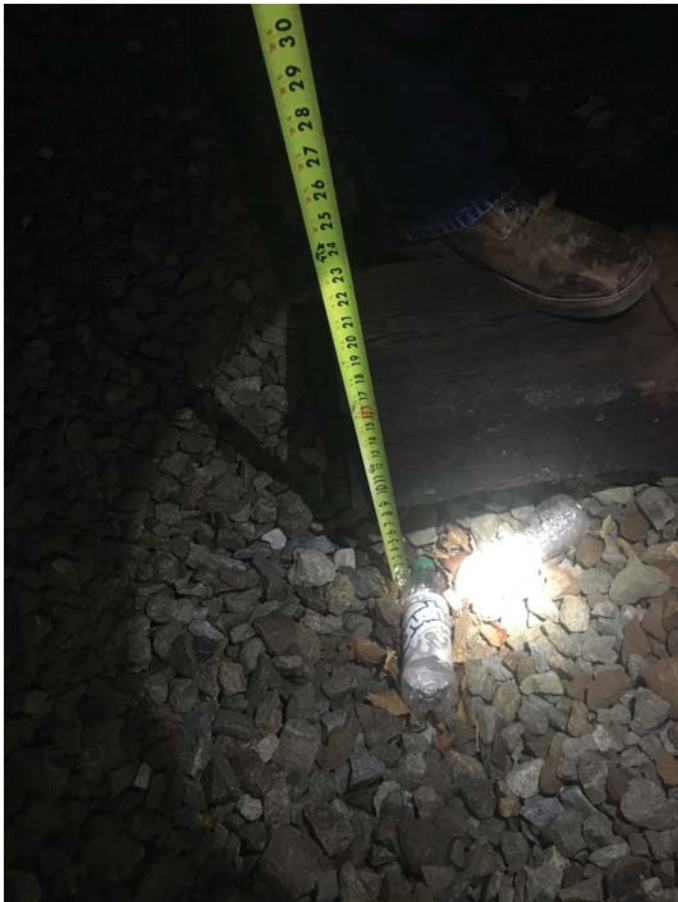
Figure 1: Low ballast condition at right rail tie end at C2 411+50. Ballast 8 inches below tie end.
