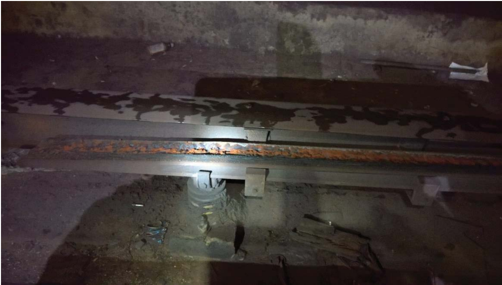
Figure 2: Wear on end approach at D2 45+00.
