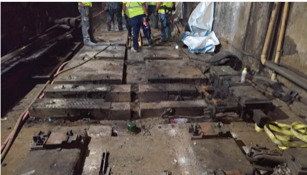
Figure 3: Switch components removed from switch #3.
