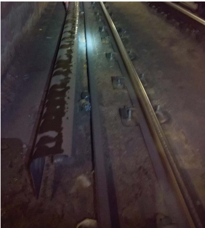
Figure 1: Relay rail stored between running rail and third rail between D2 43+06 and 43+60.
