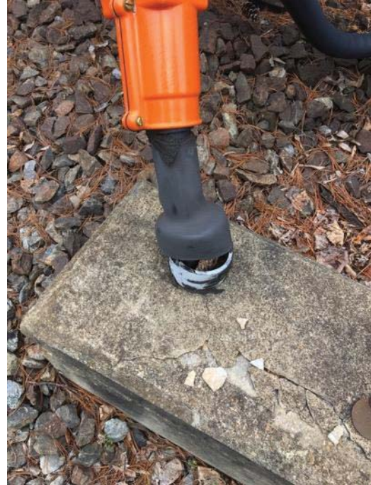
FIGURE 2 - YCR 16B – HEAT SHRINK ON CONDUIT STUB-UP COMPROMISED
