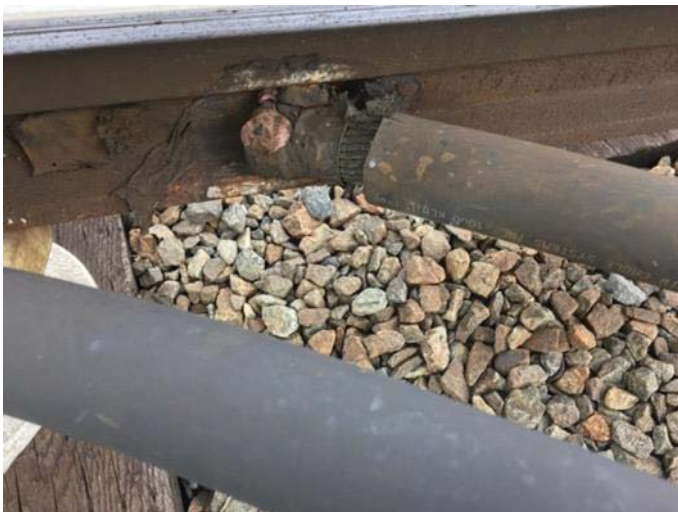
FIGURE 9 - YCR 69 – PIGTAIL CADWELD COMPROMISED TO STEEL 3RD RAIL
