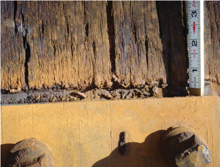
Figure 2 - Lateral Track Movement - 1/2" of plate movement.
