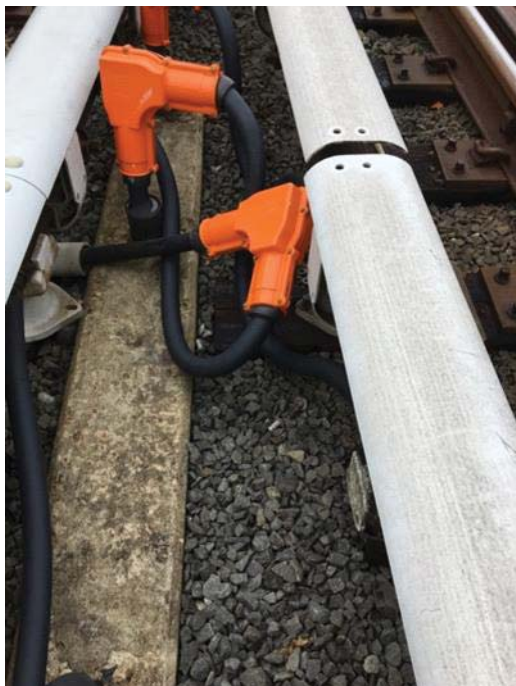
FIGURE 13 - YCR 6 –ORANGE BOOT POWER ASSEMBLY TOO CLOSE TO KICKER 3RD RAIL
