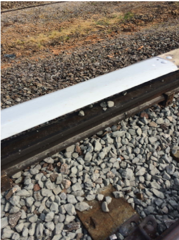
Photo 4: Ballast piled up against the third rail seen in work zone.
