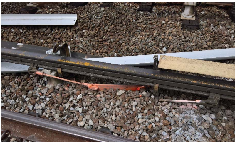
Photo 3: Example of a third rail anchor not reinstalled.
