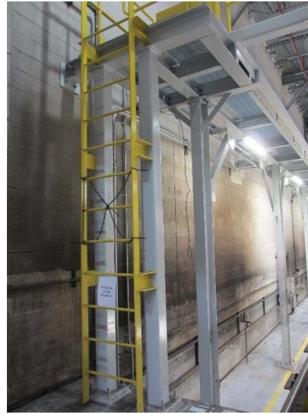
Figure 6: Safety has posted a sign and placed chain to prevent access.
