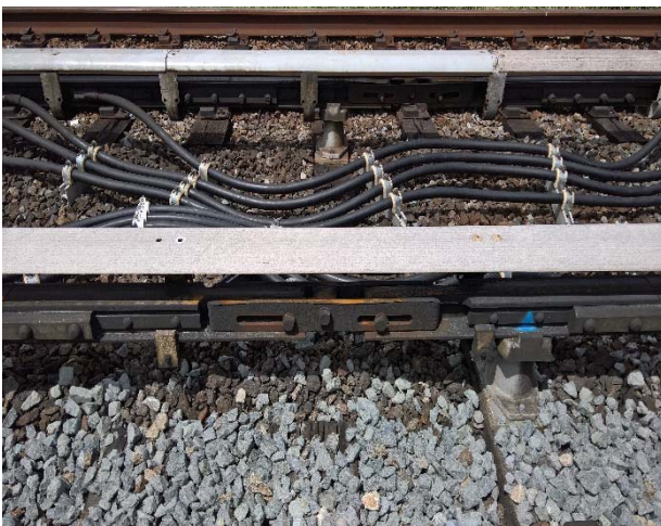
Photo 2: Example of a third rail expansion joint not adjusted properly.
