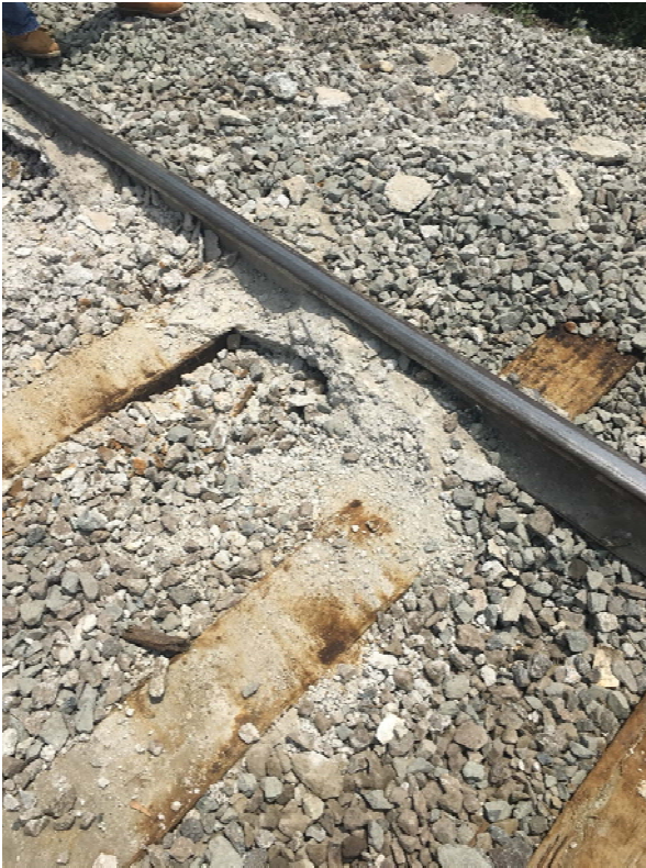
Photo 1: Grout on running rail at D1 414+00.
