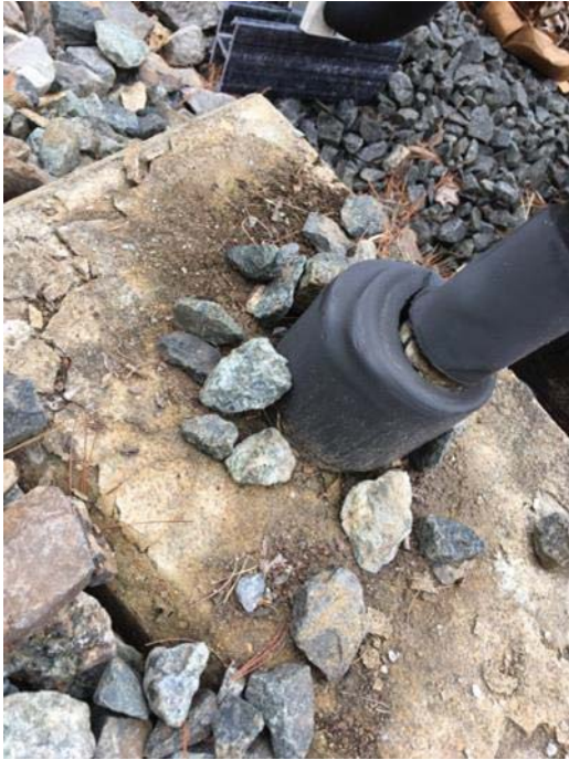
FIGURE 3 - YCR 13 – HEAT SHRINK ON CONDUIT STUB-UP COMPROMISED
