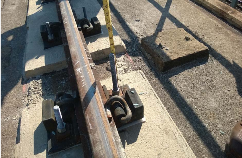
Photo 1: Studs exceed the allowable 3 inch (TRST 1000).
