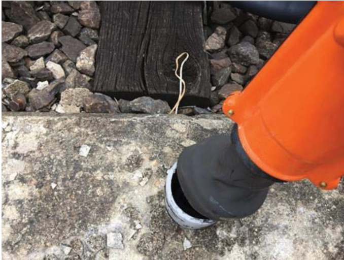
FIGURE 7 - YCR 7 – HEAT SHRINK ON CONDUIT STUB-UP COMPROMISED
