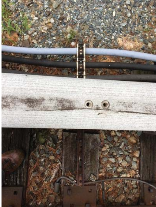
FIGURE 1 - YARD CONTACT RAIL (YCR) 17D – METAL KINDORF STRUCTURE RATHER THAN EMI APPROVED FIBERGLASS KINDORF STANDING CABLES OFF THE GROUND. METAL STRUCTURE ON GAUGE SIDE OF 3RD RAIL
