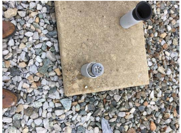
FIGURE 12 - YCR 3 – CAP UNUSED CONDUIT PROPERLY
