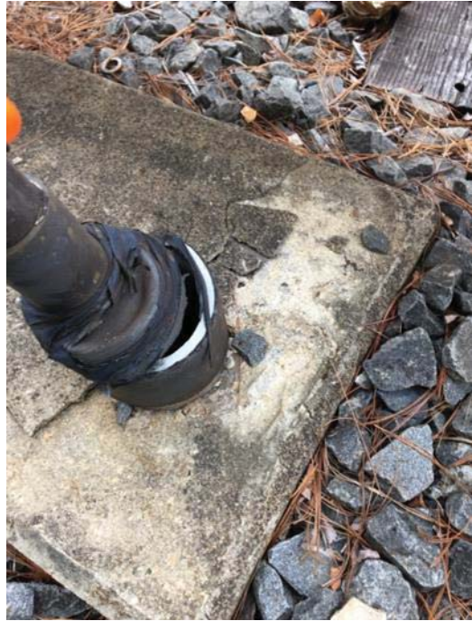
FIGURE 4 - YCR 12 – HEAT SHRINK ON CONDUIT STUB-UP COMPROMISED
