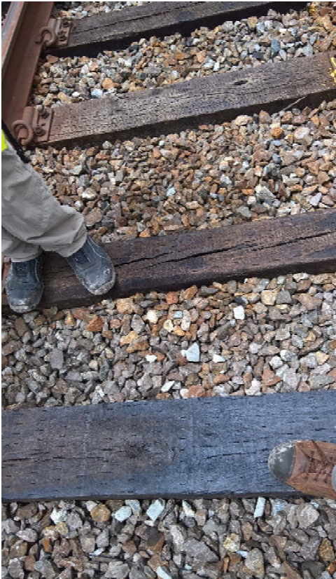
Photo 4: Example of tie spacing between the Rockville and Twinbrook Stations on track 2. The cross tie spacings were inconsistent, ranging from 22 - 36 inches.
