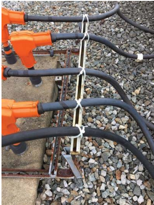
FIGURE 11 – YCR 3 - FEEDER CABLES STOOD OFF THE GROUND WITH METAL KINDORF STRUCTURE AND ZIP TIES
