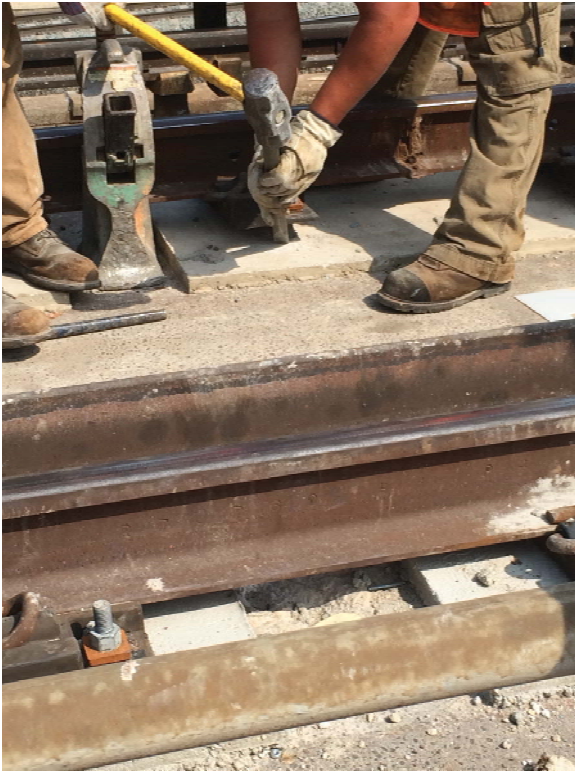
Photo 5: Hammer and chisel technique being used to provide uniform surface under fastener.
