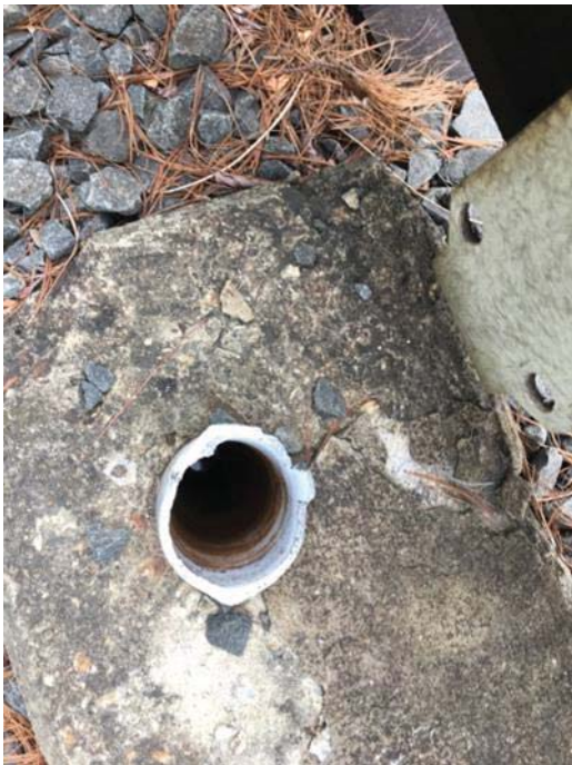
FIGURE 5 - YCR 12 – CAP UNUSED CONDUIT
