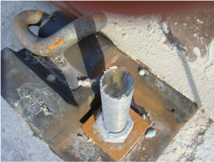
Figure 3 - Newly installed stud bolt on New Carrollton aerial, track 2.
