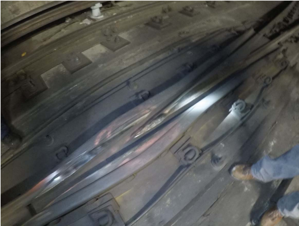
Photo 1: Battered frog point at C2 65+00.
