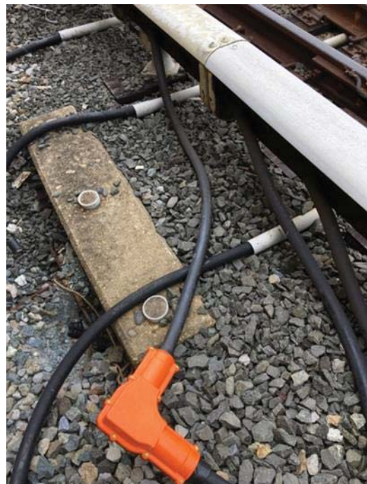
FIGURE 14 - YCR 4 – ORANGE BOOT POWER ASSEMBLY LYING ON THE BALLAST
