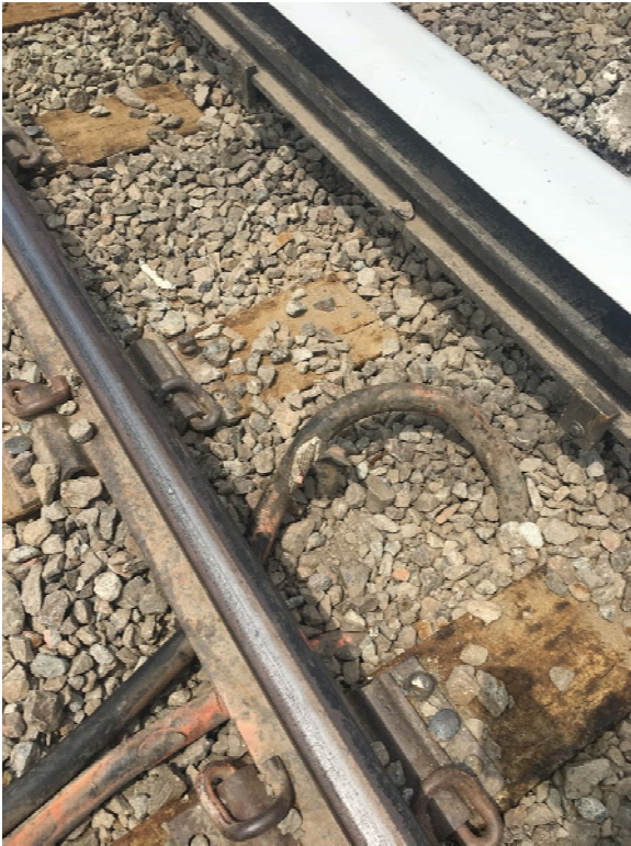
Photo 3: Example of damaged negative return cable seen in work zone.
