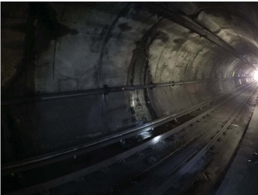
Photo 2: Tunnel leak at C2 107+00.
