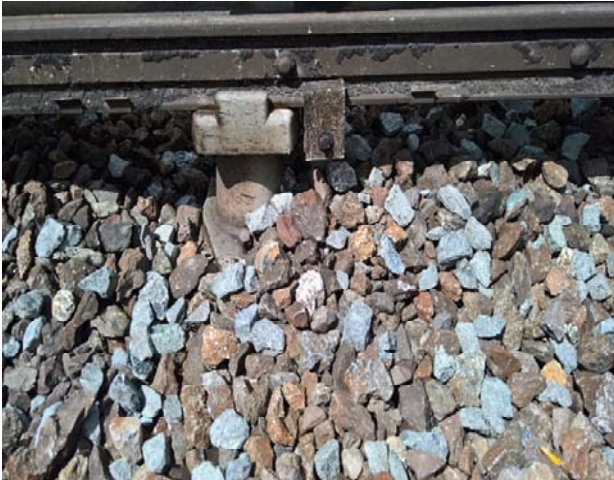
Photo 1: Example of a third rail bracket installed too close to the third rail pedestal.
