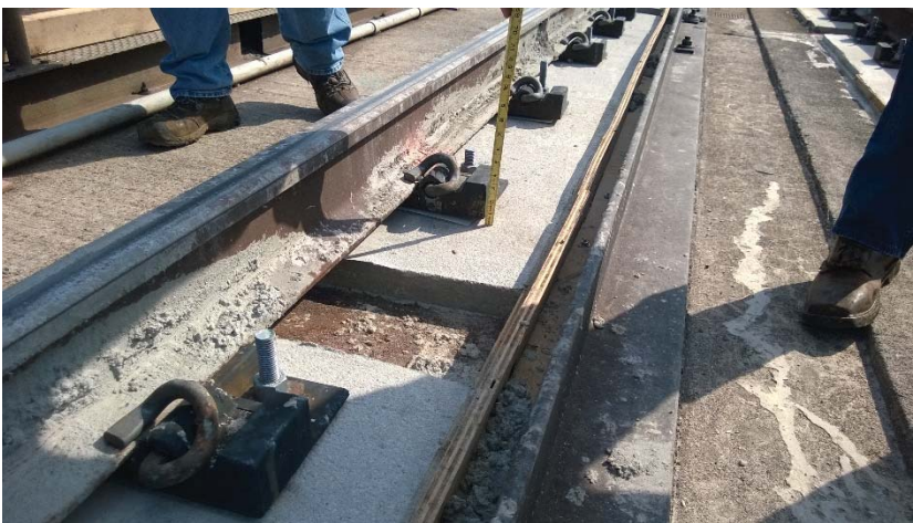
Photo 2: Elastic fasteners not seated to the grout pad.
