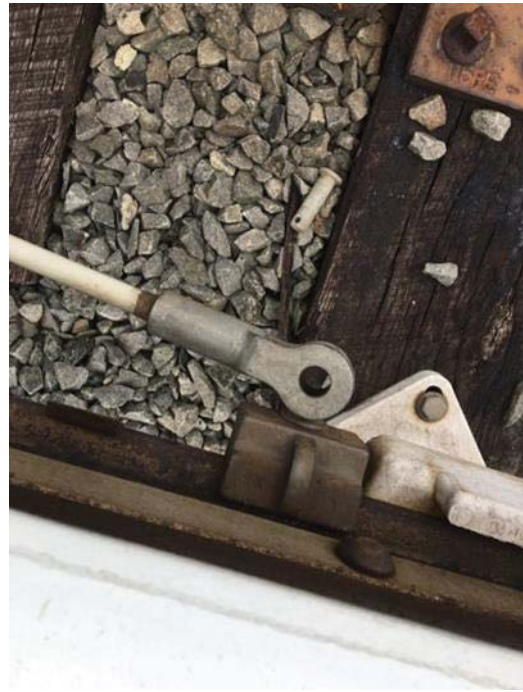
FIGURE 8 - YCR 70 – 3RD RAIL TIE ANCHOR MISSING BOLT
