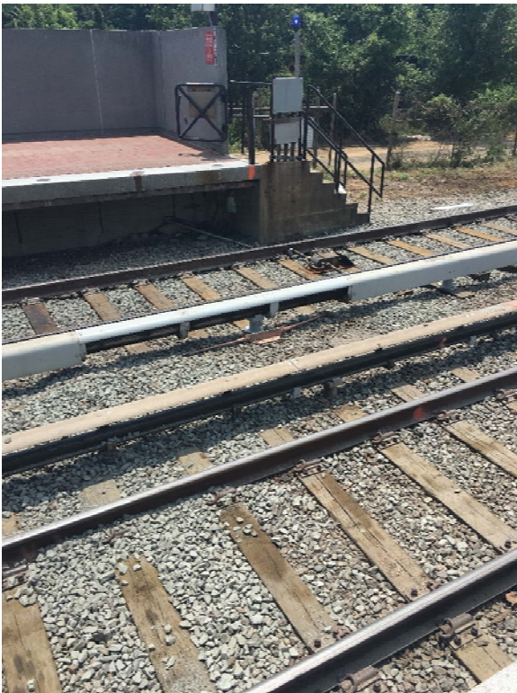
Photo 2: Unsecured third rail anchor arm at D1 420+00
