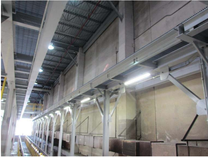
Figure 5: New platform; note lack of railing.
