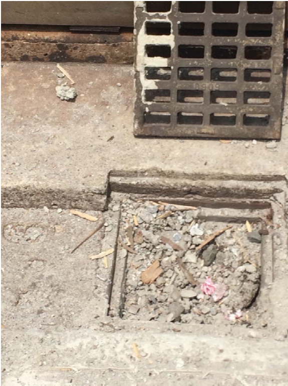
Photo 7: Example of clogged drains seen on aerial structure in work zone.
