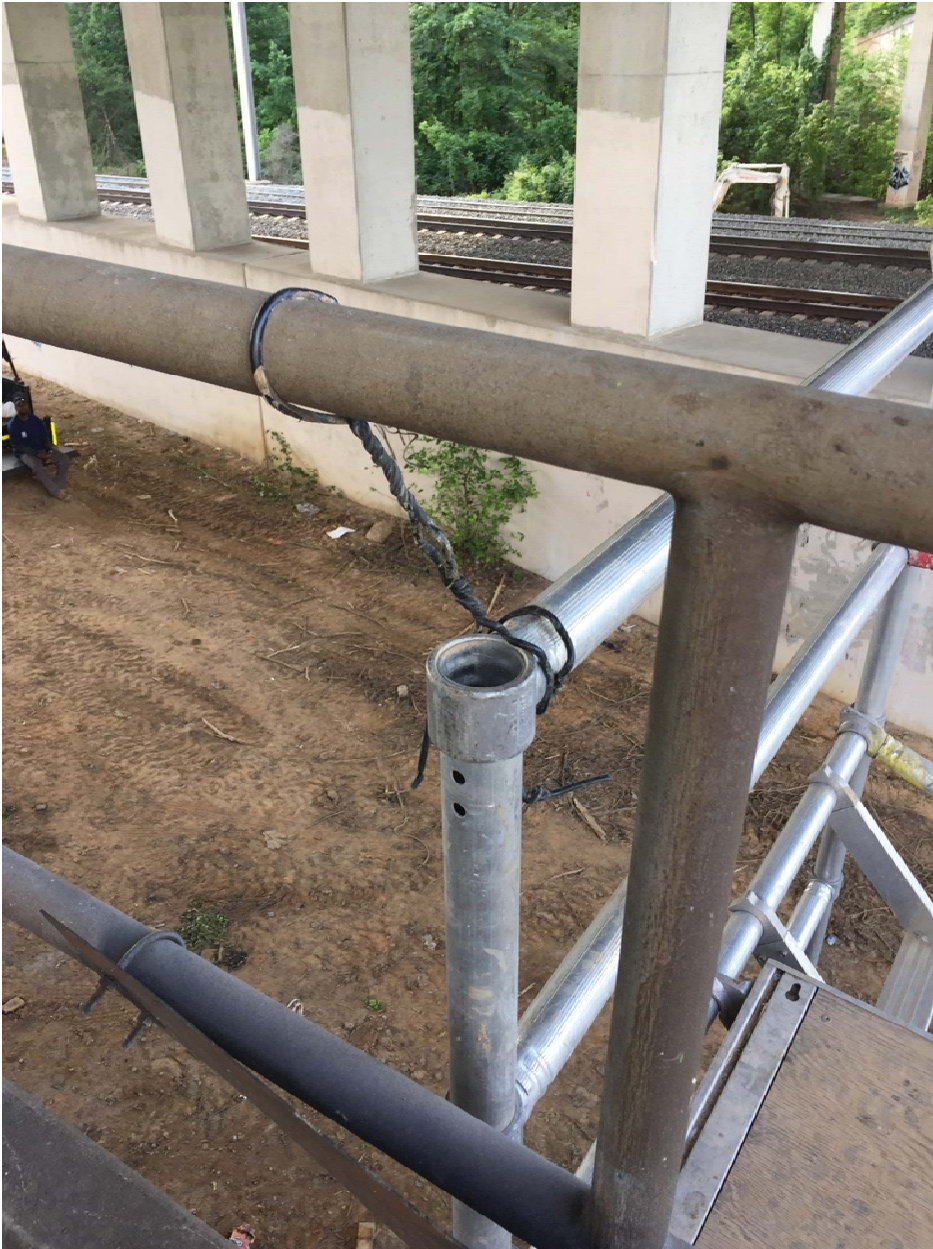
Photo 3: Scaffolding tied off with wire.
