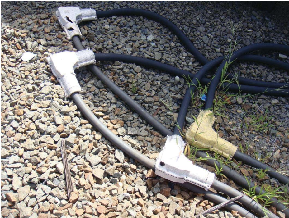
Figure 3 - 3rd Rail feeder cables lying on the ground. Connection boots are cracked.
