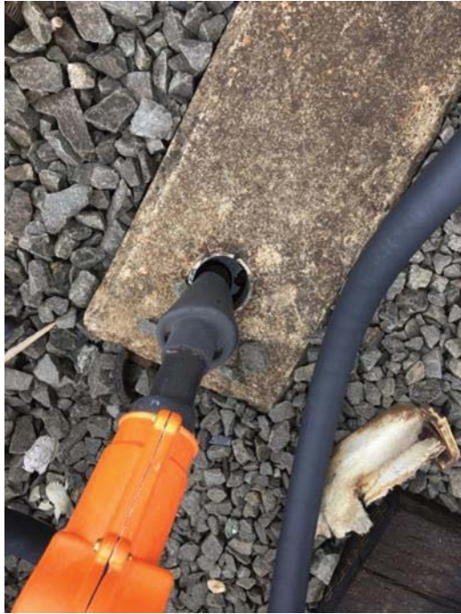
FIGURE 15 - YCR 2 – HEAT SHRINK ON CONDUIT STUB-UP COMPROMISED
