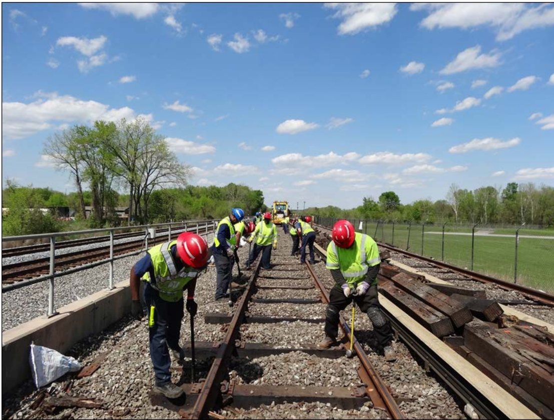
Surge 14 – Prince George’s Plaza to Greenbelt – WMATA Track and Structures gang connecting new ties to Track 2 rail in the vicinity of College Park-University of Maryland Station, April 18, 2017.
