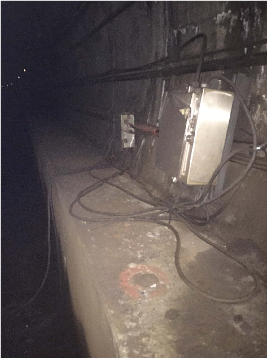
Photo 3. Exposed, non-secure wires on the tunnel walkway allowing a potential trip-and -fall hazard. This condition is compounded with the lack of tunnel lighting.
