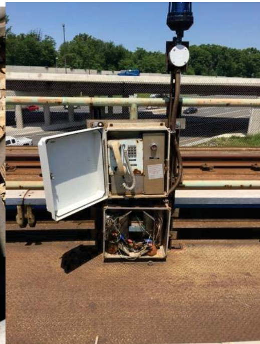
FIGURE 8 - TRK 1 CM 623+00 – ETS BOX ON AERIAL STRUCTURE MISSING FRONT PANEL AND NEED COMPLETE REPLACEMENT
