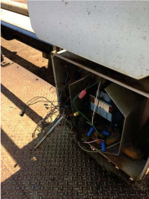
FIGURE 9 - TRK 2 CM 623+00 – ETS BOX ON AERIAL STRUCTURE MISSING FRONT PANEL AND NEED
