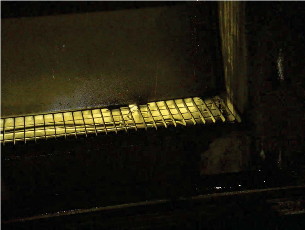
Figure 2 - Water leaking down above light fixture. Small white dots above the right end of the light fixture is water dripping
