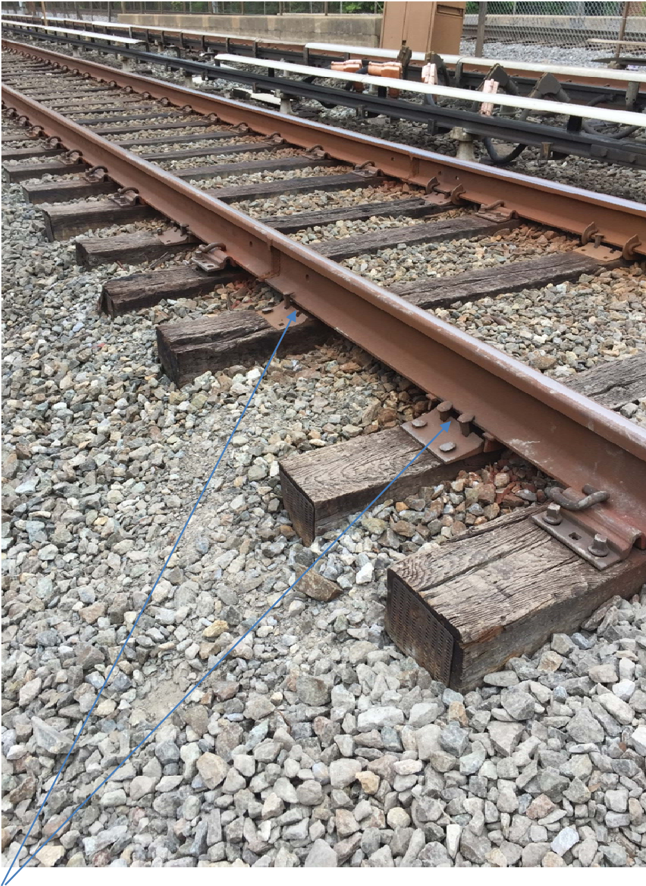
Photo 1. Overview of condition at B-07-08 signal, track two. Note rail was not seated properly into plates.
