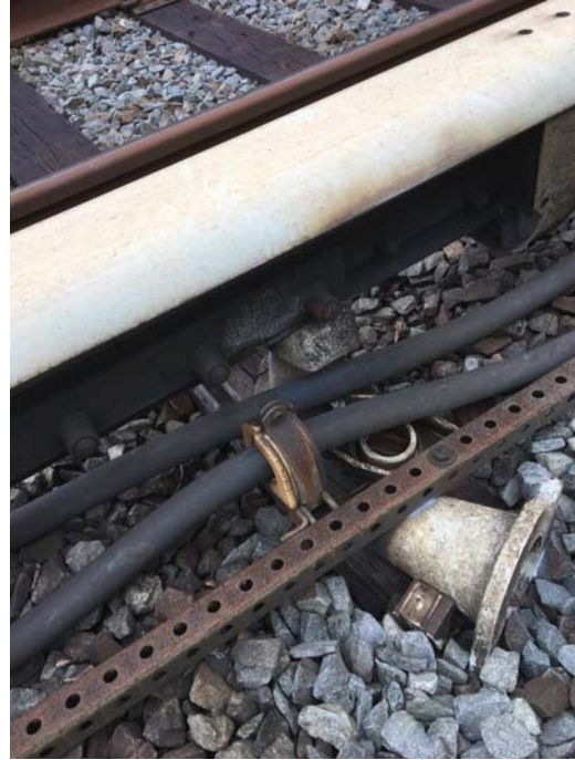
FIGURE 1 - TRK 2 CM 773+00 – CABLES STOOD OFF THE GROUND WITH THE OLD METAL KINDORF CHANNEL. THE CABLES HAVE SHIFTED TO WHERE A PORTION OF METAL KINDORF LATTICE STRUCTURE (OLD WAY OF STANDING CABLES OFF THE GROUND) IS ON THE GAGE SIDE OF THE THIRD RAIL
