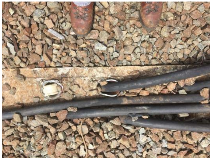
FIGURE 4 - TRK 2 CM 319+00 – NEGATIVE RETURN CABLE CONDUIT STUB-UP IN POWER DUCT BANK MISSING O-RING BUSHING.
