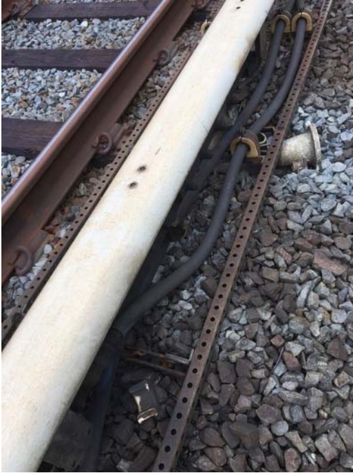
FIGURE 1 - TRK 2 CM 773+00 – CABLES STOOD OFF THE GROUND WITH THE OLD METAL KINDORF CHANNEL. THE CABLES HAVE SHIFTED TO WHERE A PORTION OF METAL KINDORF LATTICE STRUCTURE (OLD WAY OF STANDING CABLES OFF THE GROUND) IS ON THE GAGE SIDE OF THE THIRD RAIL
