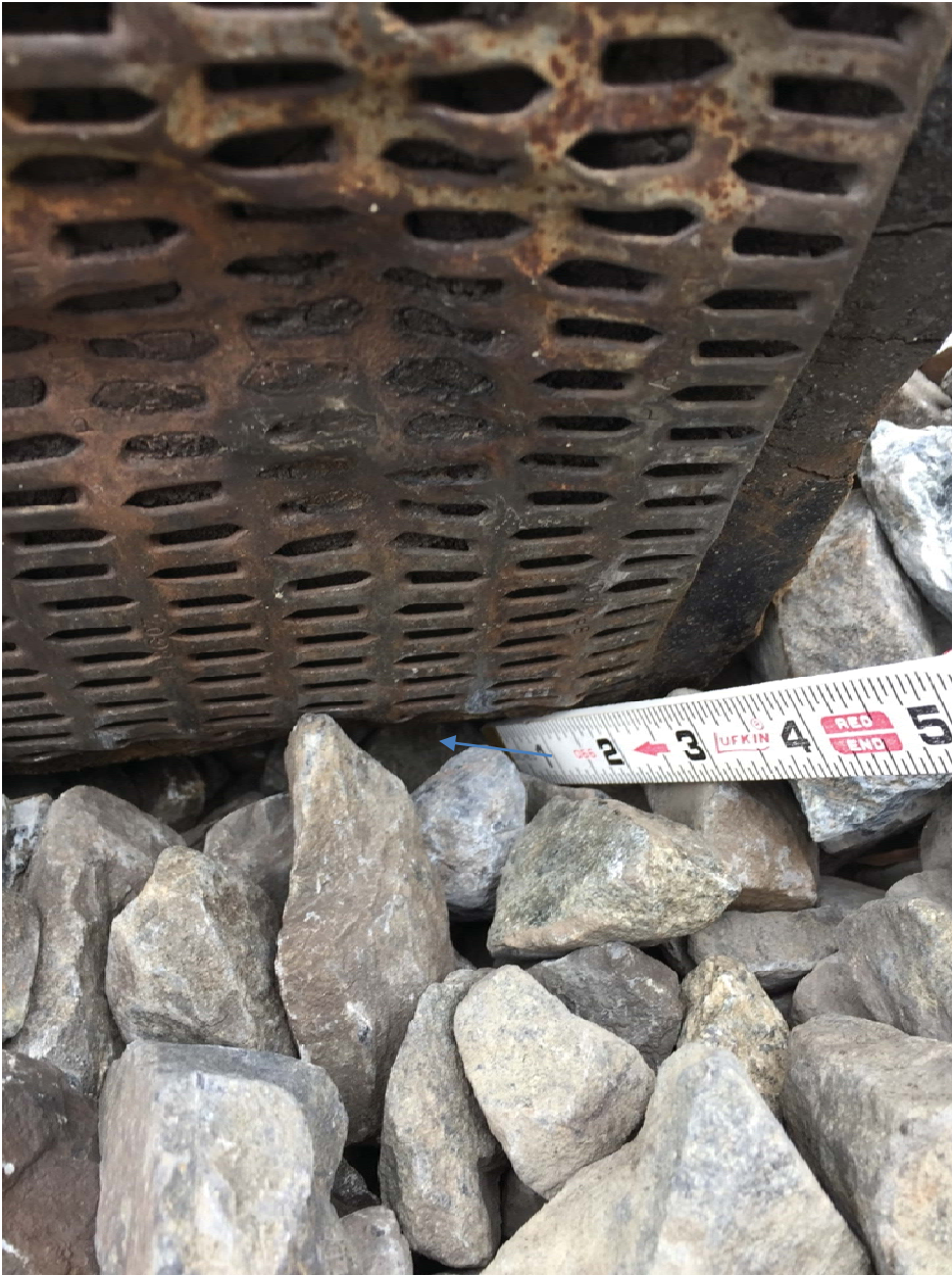
Photo 4. One inch void between bottom of tie and ballast
