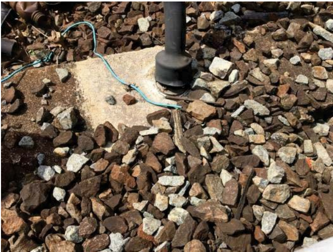
FIGURE 1 - TRK 1 CM 526+00 – CONDUIT STUB-UP HEAT SHRINK COMPROMISED
