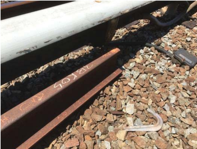
FIGURE 1 - TRK 2 CM 406+00 – RELAY RAIL TOO CLOSE TO 3 RD RAIL.
