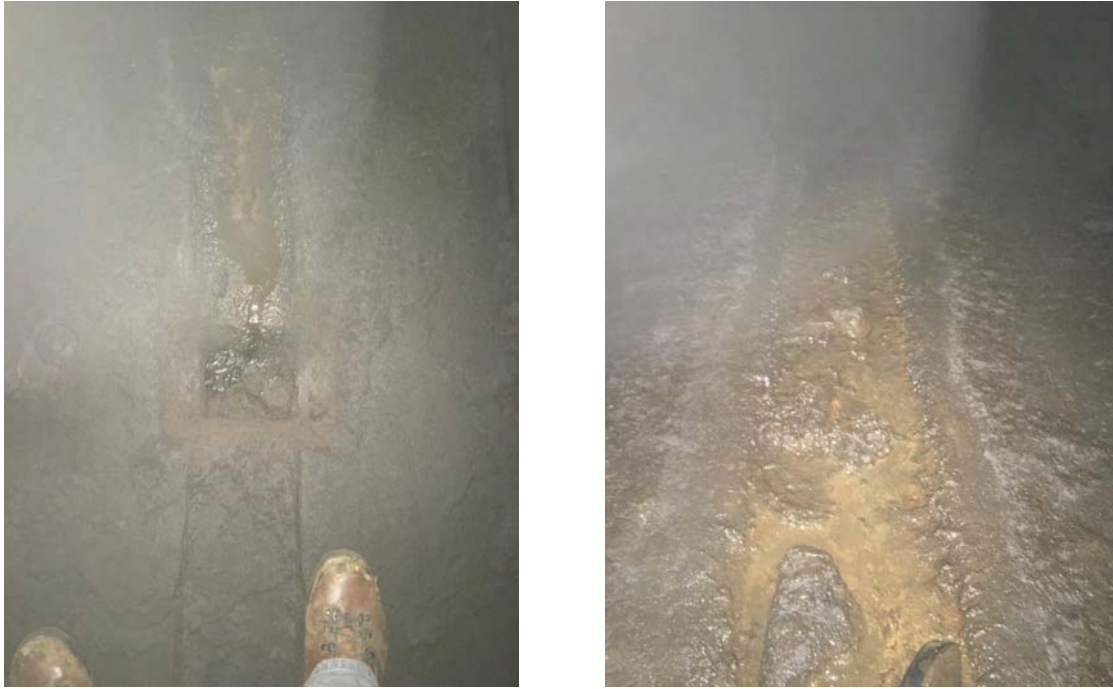
FIGURE 1 - TRK 2 CM 088+00 TO CM 089+00 – TRACK INVERT CLOGGED WITH MUD AND DEBRIS CAUSING STANDING WATER.
