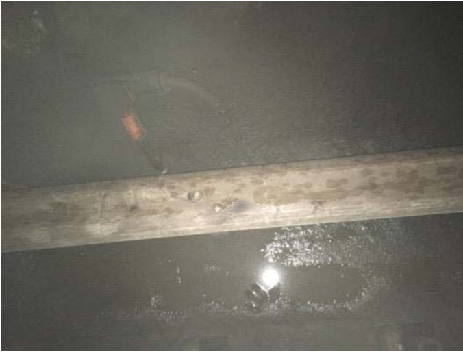
FIGURE 1 - TRK 2 CM 325+00 – MUD AND STANDING WATER SURROUNDING POWER CONDUIT STUB-UPS, ORANGE BOOTS, AND 3 RD RAIL POST INSULATORS
