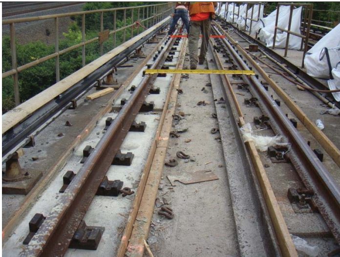
Figure 7 - New stud bolts are added and rail is lowered
