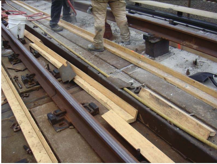
Figure 1 - New forms are constructed
