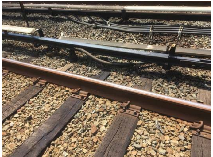
FIGURE 2 - TRK 2 CM 392+00 – EXPANSION CABLES ON FIELD SIDE OF 3 RD RAIL.
