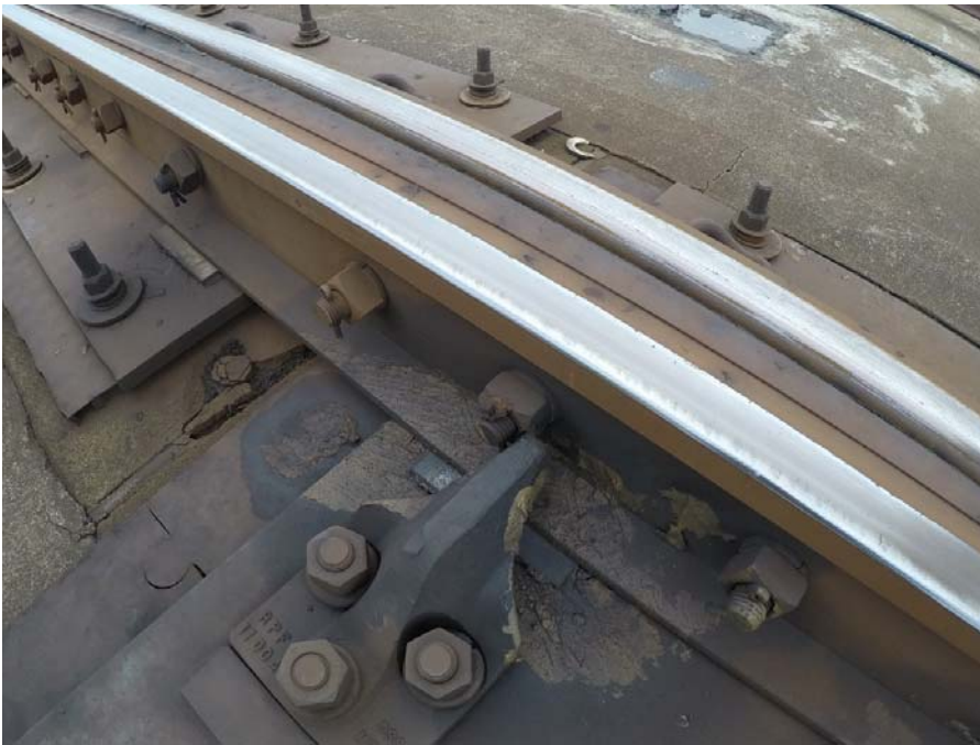
Photo 3: Switch point stop interfering with bolts preventing the switch from fully positioning when lined for turnout movement at switch nine at C1 360+70.
