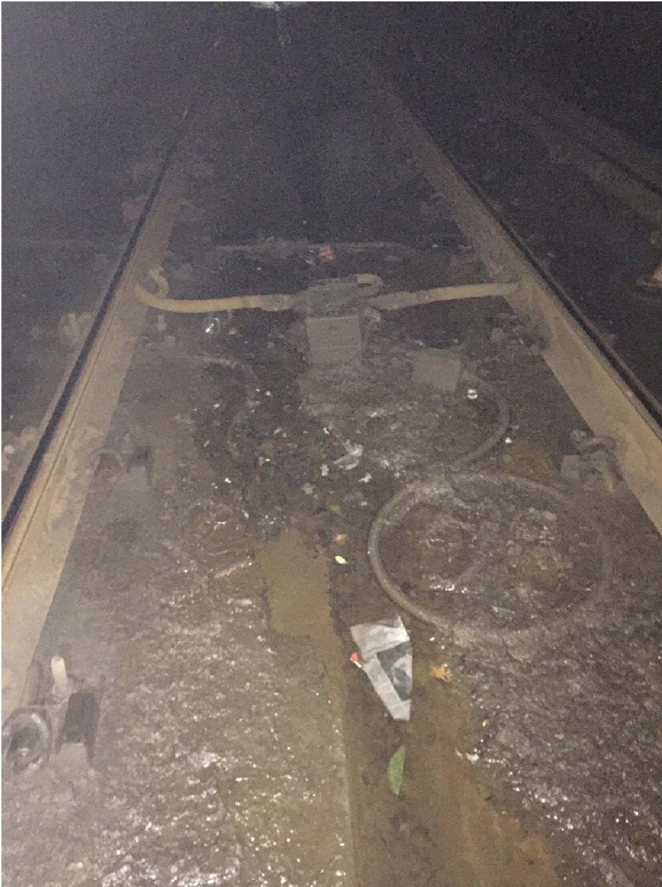
Photo 4. Mud and debris blocking center scupper, not allowing water to drain as designed.
