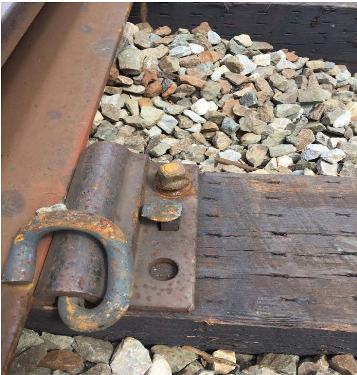
Photo 2: Gage spike not completely driven down.
