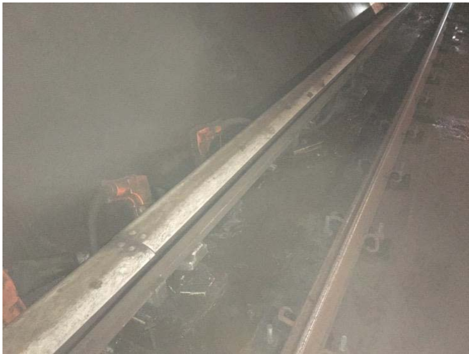
FIGURE 2 - TRK 2 CM 304+00 – MUD AND STANDING WATER SURROUNDING POWER CONDUIT STUB-UPS, ORANGE BOOTS, AND 3 RD RAIL POST INSULATORS
