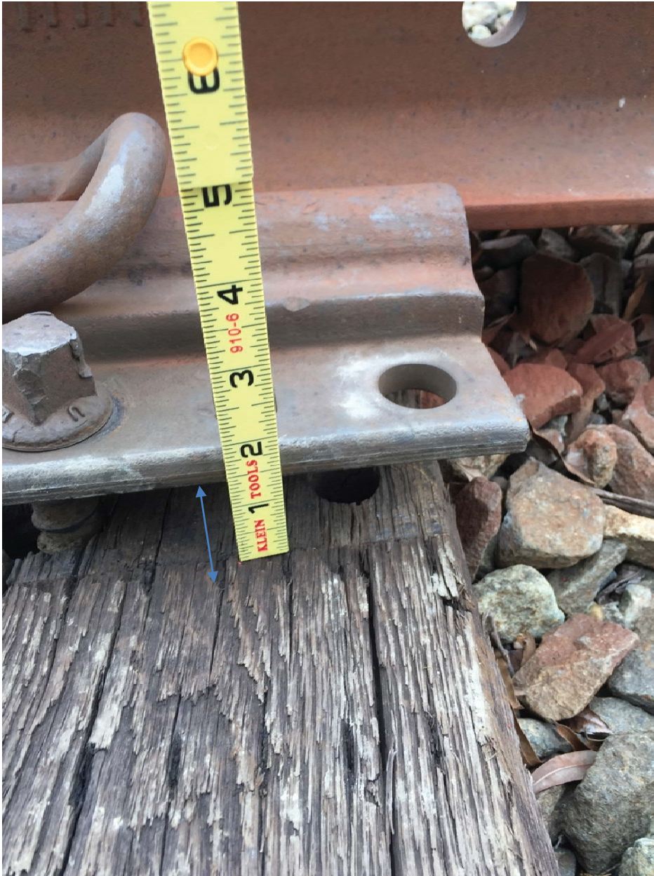
Photo 2. 1-5/8-inch spacing between tie and tie plate
