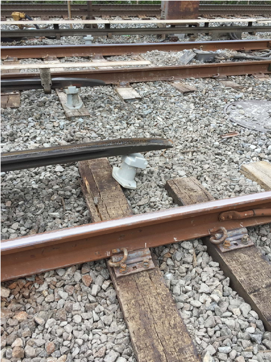
Photo 5. At the B-07-08 signal, unsecure third rail insulator and missing cover board
