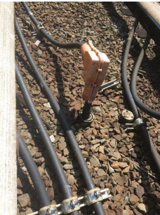
FIGURE 3 - TRK 2 CM 361+00 – POWER CONDUIT STUB-UP MISSING HEAT SHRINK.
