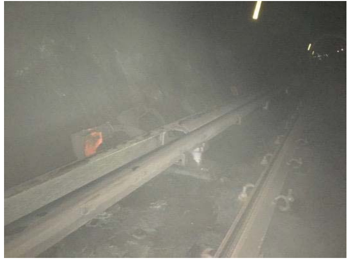
FIGURE 1 - TRK 2 CM 325+00 – MUD AND STANDING WATER SURROUNDING POWER CONDUIT STUB-UPS, ORANGE BOOTS, AND 3 RD RAIL POST INSULATORS
