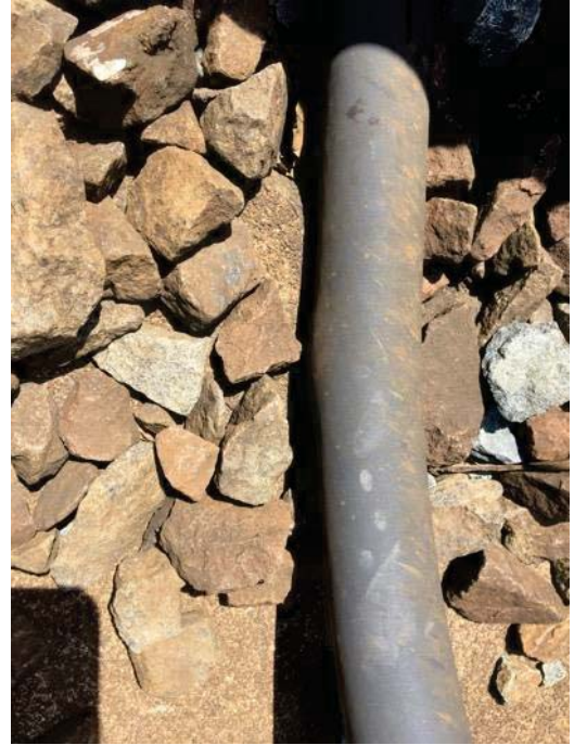
FIGURE 6 - TRK 1 CM 599+00 – CABLE NICKED/TORN
