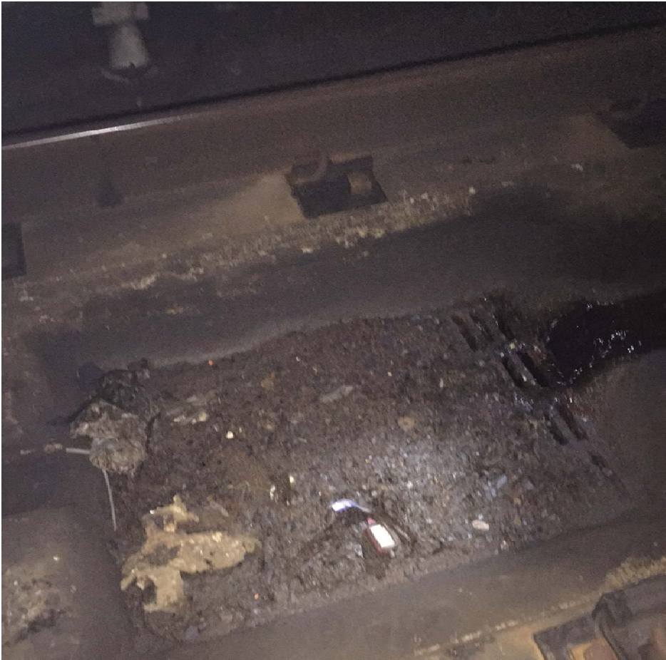
Photo 2. Blocked center drain.
