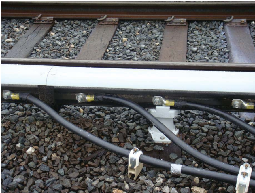
Figure 1 - Third rail jumper cables bolted to third rail.
