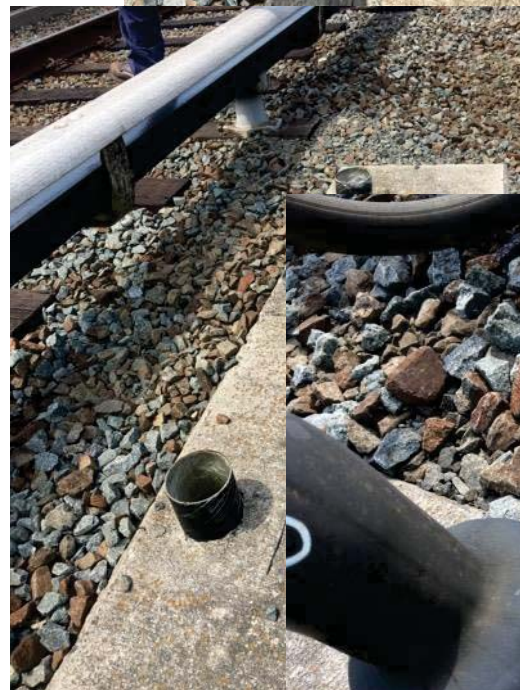
FIGURE 3 - TRK 1 CM 537+00 – NEEDED IN EMPTY/SPARE CON PREVENT WATER INFILTRATION
