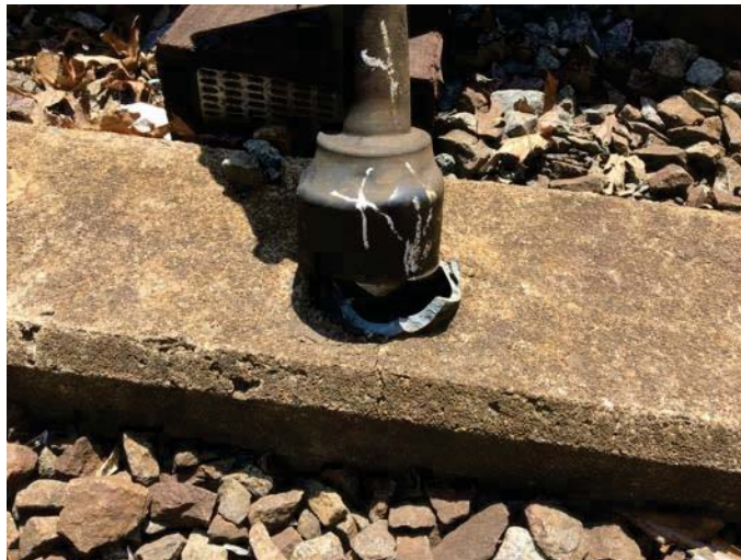
FIGURE 11 - TRK 1 CM 645+00 – CONDUIT STUB-UP BROKEN
