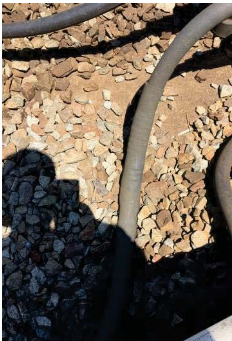
FIGURE 7 - TRK 1 CM 610+00 – CABLE PIGTAIL HAS TEMPORARY REPAIR, NEEDS REPLACEMENT
