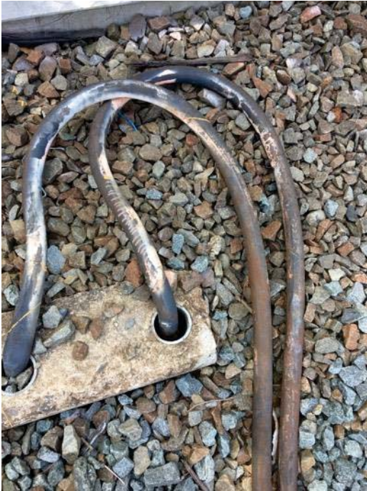
FIGURE 5 - TRK 1 CM 547+50 – O-Z/GEDNEY BUSHING NEEDED IN NEGATIVE RETURN CABLE CONDUIT STUB-UPS TO PREVENT WATER INFILTRATION (2 TOTAL)
