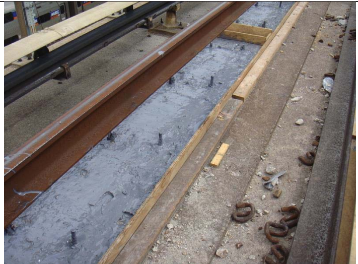
Figure 4 - New concrete cures around old stud bolts
