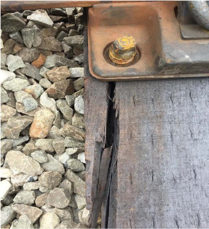
Photo 1: Newly installed crosstie split when lag bolt was installed.
