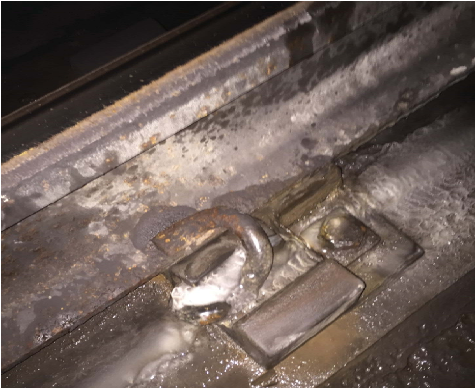
Photo 1. Tunnel leak permitting water to back-up to rail base and fastening system. Water condition beginning to cause corrosion to Pandrol clip.
