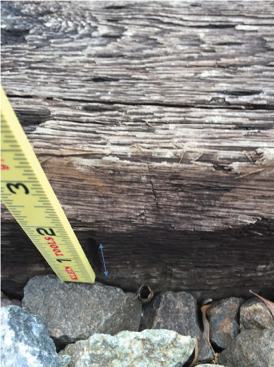
Photo 3. 1-3/8-inch dynamic (pumping mark) on tie
