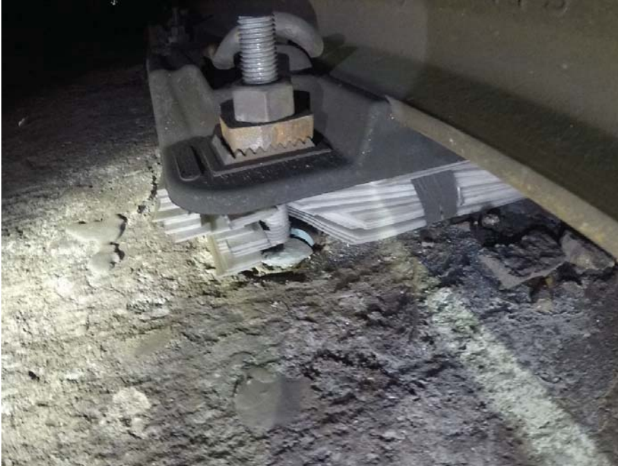
Photo 1: Shims used in lieu of grout pad at C1 301+20.
