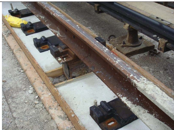
Figure 6 - New rail plates are placed under the rail
