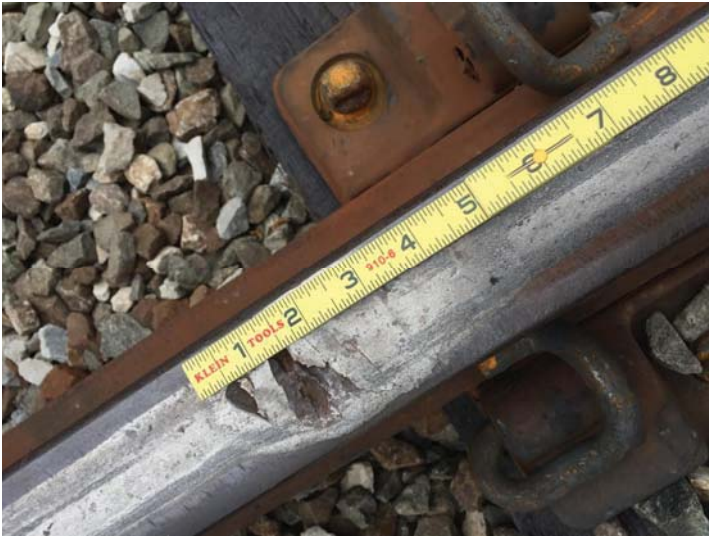
Photo 3: Four-inch running surface rail defect.
