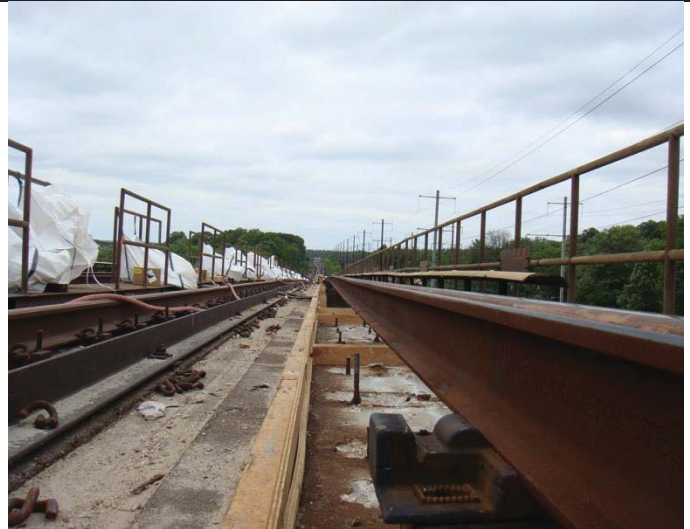
Figure 2 - Rail is raised up approximately 1-foot above the form
