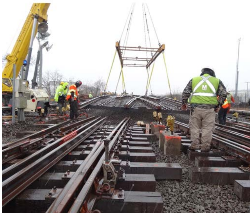
WMATA Force Account and Contractor G.W. Peoples installing new crossover at C98 interlocking on the "J" Line (vicinity Alexandria Yard). Photo taken March 10, 2017.
