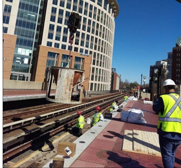
Surge 13 - Constructing Grout Pads at Eisenhower Avenue Station (top four photos)
