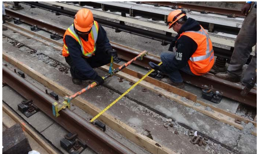
Surge 13 - From King Street Portal to Eisenhower Avenue Station - Checking the Gage
