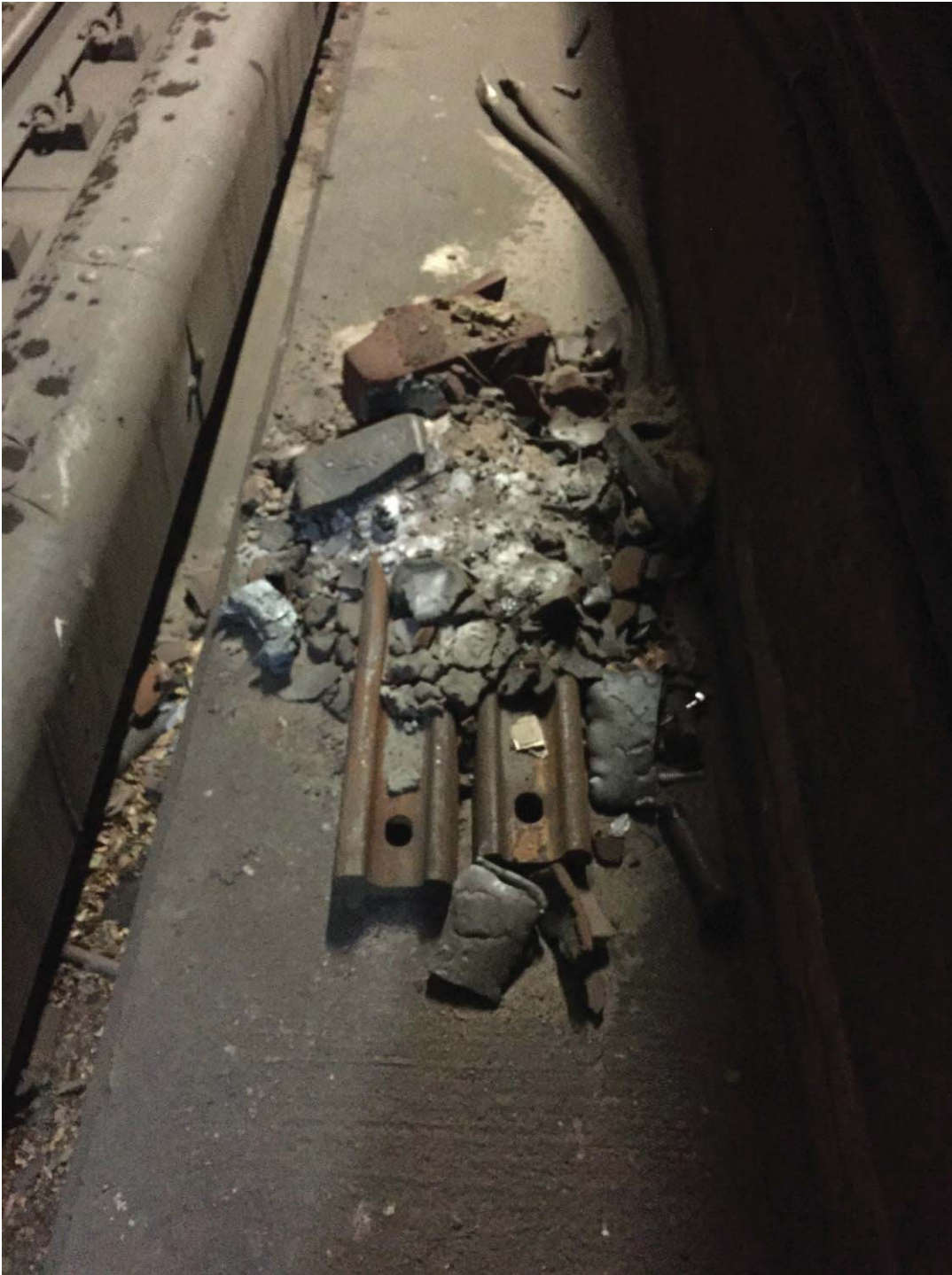
Other track material and debris blocking catwalk
