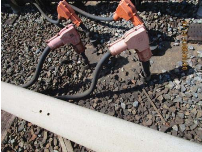
FIGURE 1 - TRK 2 CM 788+00 – HEAT SHRINK NEEDS REPLACEMENT ON CONDUIT STUB-UPS.
