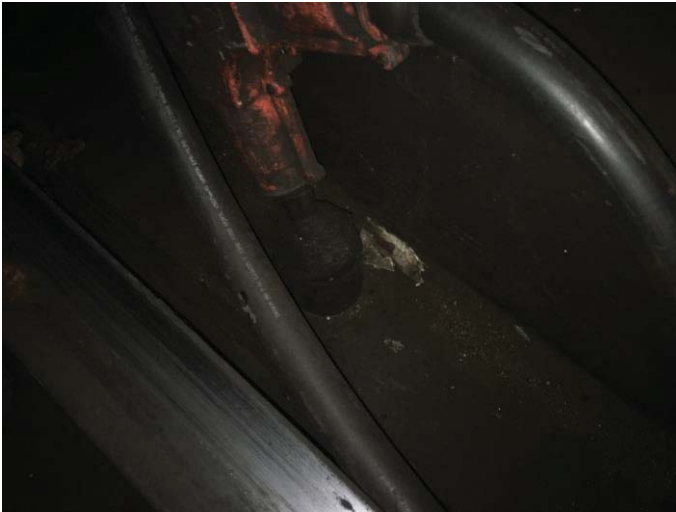
FIGURE 1 - TRK 1 CM 31+00 – CONDUIT STUB-UP COMPROMISED; HEAT SHRINK COMPROMISED ON CONDUIT STUB-UP
