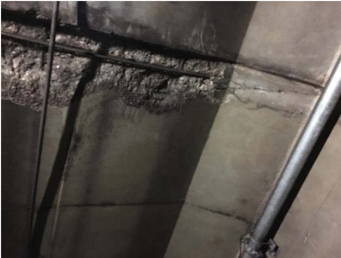
FIGURE 4 - TRK 1 CM 25+50 – CONCRETE DEBRIS FALLING FROM THE CEILING OF THE TUNNEL CLOSE TO THE 3 RD RAIL
