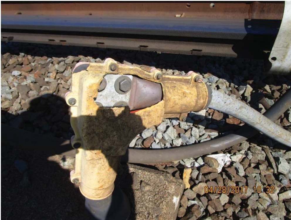
FIGURE 1 - TRK 2 CM 772+00 – BROKEN ORANGE BOOT
