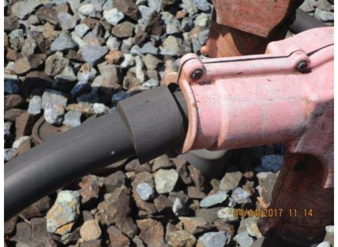
FIGURE 2 - TRK 2 CM 787+00 – NEOPRENE SLEEVE (SEALING COLLAR) WHERE CABLE PIGTAIL AND ORANGE BOOT MEET IS COMPROMISED.
