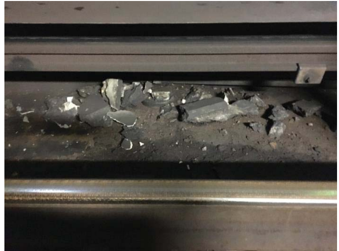
FIGURE 4 - TRK 1 CM 25+50 – CONCRETE DEBRIS FALLING FROM THE CEILING OF THE TUNNEL CLOSE TO THE 3 RD RAIL
