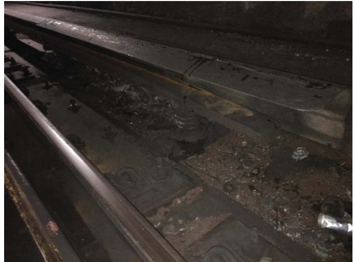
FIGURE 2 - TRK 1 CM 30+00 – CONDUIT STUB-UP COMPROMISED
