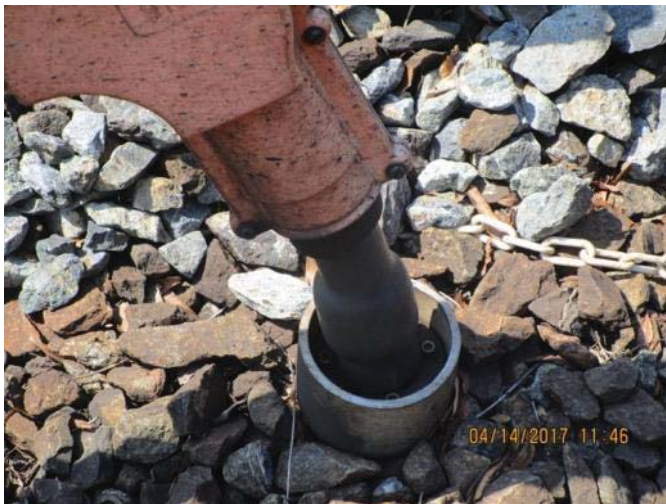
FIGURE 3 - TRK 2 CM 737+00 – HEAT SHRINK NEEDS REPLACEMENT ON CONDUIT STUB-UP.
