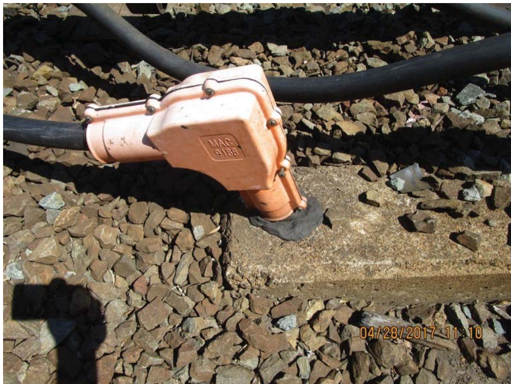
FIGURE 2 - TRK 2 CM 708+00 – CAPTIVE SCREWS LOOSE ON ORANGE BOOT
