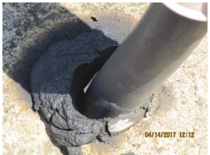
FIGURE 4 - TRK 2 CM 701+00 – HEAT SHRINK NEEDS REPLACEMENT ON CONDUIT STUB-UP.
