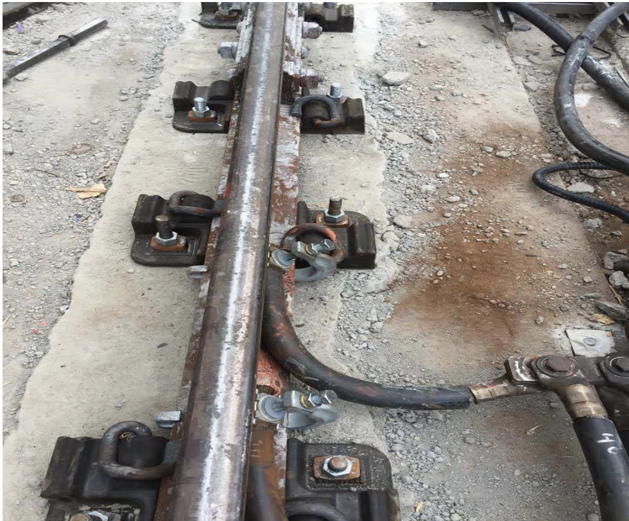
AT C14-06 SIGNAL, CM 592+90 DEFECTIVE GROUT PAD
