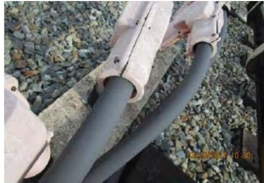
FIGURE 14 - YCR 59 – NEOPRENE SLEEVE COMPROMISED ON ORANGE BOOT
