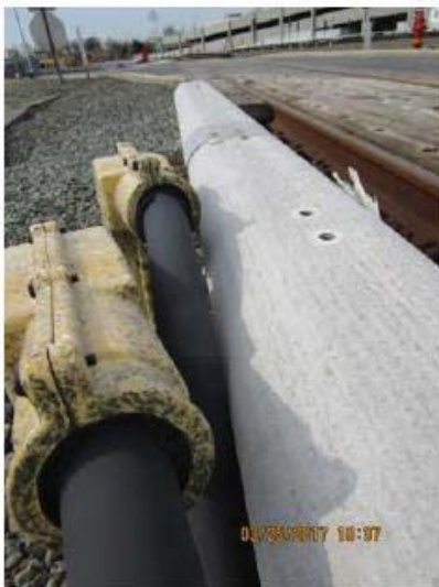
FIGURE 19 - YCR 138 – CABLES AND "BLOW DRYERS" TOO CLOSE TO 3 RD RAIL
