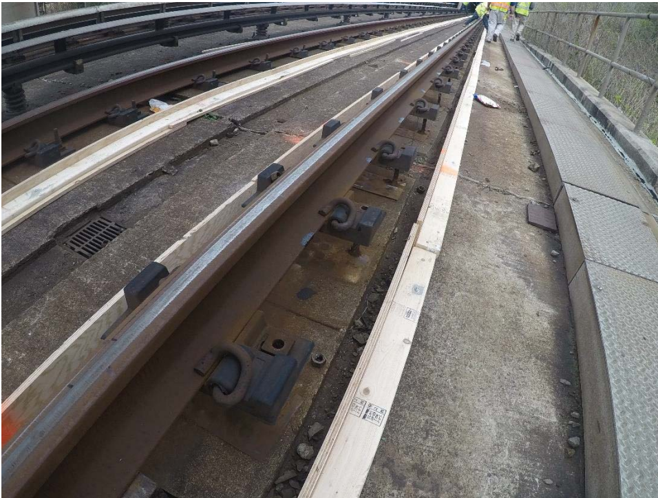
Newly installed forms for grout pads
