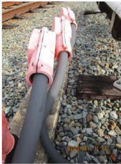
FIGURE 2 - YCR 62 – NEOPRENE SLEEVE COMPROMISED ON ORANGE BOOT
