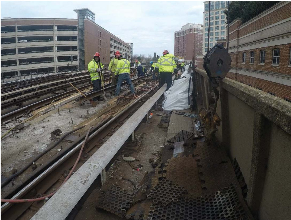
WMATA personnel jackhammering old grout pads.
