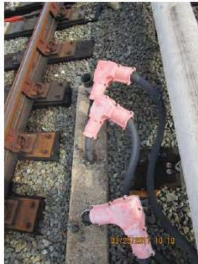
FIGURE 5 - YCR 77 – HEAT SHRINK COMPROMISED ON CONDUIT STUB-UP
