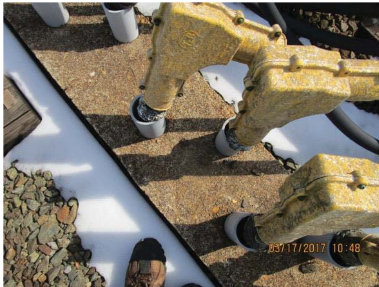
FIGURE 4 - YCR (YARD CONTACT RAIL) 25 – HEAT SHRINK COMPROMISED ON CONDUIT STUB-UPS
