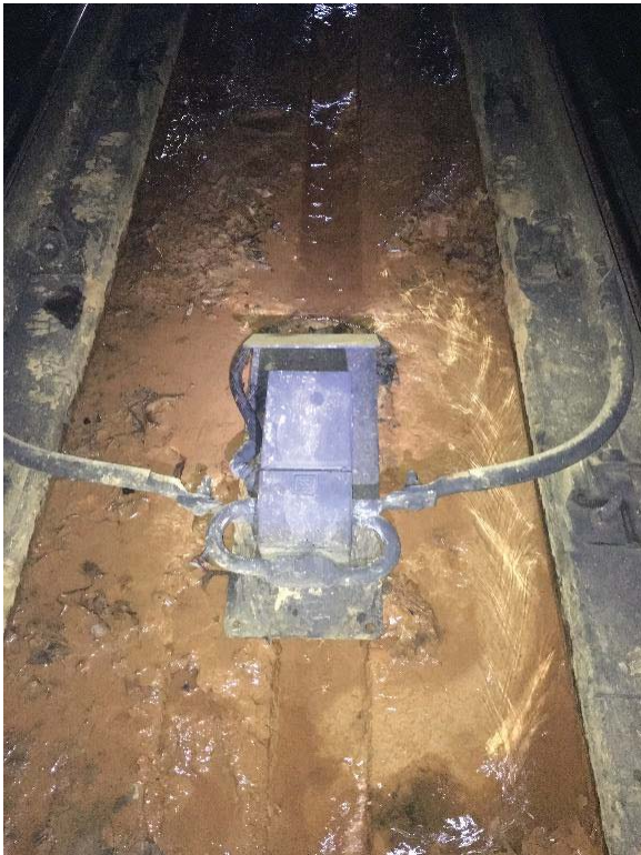
Clog under impedance bond at D2 230+50.
