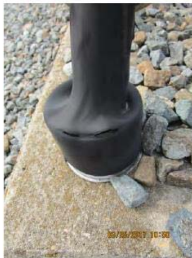
FIGURE 20 - YCR 35 – HEAT SHRINK COMPROMISED ON CONDUIT STUB-UP
