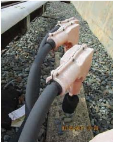
FIGURE 13 - YCR 123 – NEOPRENE SLEEVE COMPROMISED ON ORANGE BOOT
