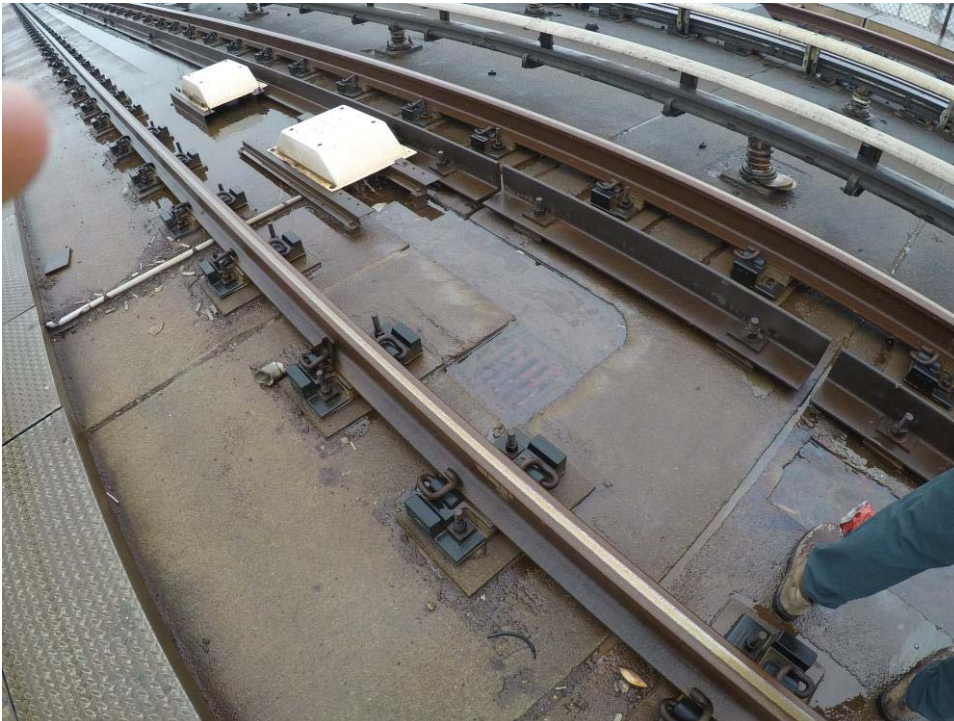
Clogged Drain at C1 603+00
