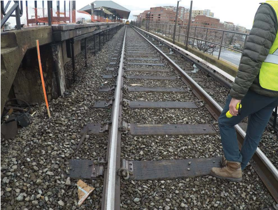
Recently Replaced Ties at Braddock Road Station
