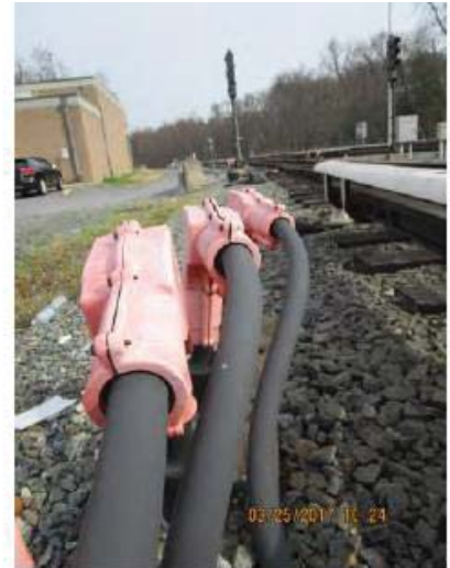
FIGURE 9 - YCR 75 – NEOPRENE SLEEVE COMPROMISED ON ORANGE BOOT
