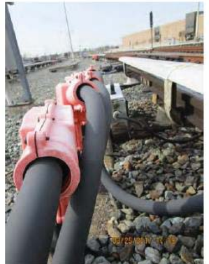
FIGURE 6 - YCR 76 – NEOPRENE SLEEVE COMPROMISED ON ORANGE BOOT
