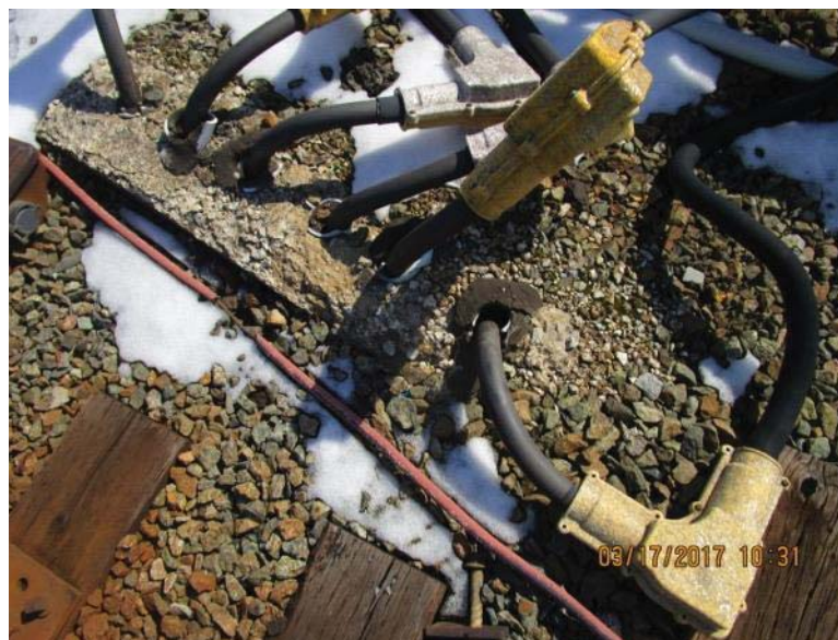
FIGURE 2 - YCR (YARD CONTACT RAIL) 81 – OZ GEDNEY BUSHINGS COMPROMISED
