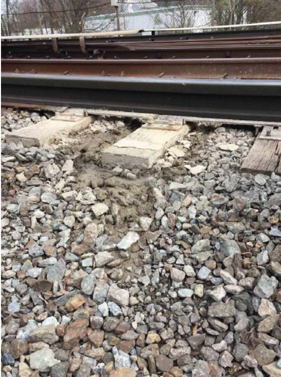
Foul ballast CM 351+10 static condition
