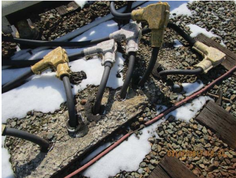
FIGURE 1 - YCR (YARD CONTACT RAIL) 81 – CONDUIT STUB-UPS BROKEN
