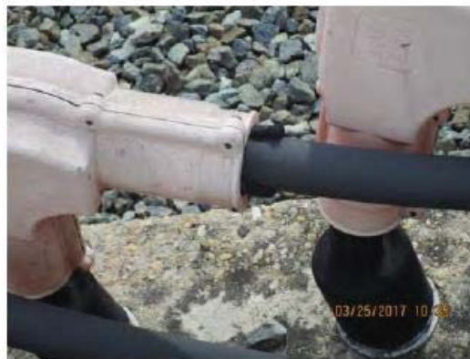
FIGURE 18 - YCR 144 – NEOPRENE SLEEVE COMPROMISED ON ORANGE BOOT
