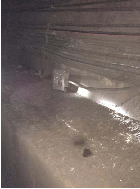
110-volt electrical box unsecured from the wall and on the walkway
