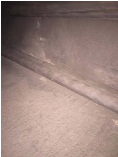
Conduit that became unattached from the wall and lying on the walkway
