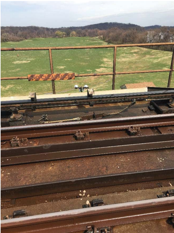
Broken third rail anchor at D2 266+20.
