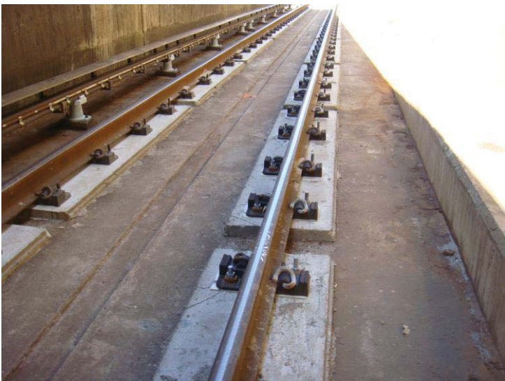
Figure 3 - New Grout Pad, Fasteners and Stud Bolts
