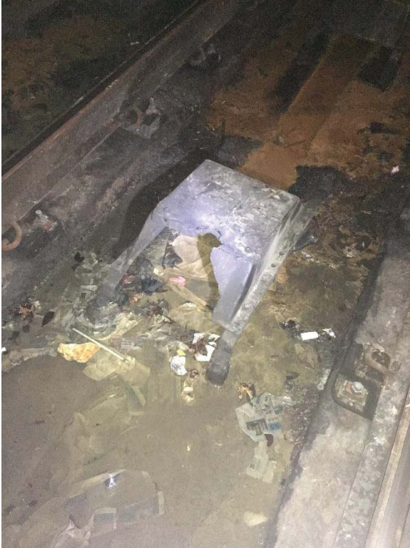
Clog under marker coil at D1 226+70
