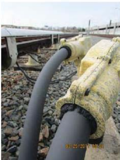
FIGURE 22 - YCR 37 – NEOPRENE SLEEVE COMPROMISED ON ORANGE BOOT
