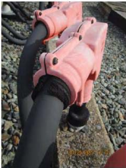
FIGURE 1 - YCR 63 – NEOPRENE SLEEVE COMPROMISED ON ORANGE BOOT
