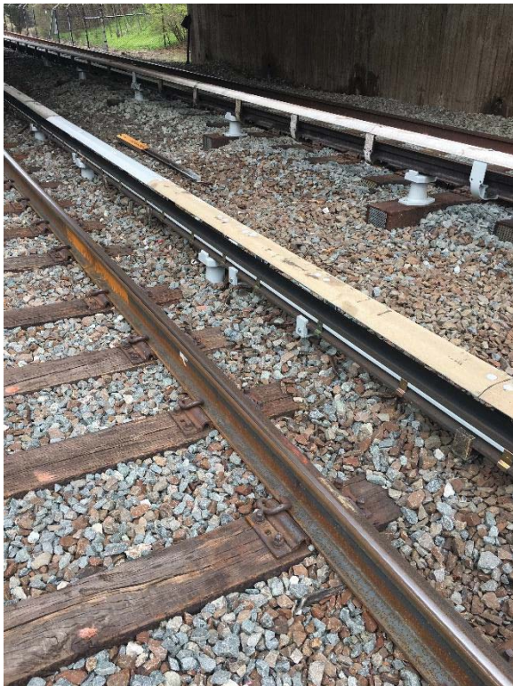
Ballast piled up against third rail between C2 195+40 and C2 207+00.
