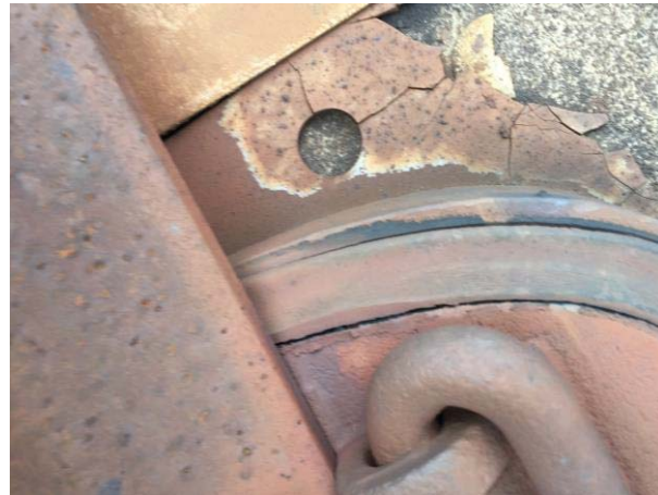
Broken and cracked egg fasteners. 360 degree cracks, not secure to the fastener and allowing rails to float, which threatens track geometry.
