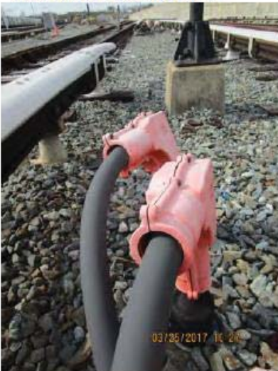
FIGURE 10 - YCR 61 – NEOPRENE SLEEVE COMPROMISED ON ORANGE BOOT
