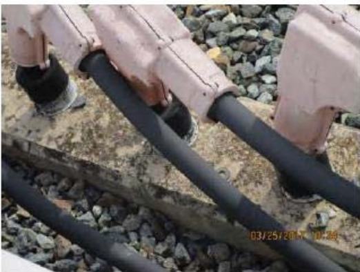
FIGURE 17 - YCR 60 – HEAT SHRINK COMPROMISED ON CONDUIT STUB-UP
