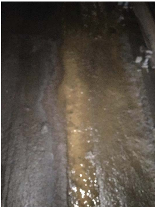
FIGURE 3 - TRK 1 CM 194+00 TO CM 196+00 - EXISTING DRAINAGE DITCHES IN TUNNEL ARE FULL OF MUD AND DEBRIS.
