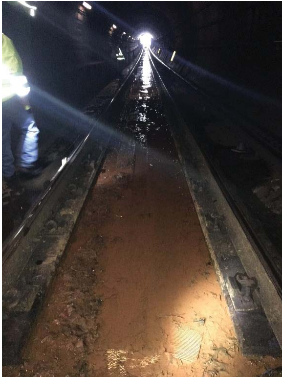
Poor drainage at D2 226+50.
