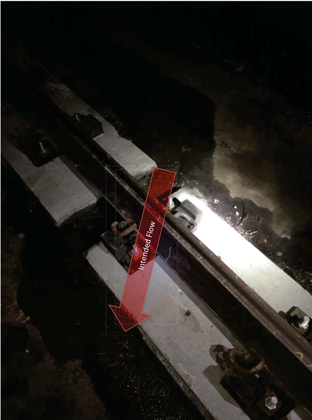
Grout pad obstructing drain at C2 162+60.
