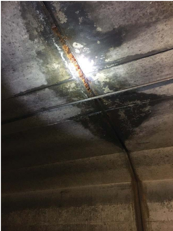
Leak in tunnel ceiling at C2 233+90.
