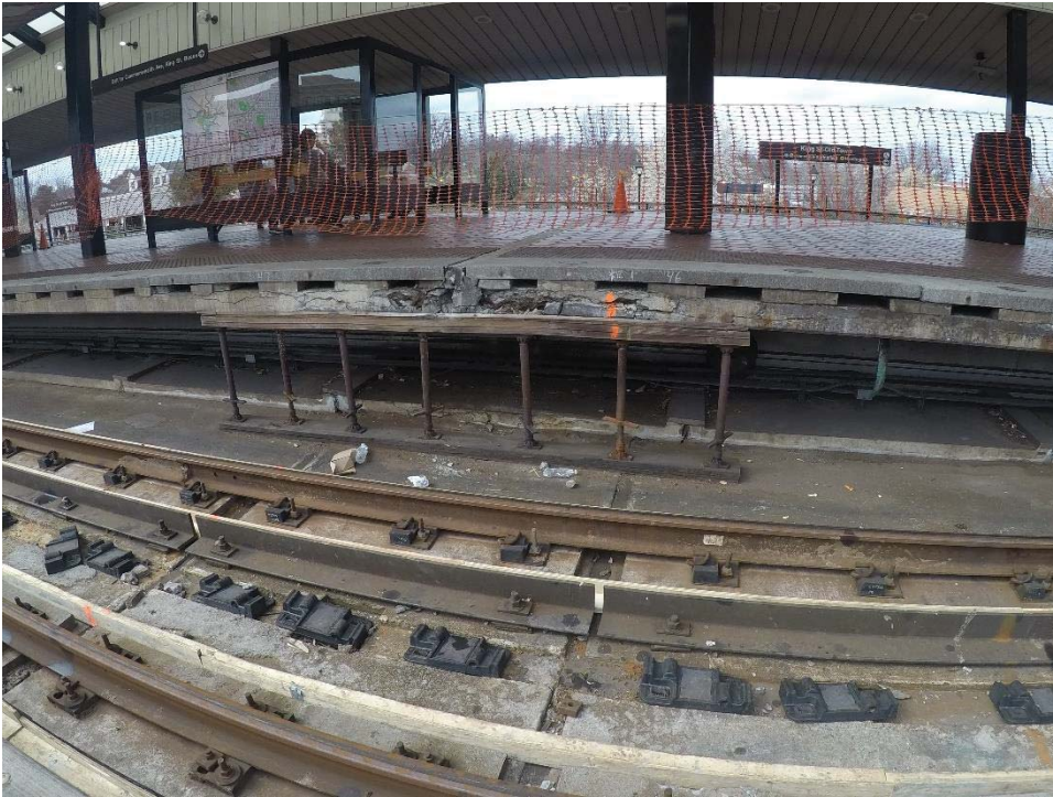
Granite platform edge supported by jacks
