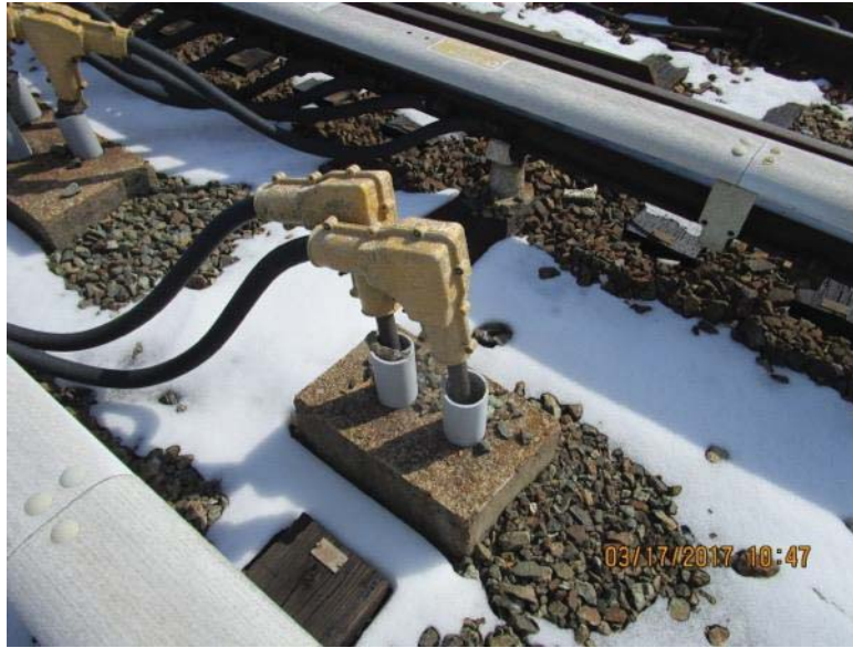
FIGURE 3 - YCR (YARD CONTACT RAIL) 16 – MISSING HEAT SHRINK ON CONDUIT STUB-UPS
