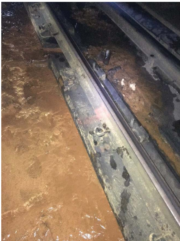
Defective fasteners at D2 231+50.
