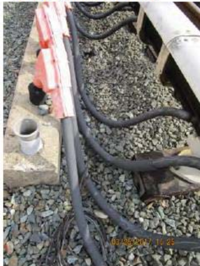
FIGURE 11 - YCR 61 – CABLE WITH TEMPORARY REPAIR
