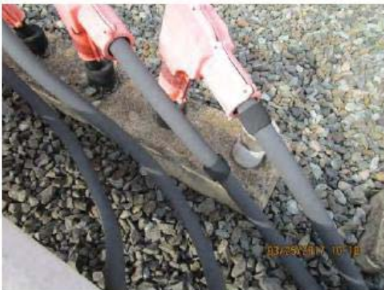
FIGURE 4 - YCR 77 – NEOPRENE SLEEVE COMPROMISED ON ORANGE BOOT
