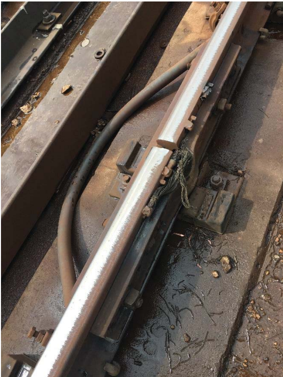
Joint bar mismatch at D1 270+10.
