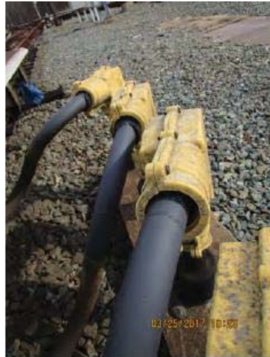
FIGURE 8 - YCR 82 – NEOPRENE SLEEVE COMPROMISED ON ORANGE BOOT
