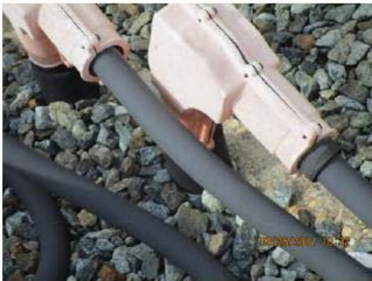
FIGURE 15 - YCR 58 – NEOPRENE SLEEVE COMPROMISED ON ORANGE BOOT
