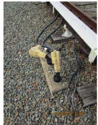
FIGURE 21 - YCR 35 –VERTICAL PORTION OF CABLE COMING THROUGH POWER DUCT BANK INTO "BLOW DRYER" TOO SHORT
