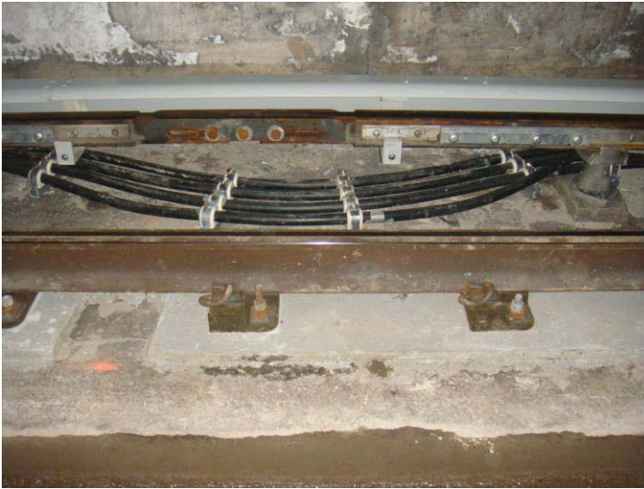
Figure 2 - New Grout Pads and Expansion Joint Cabling
