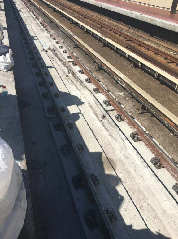
Completed Grout Pad Replacement at Eisenhower Avenue Station
