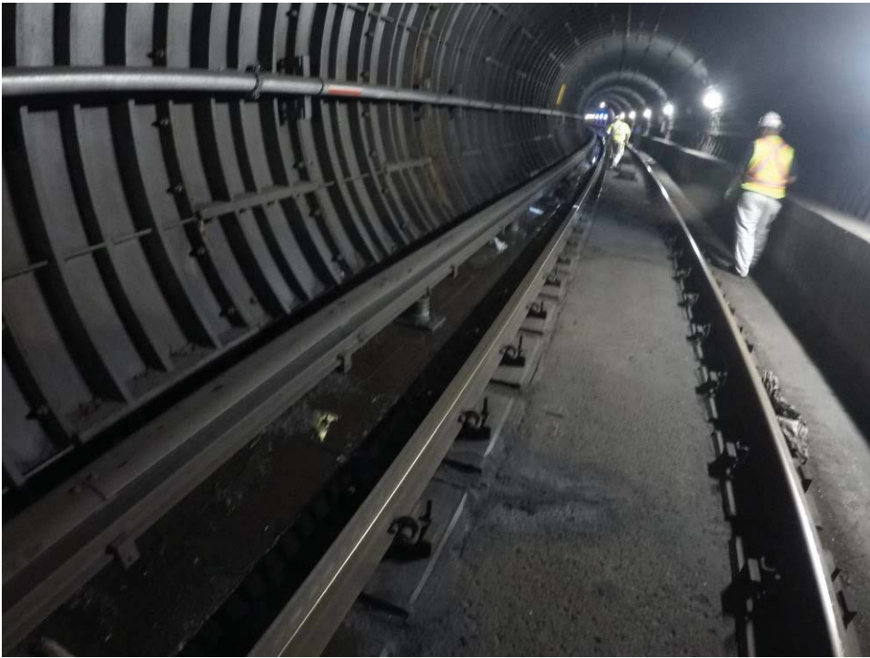
Standing Water underneath third rail at D1 74+30
