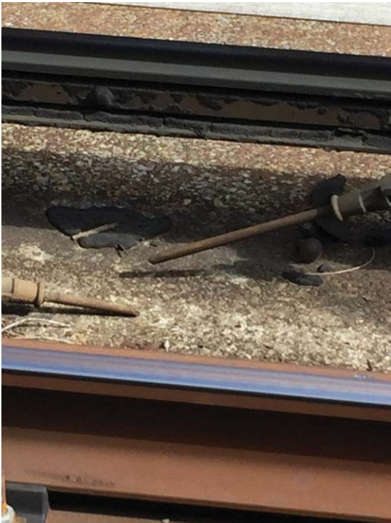
Broken third rail support cable.
