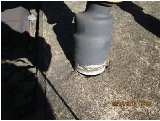
FIGURE 4 - TRK 2 CM 782+00 – CONDUIT STUB-UP BROKEN AND RUNNING RAIL JUMPER CABLES BADLY WORN
