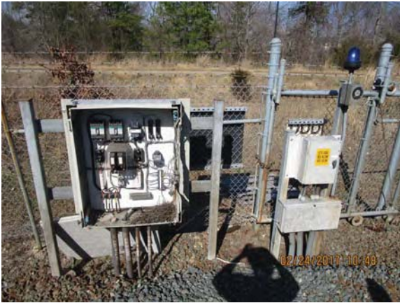
FIGURE 1 - TRK 2 CM 850+00 – TRACKSIDE HEATER PANEL DOOR MISSING
