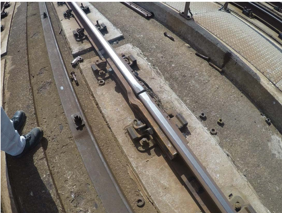
Joint Bar mismatch at A2 517+20
