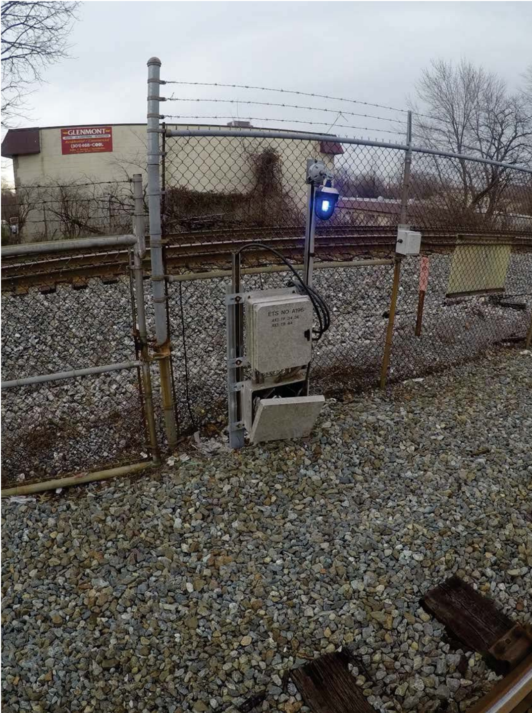
ETS box cover off at CM A2 708+00.
