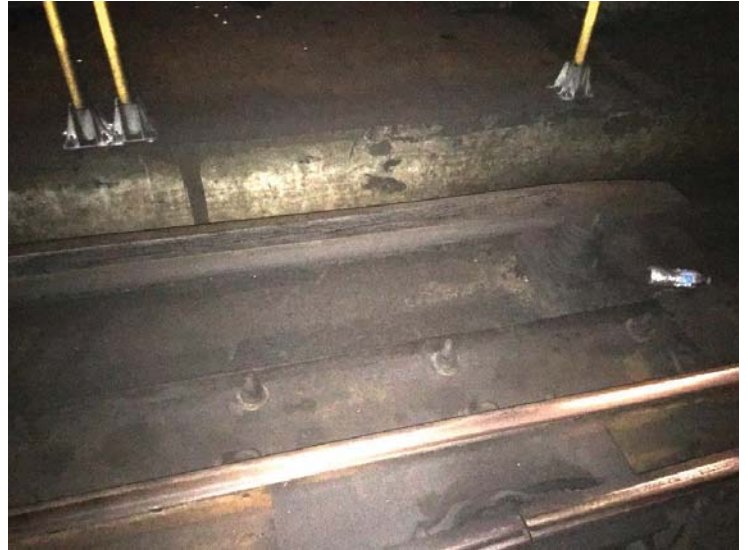
FIGURE 2 - TRK 1 CM 222+00 – 3 RD RAIL END APPROACH CORRODED
