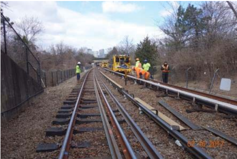
Tie crew replacing ties in surge area
