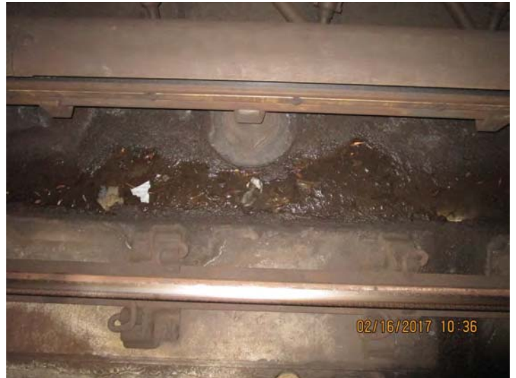
FIGURE 1 - TRK 1 CM 106+00 – WATER INTRUSION SURROUNDING CABLES
