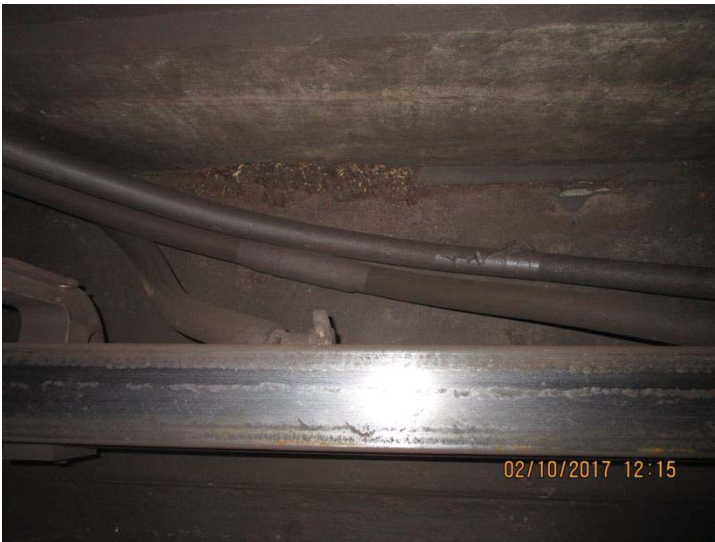
FIGURE 1 - TRK 1 CM 194+00 – WATER INTRUSION
