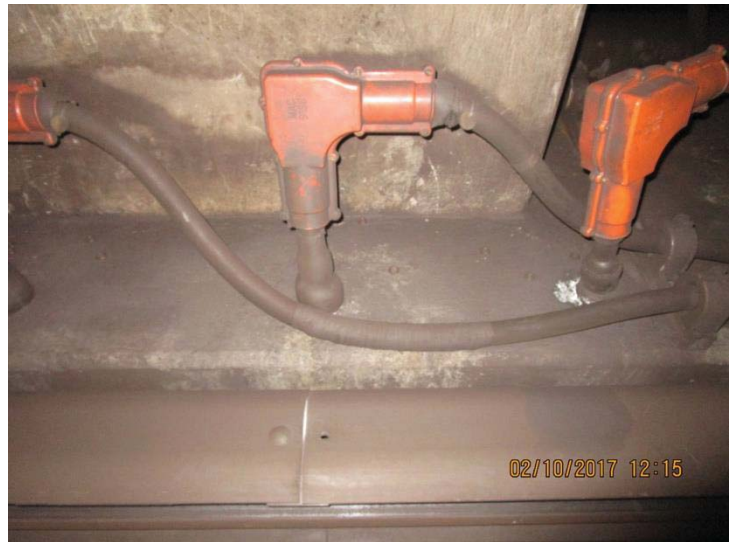
FIGURE 2 - TRK 1 CM 222+00 – 3 RD RAIL END APPROACH CORRODED
