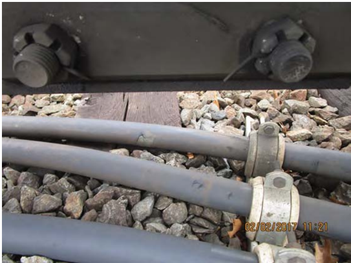
FIGURE 4 - TRK 2 CM 868+00 – DAMAGED CABLES AND TEMPORARY INSTALL OF STANDOFFS WITH ZIP TIES
