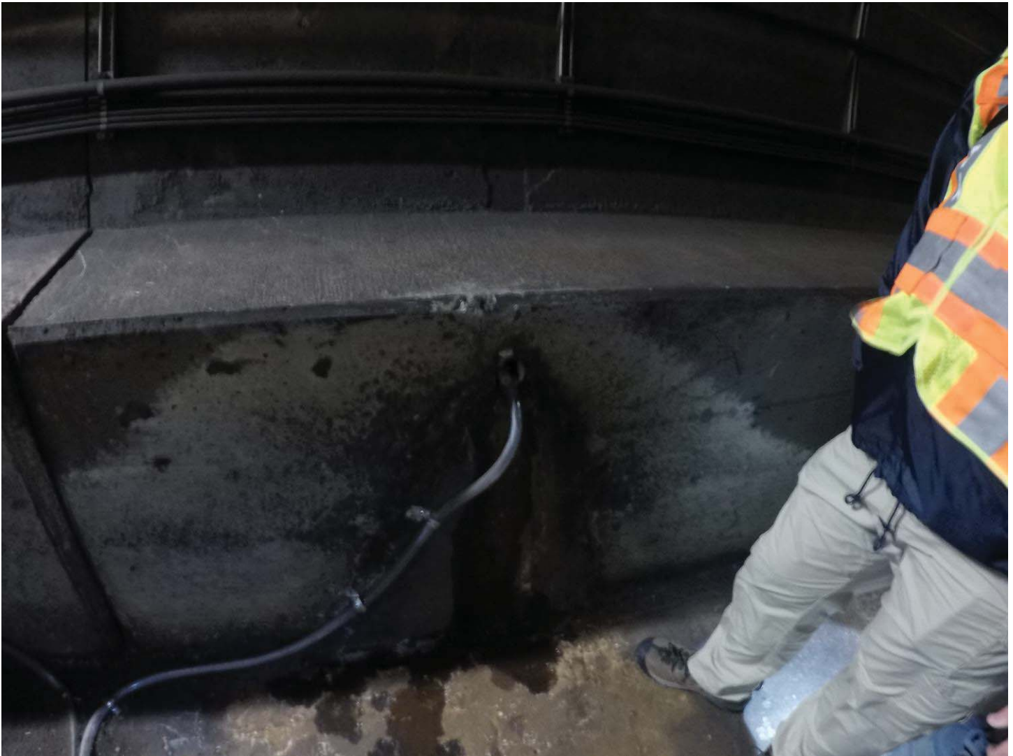
Hosing used to direct water flow
