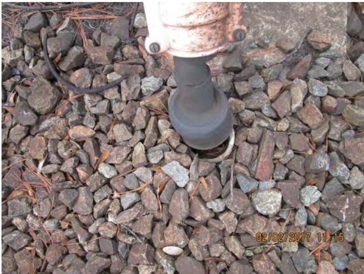
FIGURE 3 - TRK 2 CM 879+00 – HEAT SHRINK AND OZ GEDNEY BUSHING ON DUCT LINE TRANSITION COMPROMISED; TEMPORARY REPAIRED CABLE NEEDS REPLACEMENT
