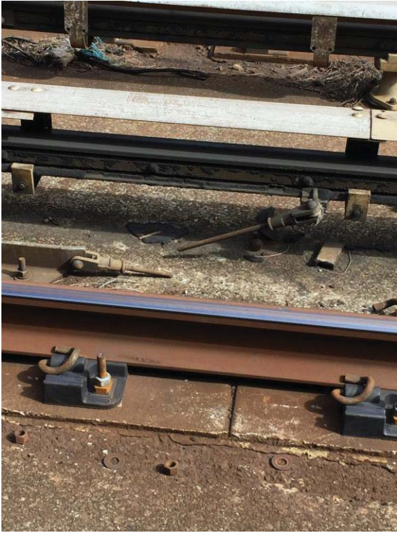
Broken third rail support cable.
