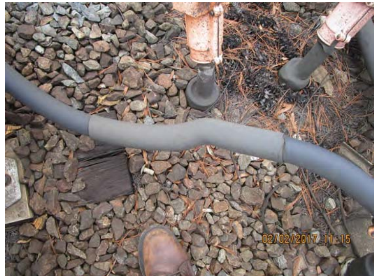
FIGURE 3 - TRK 2 CM 879+00 – HEAT SHRINK AND OZ GEDNEY BUSHING ON DUCT LINE TRANSITION COMPROMISED; TEMPORARY REPAIRED CABLE NEEDS REPLACEMENT
