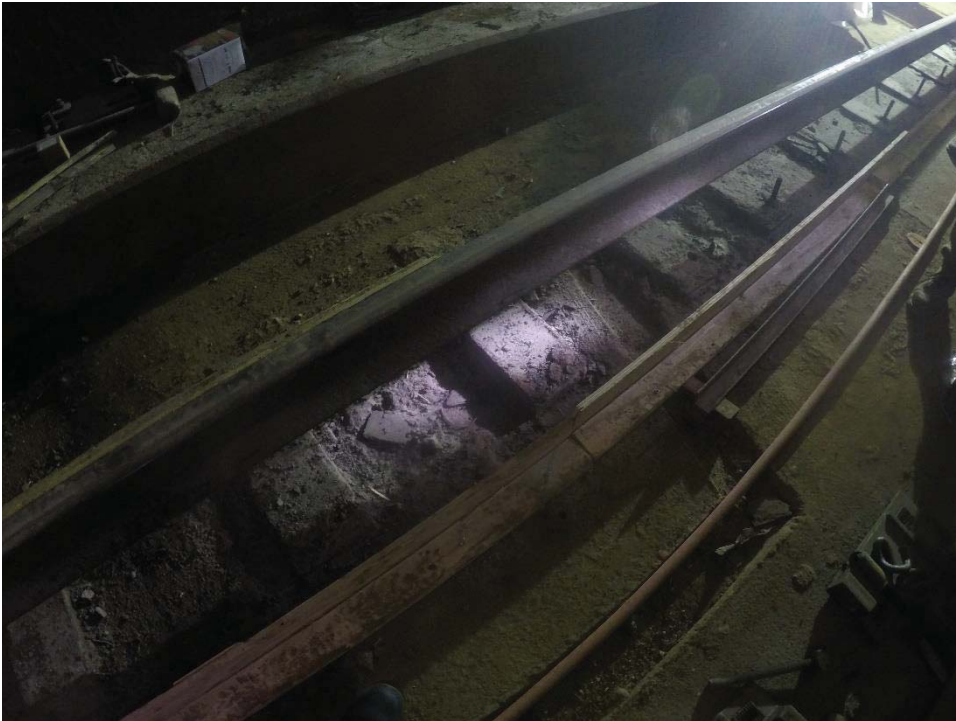
Old Grout Pads in the process of being jackhammered out
