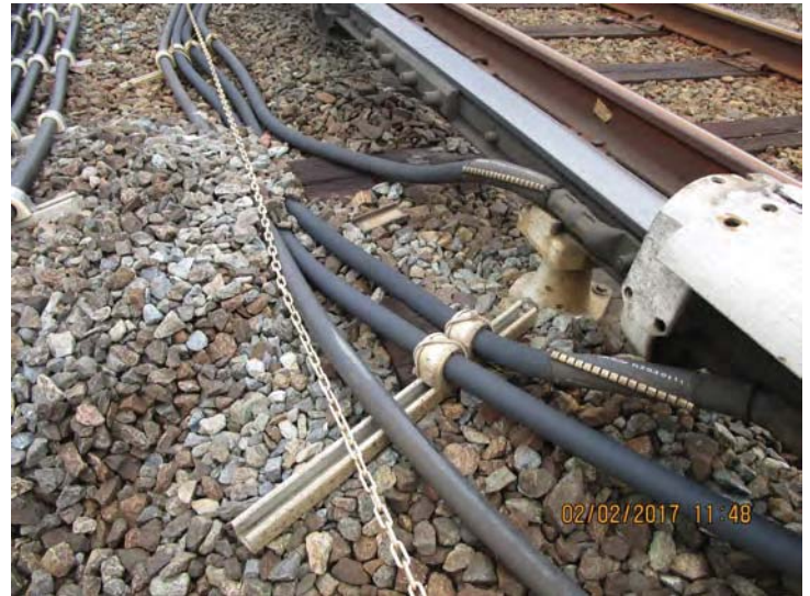
FIGURE 8 - TRK 2 CM 828+00 – TEMPORARY INSTALL OF ZIP TIES FOR FIBERGLASS CABLE STANDOFFS AND BURIED CABLES
