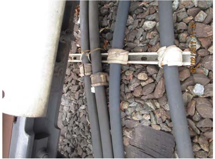
FIGURE 4 - TRK 2 CM 868+00 – DAMAGED CABLES AND TEMPORARY INSTALL OF STANDOFFS WITH ZIP TIES
