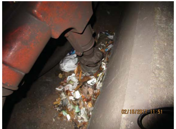
FIGURE 3 - TRK 1 CM 023+00 – HEAT SHRINK NEEDS REPLACEMENT ON STUB-UP AND TRASH SURROUNDING CABLE
