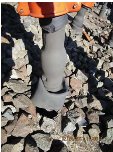
FIGURE 3 - TRK 2 CM 826+00 – CONDUIT STUB-UP AND HEAT SHRINK COMPROMISED
