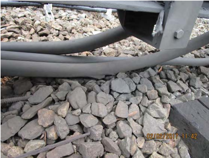
FIGURE 7 - TRK 2 CM 838+00 – DAMAGED CABLES
