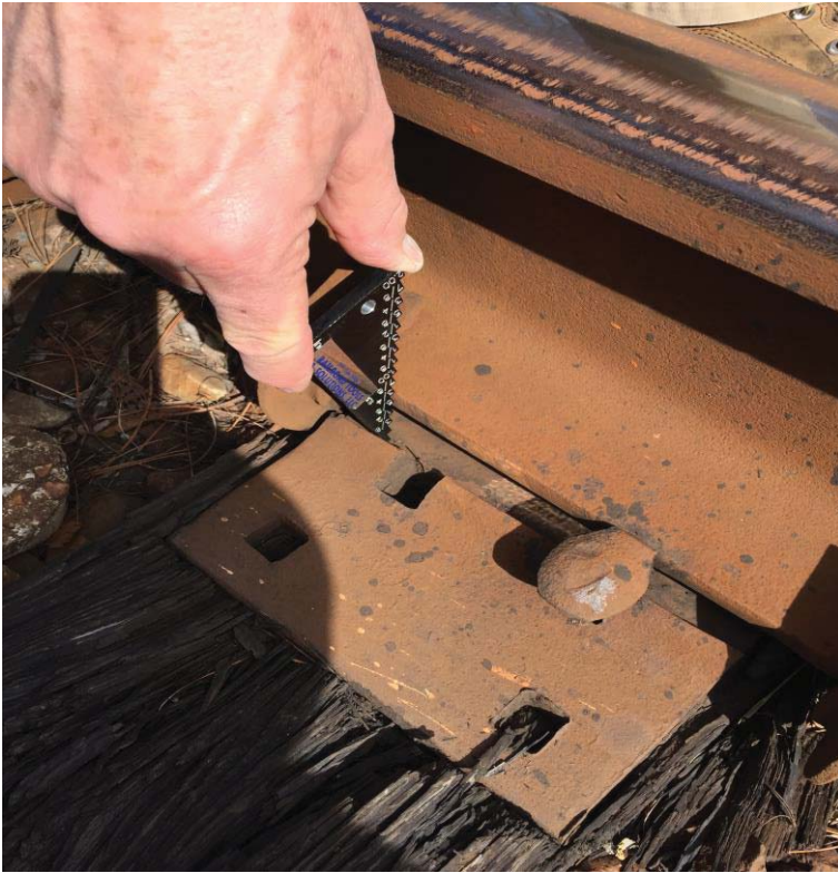
Rail not properly seated in rail plates permitting 1-inch dynamic vertical deflection under load.
