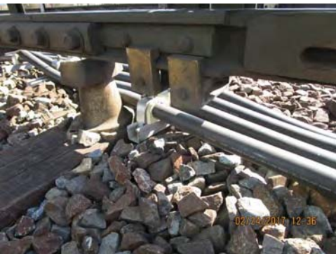
FIGURE 6 - TRK 2 CM 705+00 – 3 RD RAIL INSULATOR NOT SUPPORTING 3 RD RAIL
