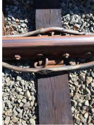
FIGURE 4 - TRK 2 CM 782+00 – CONDUIT STUB-UP BROKEN AND RUNNING RAIL JUMPER CABLES BADLY WORN
