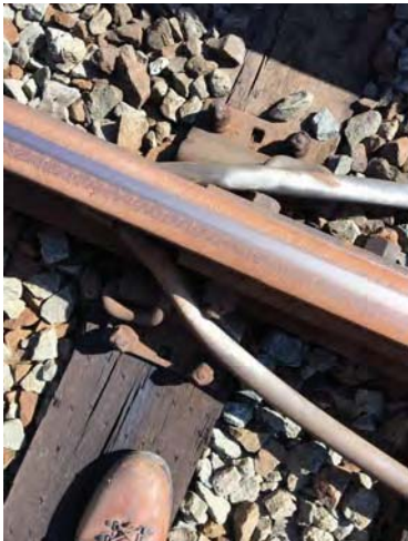
FIGURE 2 - TRK 2 CM 827+00 – RUNNING RAIL JUMPER CABLES WORN
