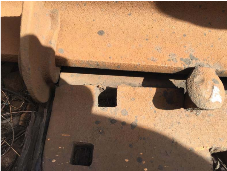
3/4 -inch gap between base of rail and rail plate
