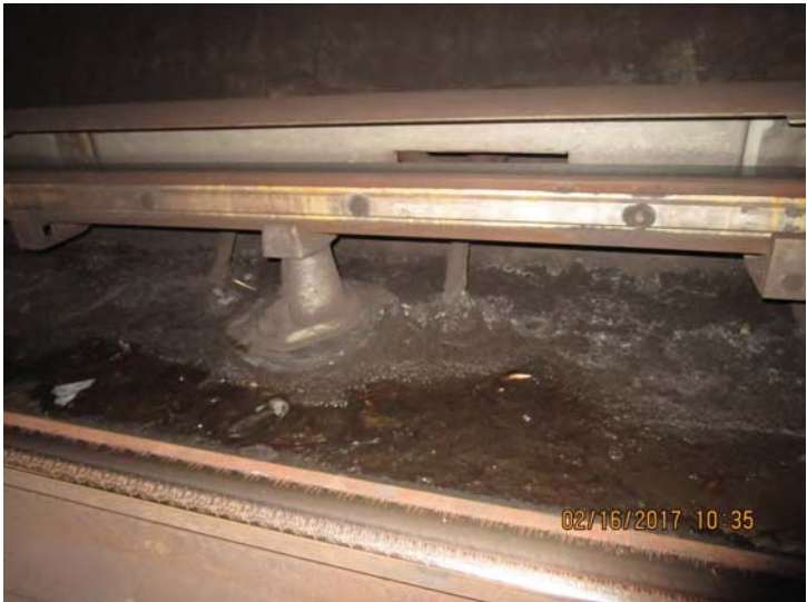
FIGURE 1 - TRK 1 CM 106+00 – WATER INTRUSION SURROUNDING CABLES
