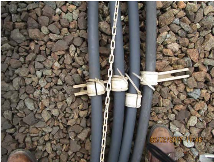
FIGURE 8 - TRK 2 CM 828+00 – TEMPORARY INSTALL OF ZIP TIES FOR FIBERGLASS CABLE STANDOFFS AND BURIED CABLES
