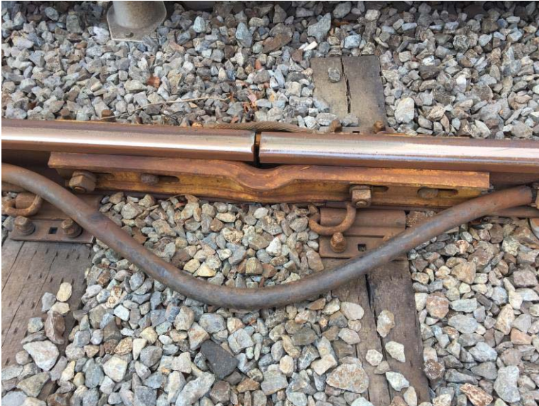
Welding strap bars being used as angle bars
