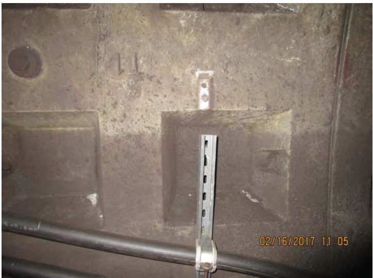
FIGURE 2 - TRK 1 CM 063+00 – KINDORF CHANNEL NEEDS REATTACHMENT TO TUNNEL WALL
