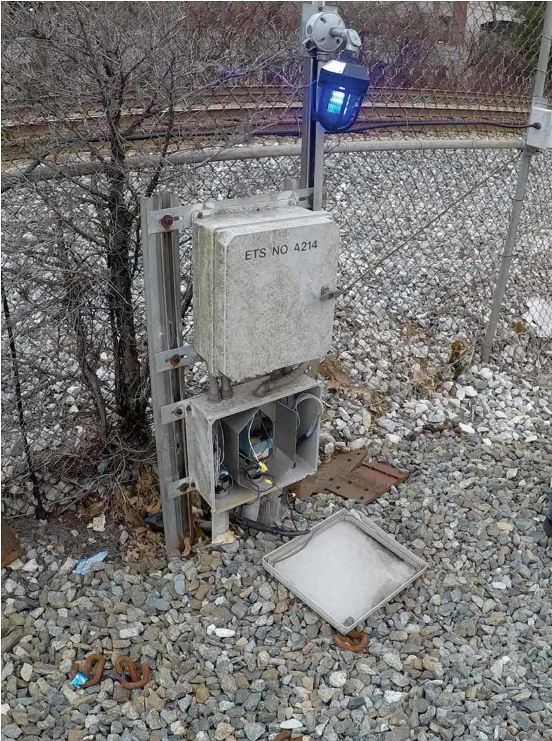
ETS box cover off at CM A2 777+15.
