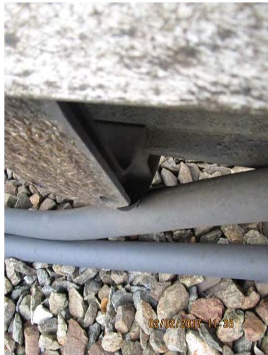
FIGURE 6 - TRK 2 CM 848+00 – CABLES TOO CLOSE TO 3 RD RAIL COVERBOARD BRACKET
