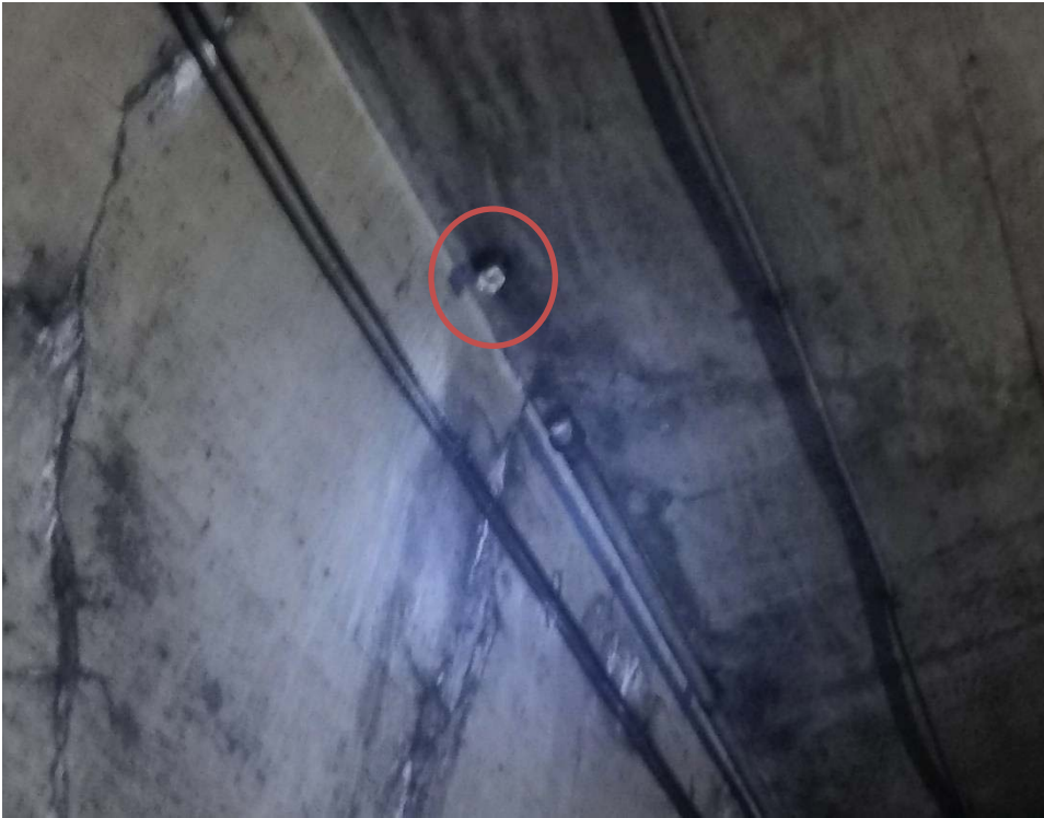
Broken Pipe at A2 451+00
