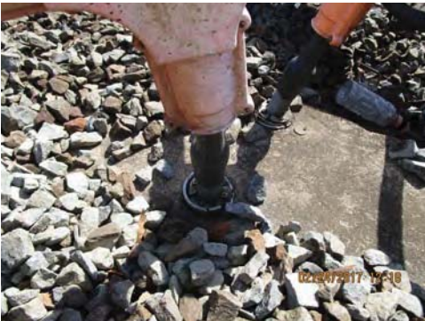
FIGURE 5 - TRK 2 CM 731+00 – CONDUIT/OZ GEDNEY BUSHING BROKEN
