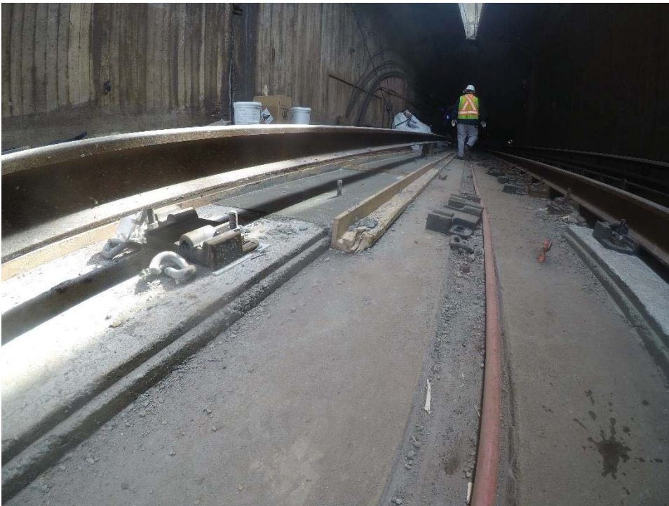
Elevated Rail during grout pad renewal
