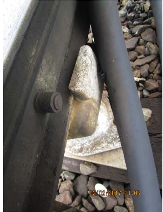
FIGURE 2 - TRK 2 CM 893+00 – DAMAGED CABLE AND PROVIDE CLEARANCE WITH INSULATOR
