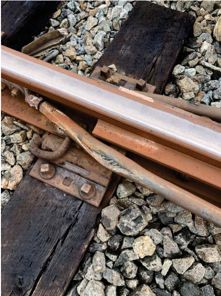
Photo 1: At A2 940+40, damaged negative return bond wire.
