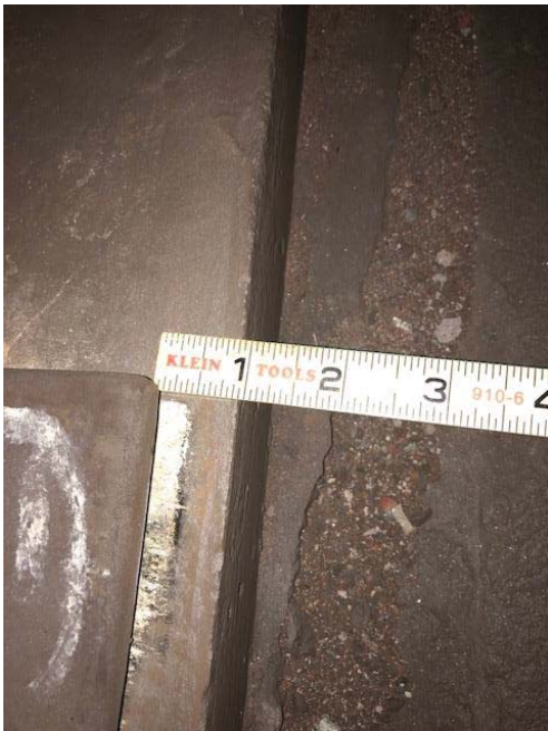
Figure 2: At K1 256+15, left rail field side ¾-inch dynamic movement (57-inches total).
