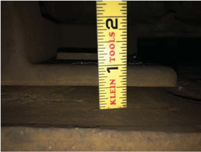
Figure 3: At K1 256+15 left rail, gauge side, 1/2-inch vertical deflection between fastener and grout pad.
