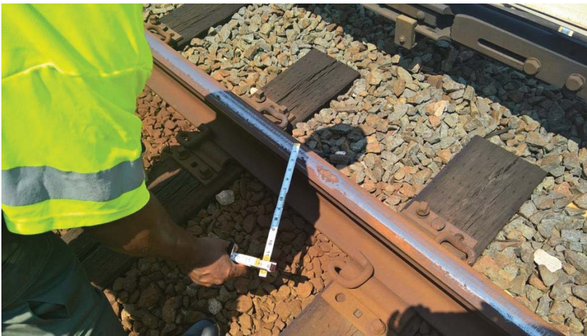
Figure 1: Shelling Condition at J1 616+60.
