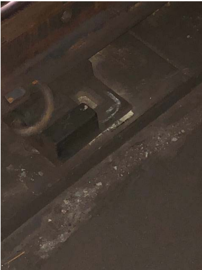
Figure 4: At K1 256+15 left rail, field side, missing stud allowing 1/4-inch dynamic deflection in gauge.
