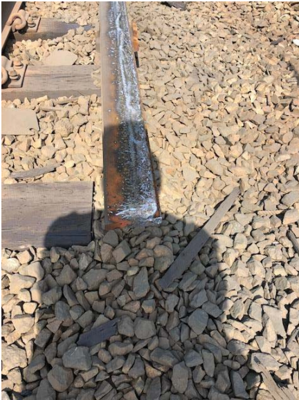
Figure 1: At K1 503+10 collector shoes striking the end of the third rail.
