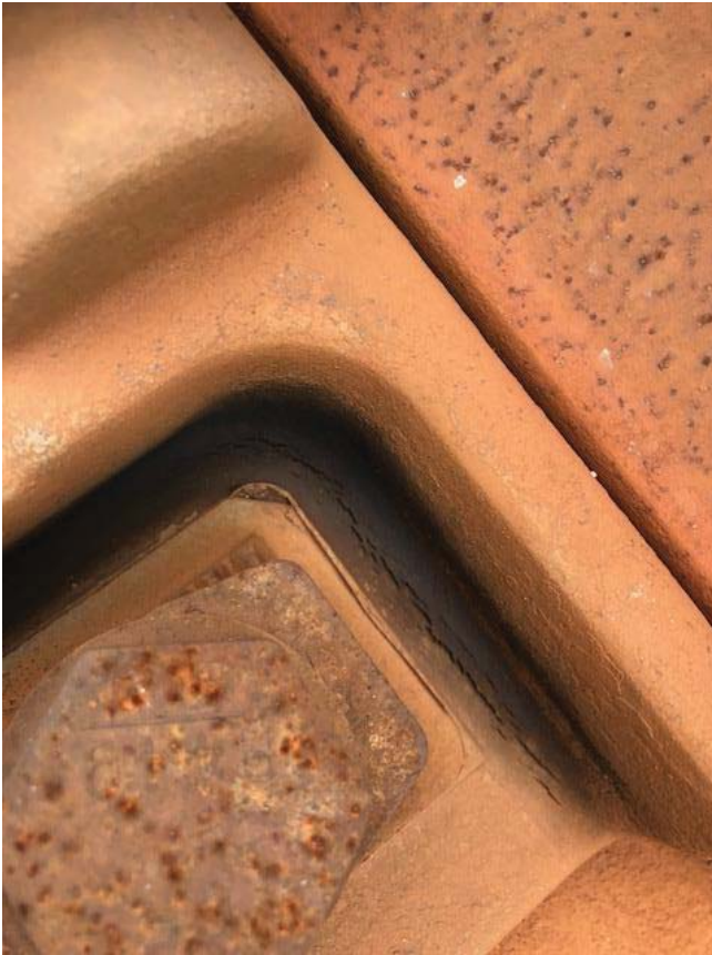
Figure 1: At N1 795+50, elastic fasteners showing signs of deterioration.
