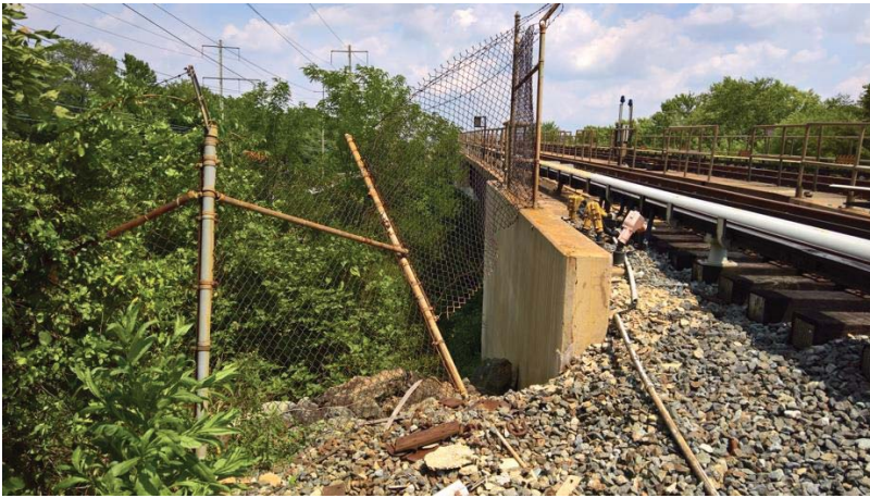
Figure 1: Hole in fence at CM D2 546+50.
