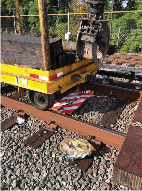
Figure 1: At B2, 254+90, a push cart connected to tie handler TC-237 breached the work zone mat.
