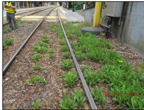
Severely Contaminated Ballasted Area with Vegetation
