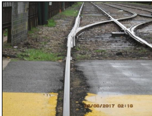
Alignment Issue on Special Trackwork Near Fixed Roadway
