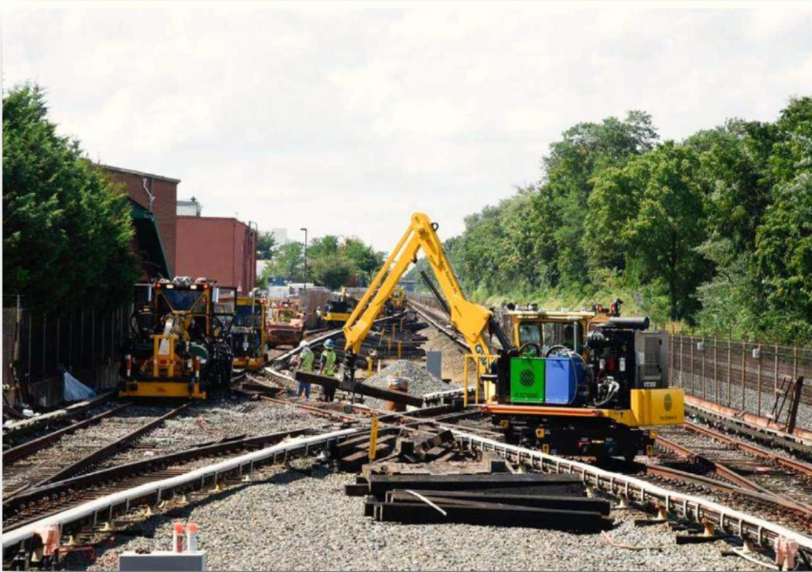
Interlocking Rehabilitation at Twinbrook Station – August 2016
