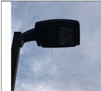
Lens Seal is ha not sealed.
