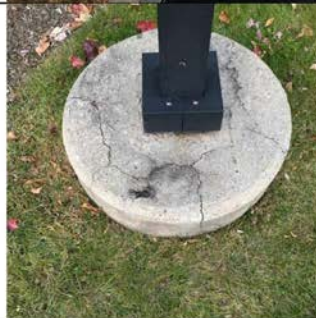
Base is cracked and should be replaced. Located to the right of the front entrance.
