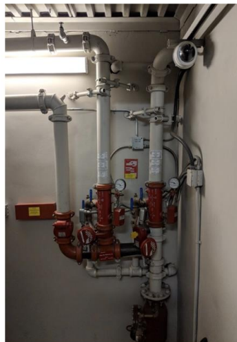
DJTC Fire Riser (1 st floor)
