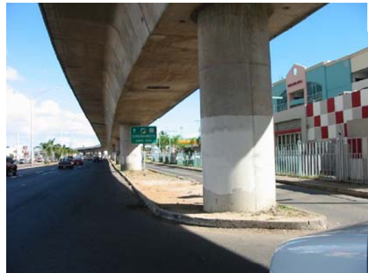
A vehicle could gain close proximity to this column or could ram it at high speed. However, the design may help inhibit an individual from attempting to climb the structure.
