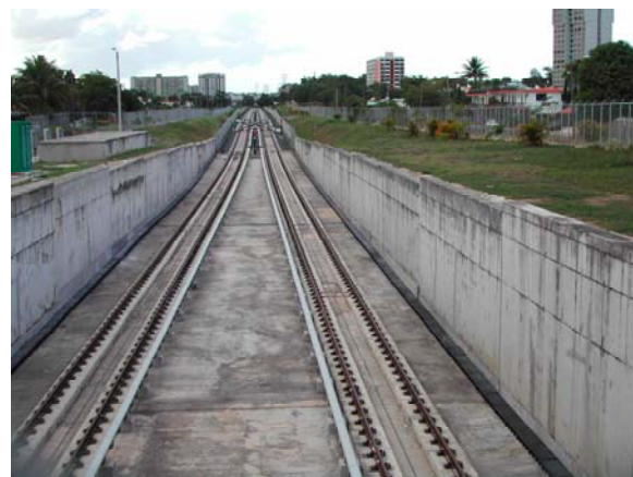
A right-of-way protected with fencing and a grade change (below) is more difficult to access (than above).
