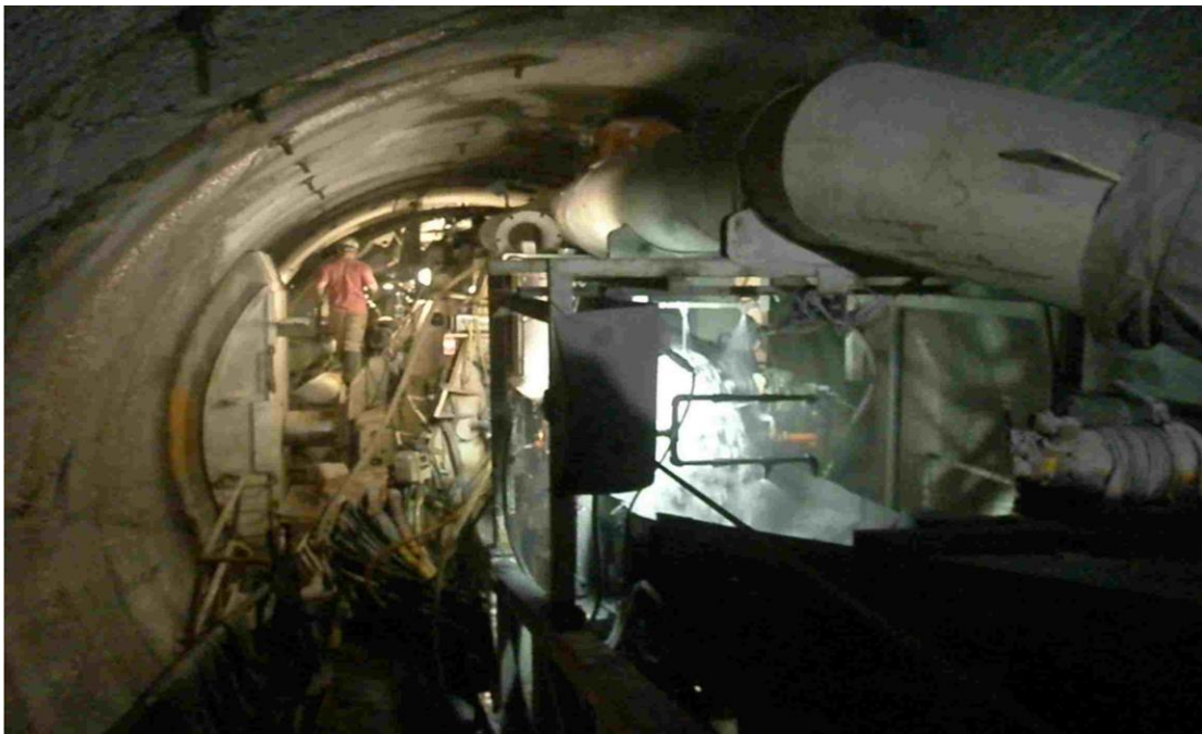
84 th -83 rd St: TBM tunneling is continuing; currently at Station 1192+07 (2982 LF) and installing initial supports (looking south)
