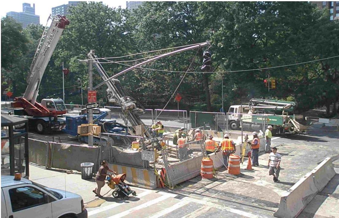
91 st -90 th St: Drilling for installation of freeze pipes for east tunnel (looking west)
