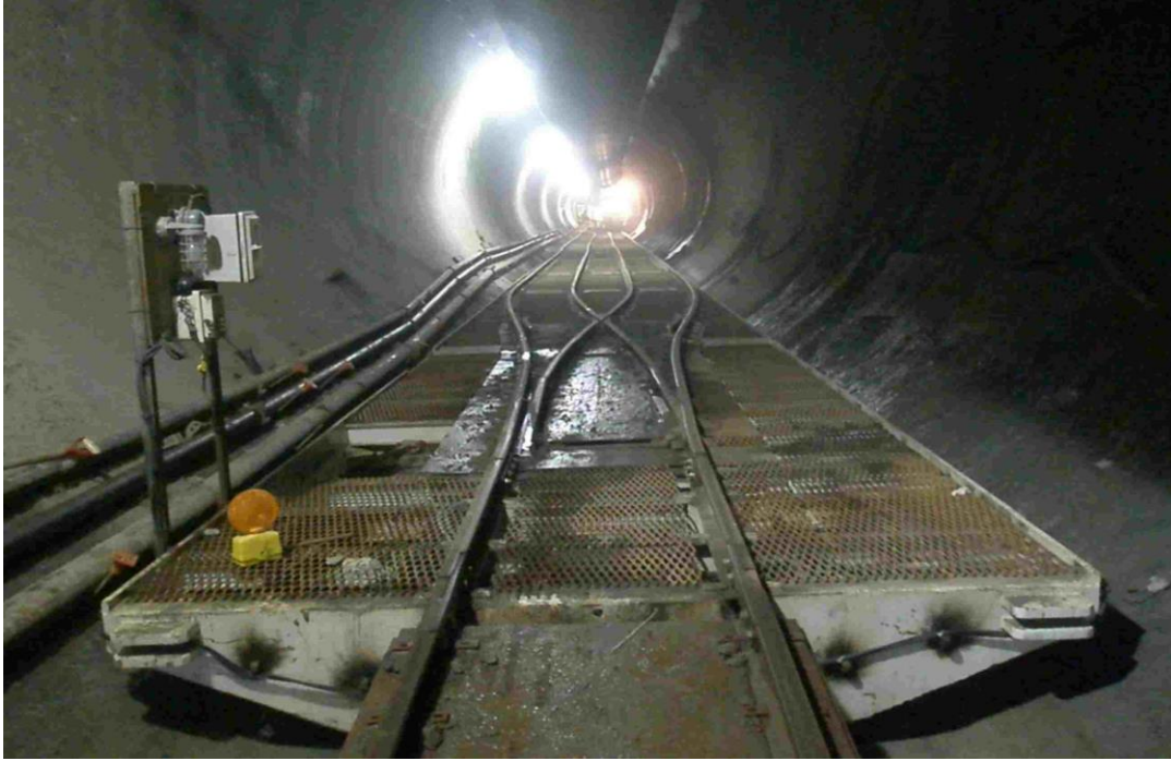
85 th St: Completed installation of the California Switch
