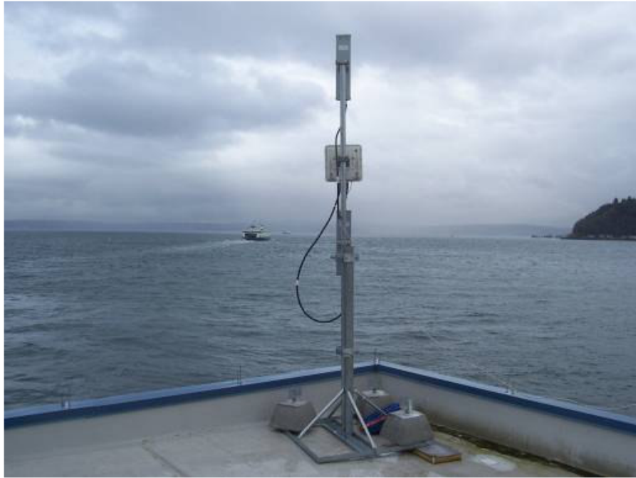
Figure 32 Southworth terminal radio and antenna installation
