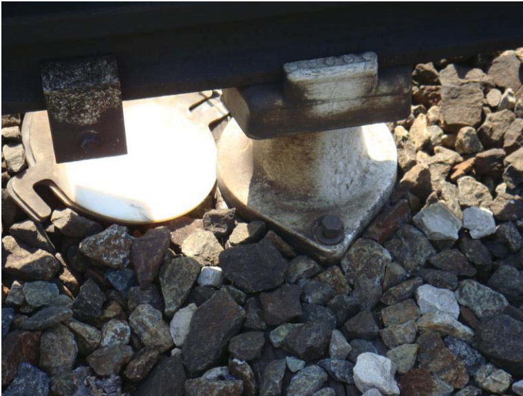
Figure 1 - Loose insulator anchors with dislodged shims
