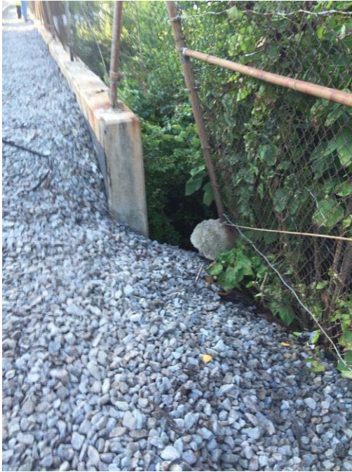
Photo 2 A1-771+00 – Severe soil erosion around wayside Fence post at bridge abutment
