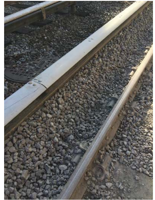
Photo 3 - Excessive ballast under third and rail and against Third Rail
