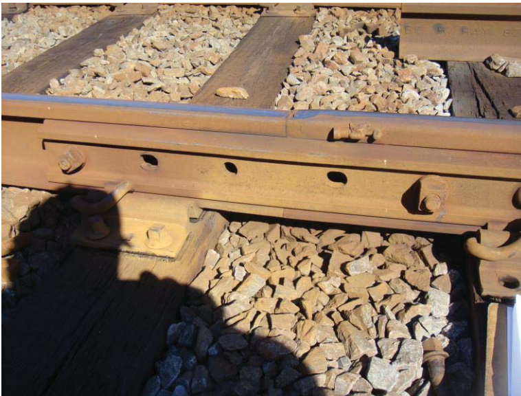
Figure 2 - Missing Bolt at K1 CM604+90
