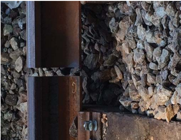
New 39' rail sections requiring weld in 4 locations.
