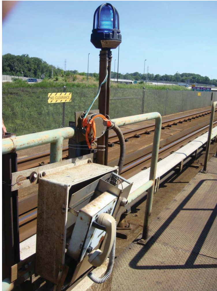
Figure 1 - ETS Box in state of poor repair
