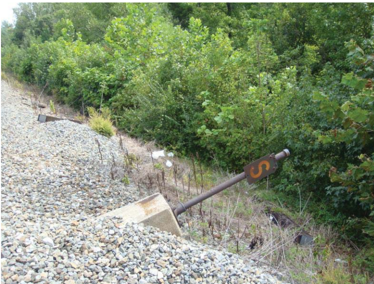
Figure 1 - Toppled Station Marker Sign at D1 CM569+50
