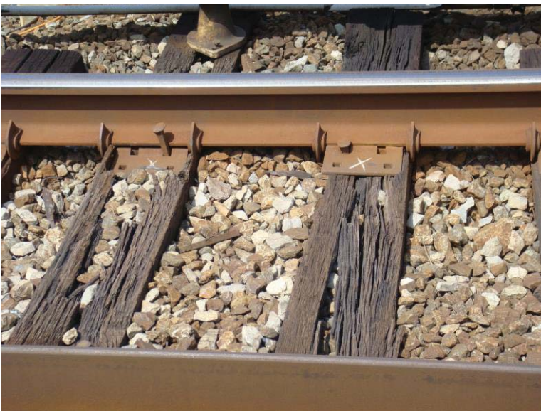
Figure 2 - Deteriorated ties at transition from direct fixation to ballasted track
