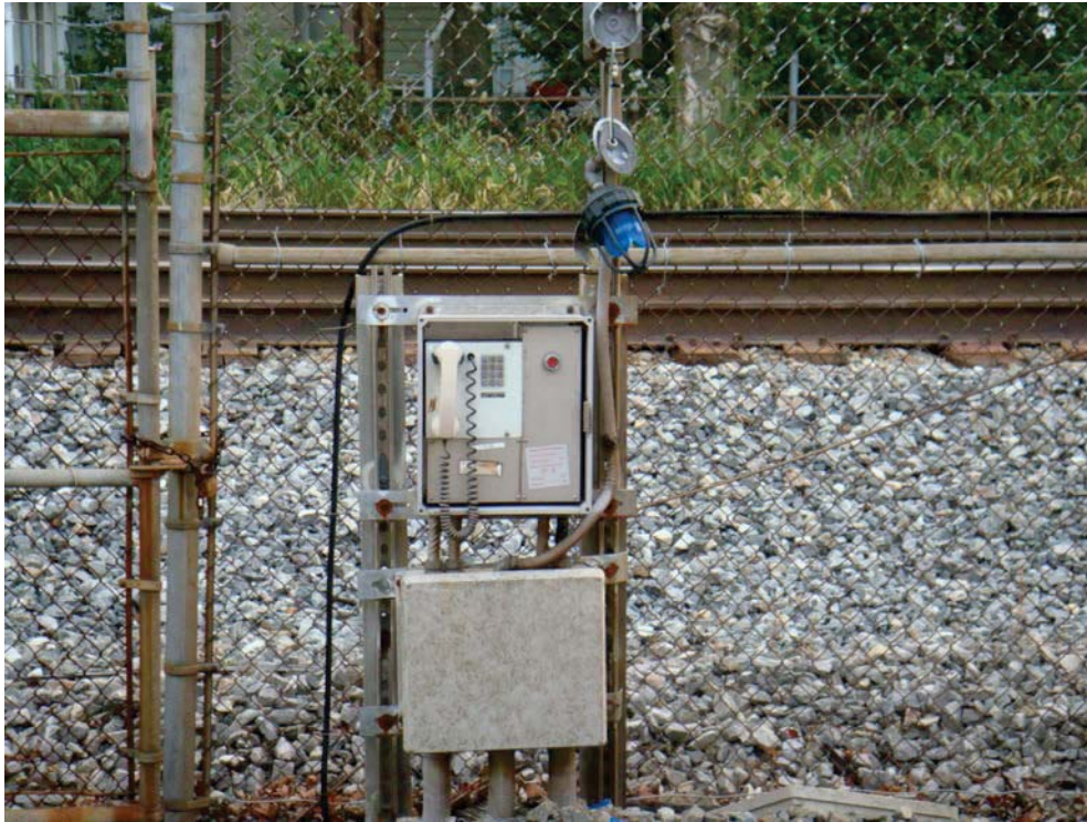
Figure 1 - A2 CM747+00 - ETS Box with no door and broken light
