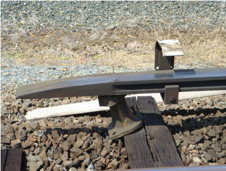
Figure 2 - Unsupported End Approach at D1 CM525+90
