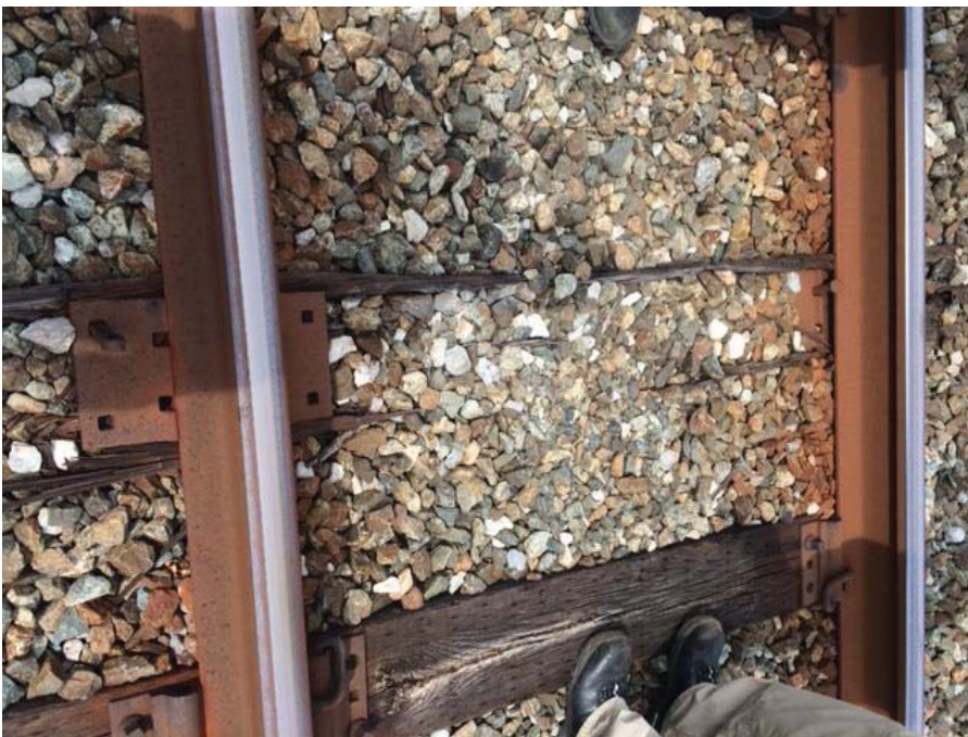
Figure 3 – Deteriorated tie conditions at approx. D1 CM580+00
