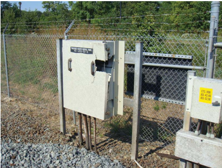
Figure 3 - Damaged Heater Control Box
