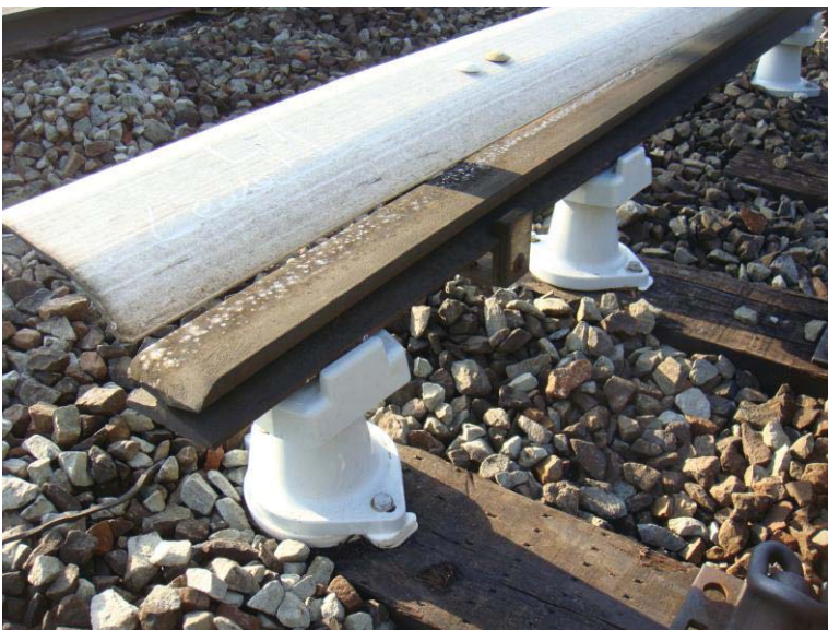
Figure 1 - J2 CM826+60 - shimmed insulator with 3/4" gap under the tie plate
