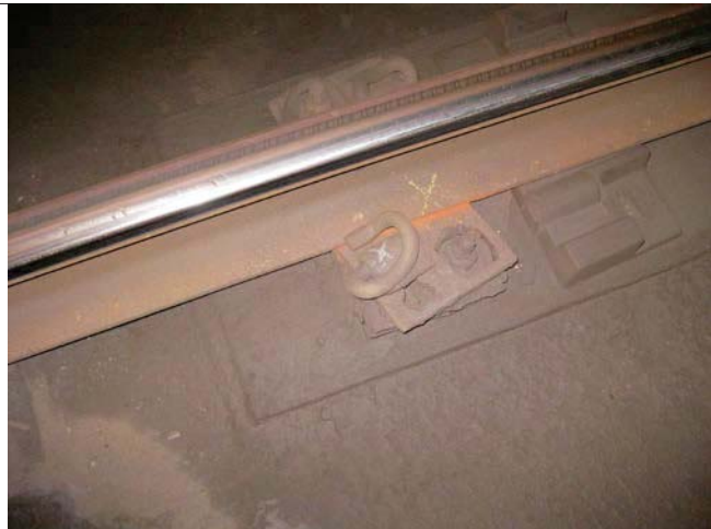
Photo #2 - Common Condition of defective Lord's fasteners
