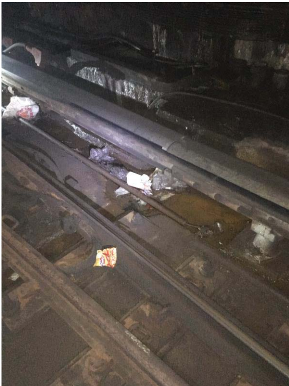
Standing Water at Medical Center Interlocking
