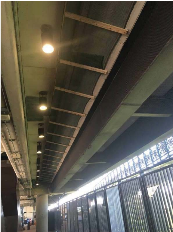
Newly installed netting over Mezzanine
