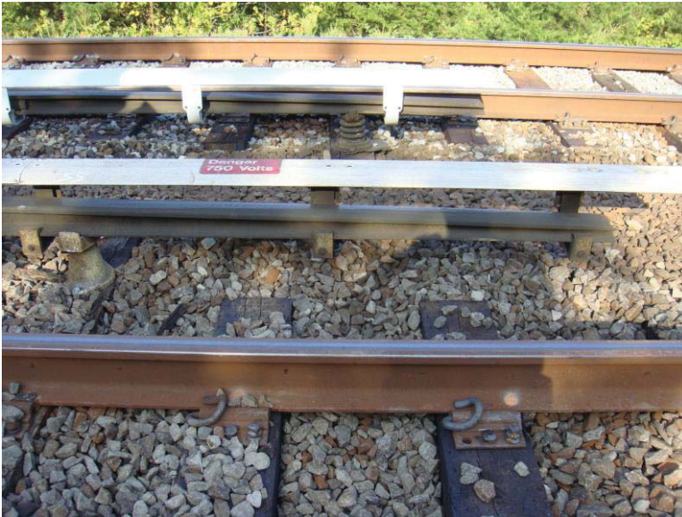
Figure 2 - 70-inch unsupported end approach at J1 CM783+20
