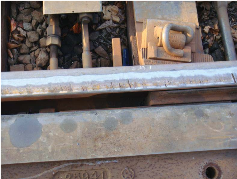
Figure 2 - Switch 17B Stock Rail Head Checking and Missing House Top Bolt
