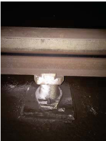
Photo #1 - Common condition of Third rail insulators
