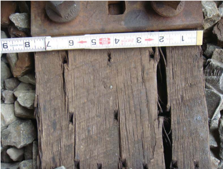
Figure 4 - 7 1/2" tie - note the split at 2" where the screw spike is
