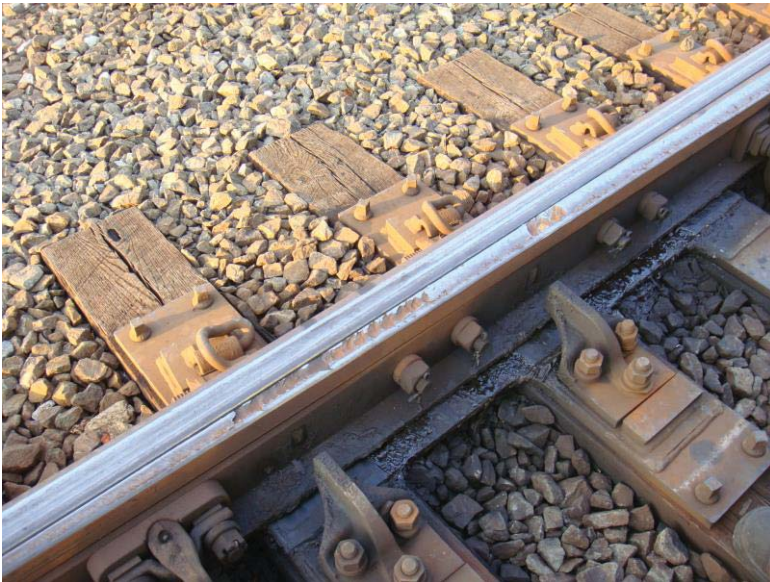
Figure 1 - Switch 17B Head Checking
