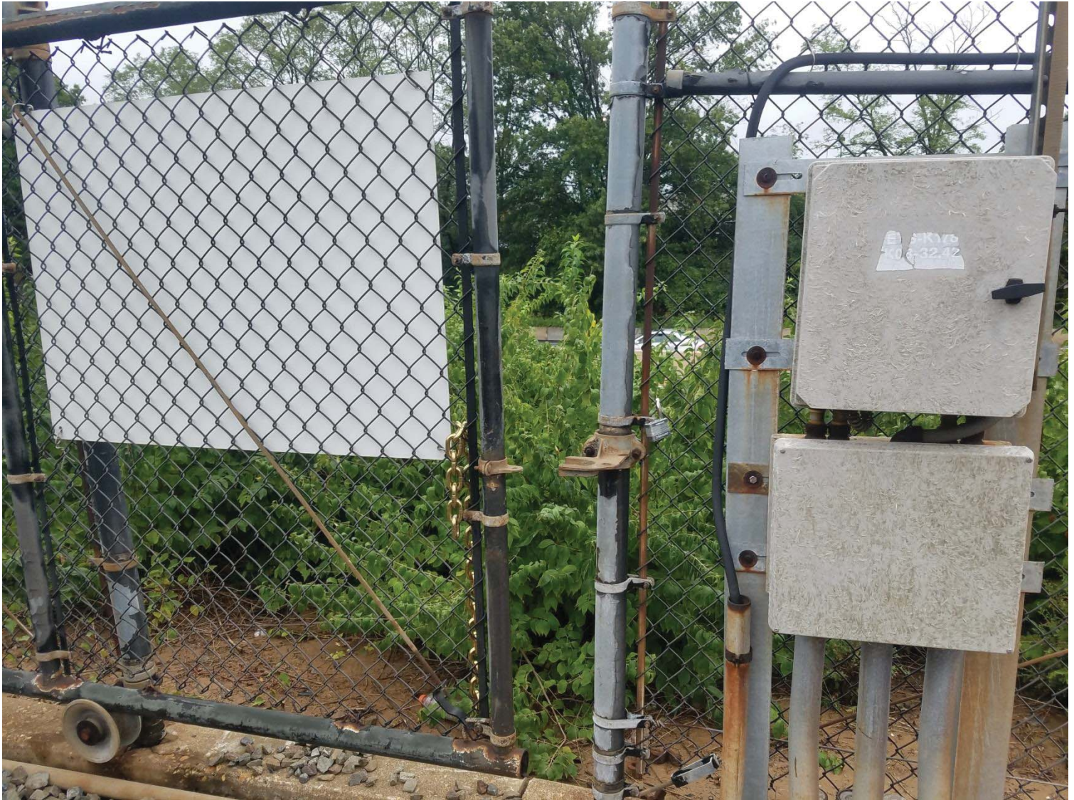
Chain Marker K-771+25 Access gate EEE K-2-771 was unsecure (the chain was to short)
