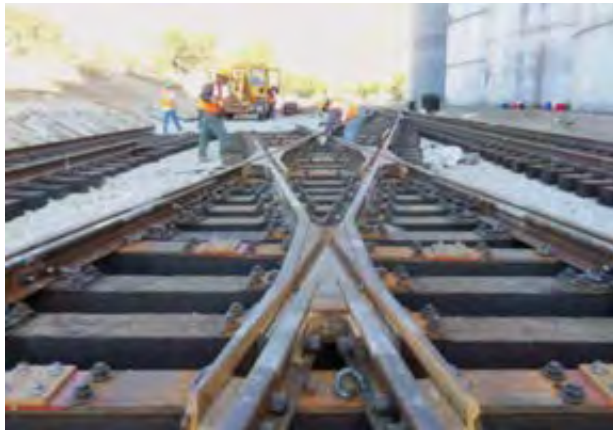
Railway maintenance of Utah Transit Authority's system (Image courtesy of UTA)
