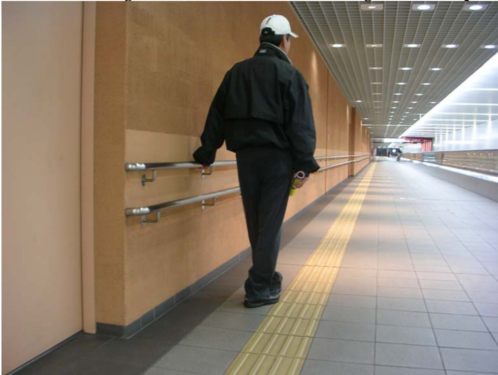
Figure 6 Different Height Handrails and Tactile Flooring, Haneda Airport Tokyo
