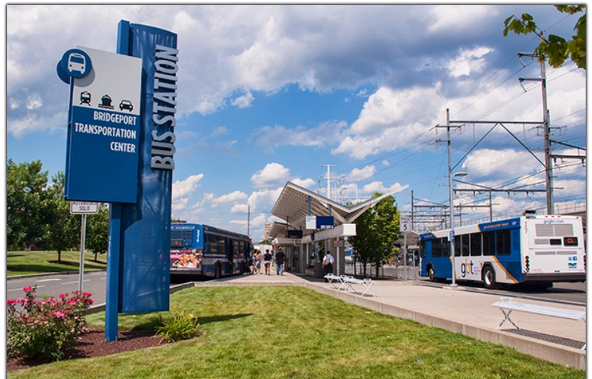
GBT multimodal transportation center
