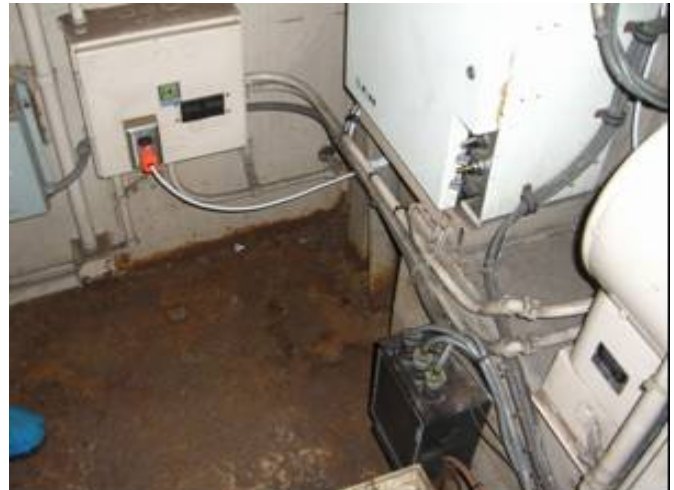
Figure 22: Proxim pre-WiMAX Station in Locomotive V02
