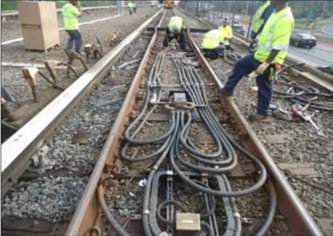
CIP 0024 SafeTrack Project – Surge No. 9 “Installation of new negative return cables” within the gage of Track #1 near Vienna Station, at 9 a.m., October 19, 2016.
