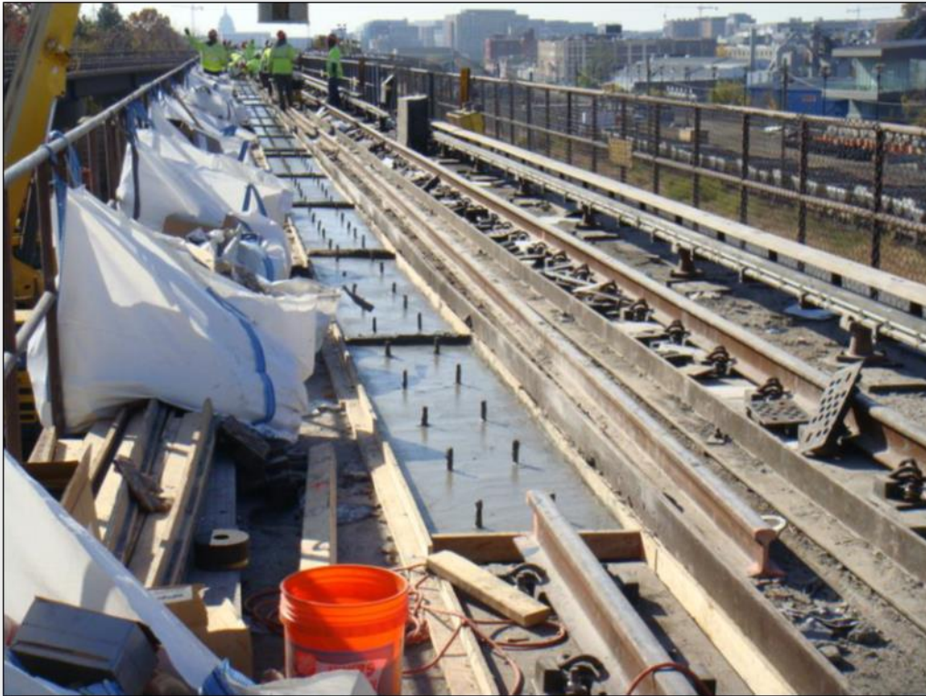
CIP 0024 SafeTrack Project – “Construction of new grout pads just south of Rhode Island Avenue Station on Track 2 of the Red Line during Surge 10,” November 11, 2016.
