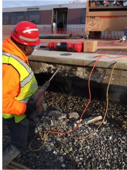
CIP 0024 SafeTrack Project – Force Account labor performing structural repairs to East Falls Church Track 1 platform edge during Surge 11 on December 2, 2016. Photos courtesy of SafeTrack Team.
