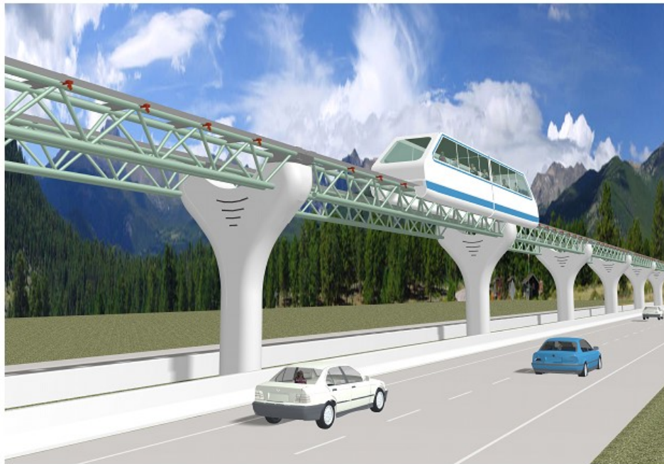
Figure 7. Tubular Steel Space Truss
