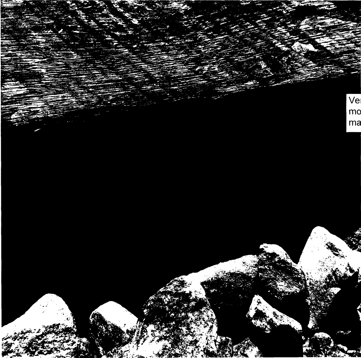
B06-08 SIGNAL FOWL BALLAST CONDITION ALLOWING VERTICAL DEFLESTION AS EVIDENT FROM THE BALLAST MARKS RUBBING AGAINST THE TIES UNDER DYNAMIC CONDITIONS
