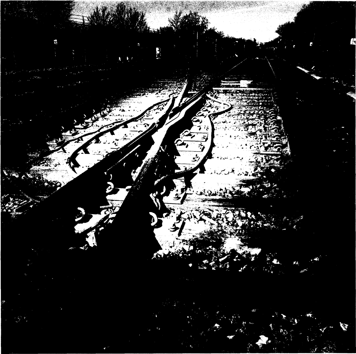
B-07, SWITCH 1A FOWL BALLAST CONDITIONS
