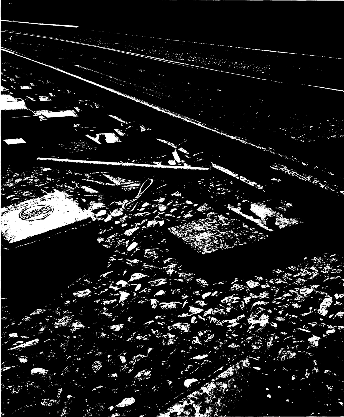
B-06 SWITCH NUMBER 1B OVERALL VIEW OF FOWL BALLAST CONDITION
