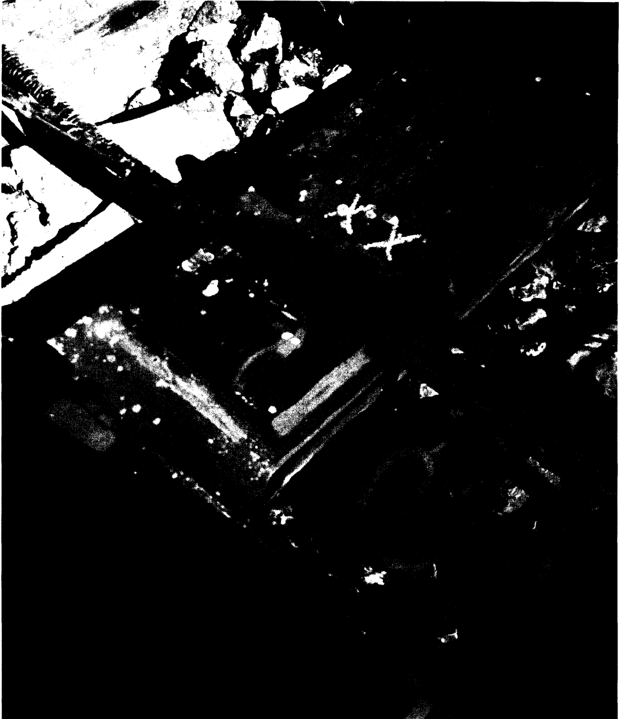
B-06 SWITCH NUMBER 1A FROG BRACE, (WEDGE MISSING) PANDRAL CLIPS NOT ATTACHED
