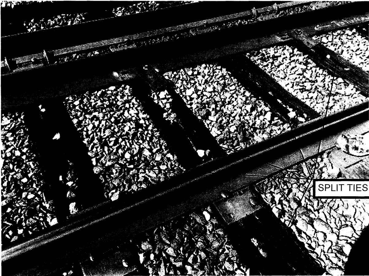
SPLIT / DEFECTIVE CROSSTIES
