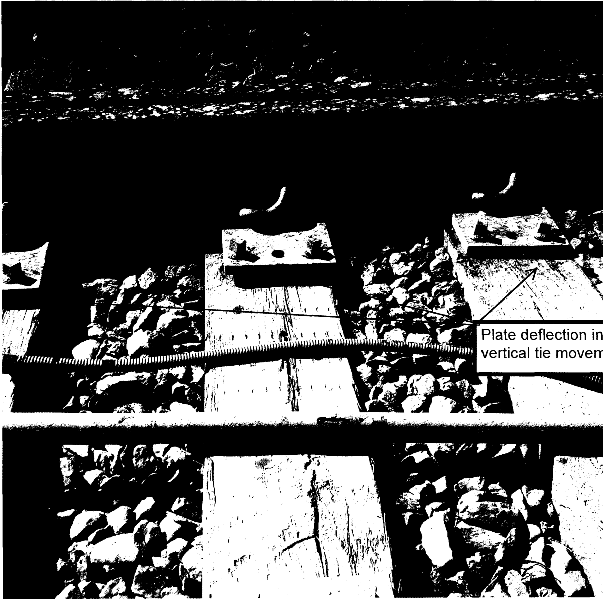
B-07 SWITCH NUMBER 1A FOWL BALLAST CONDITIONS AT FROG NOTE GAP BETWEEN TIE AND PLATE ADDING TO MOVEMENT UNDER DYNAMIC CONDITIONS
