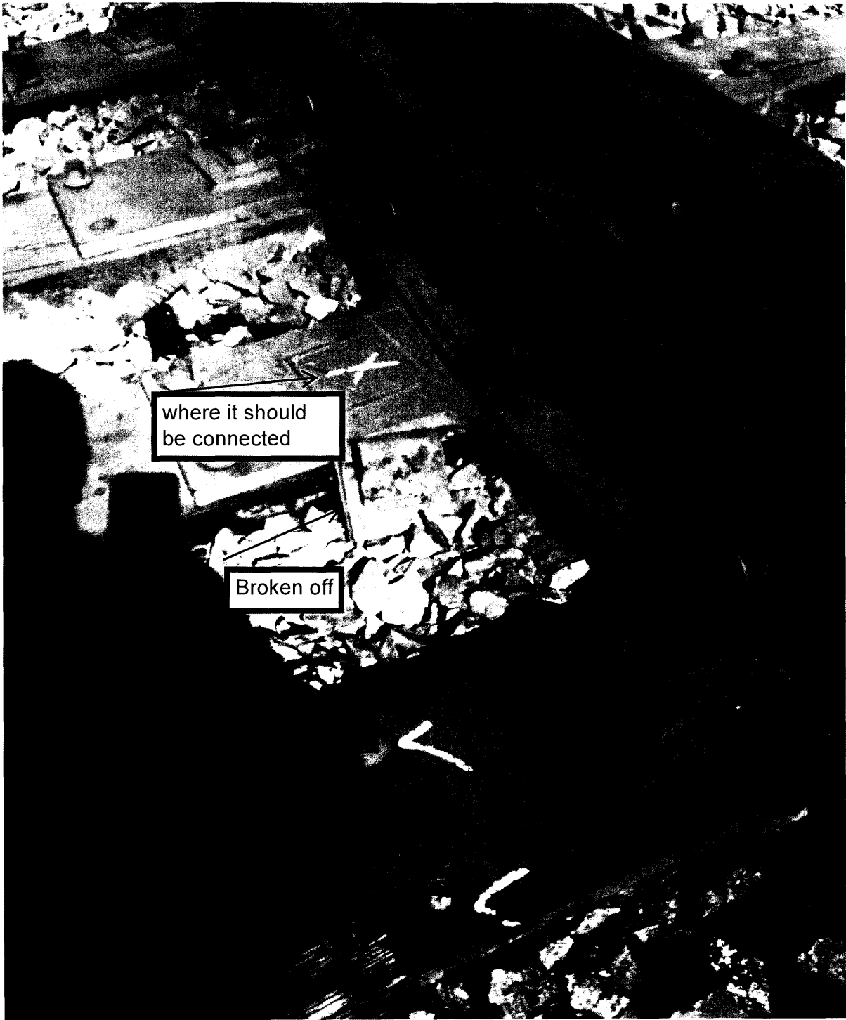
B-06 NUMBER 7 SWITCH LEFT SIDE OF FROG SHOWS A BROKEN BRACE PLATE
