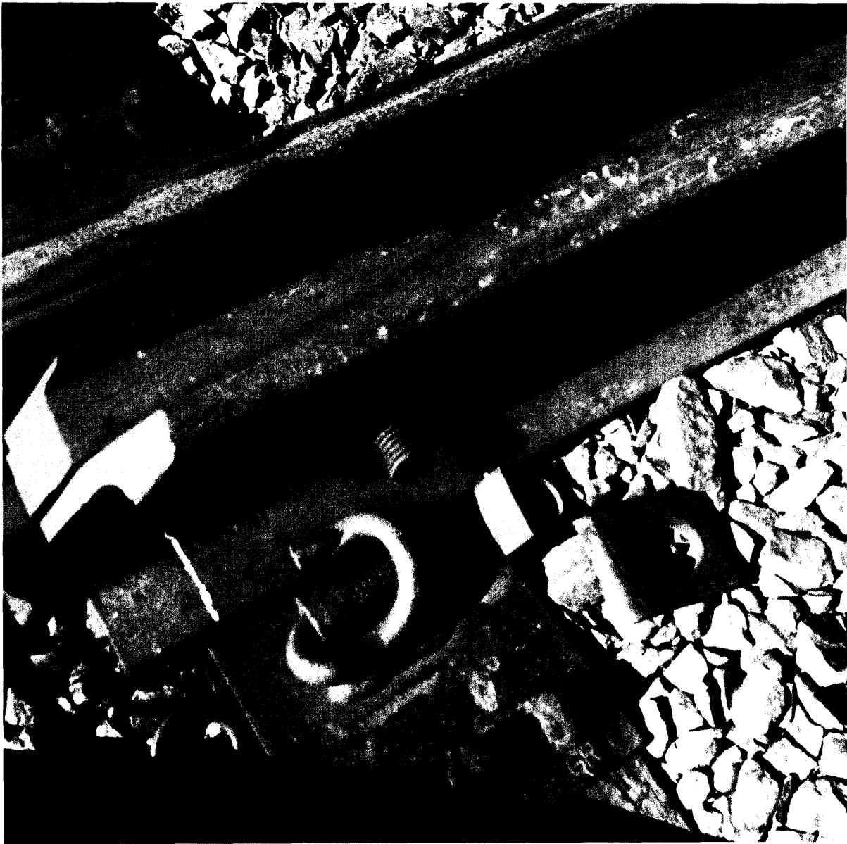
B-06 SWITCH NUMBER 1A RIGHT SIDE SWITCH POINT GUARD RAIL MISSING BOLT ANOTHER BOLT WAS FOUND LOOSE.
