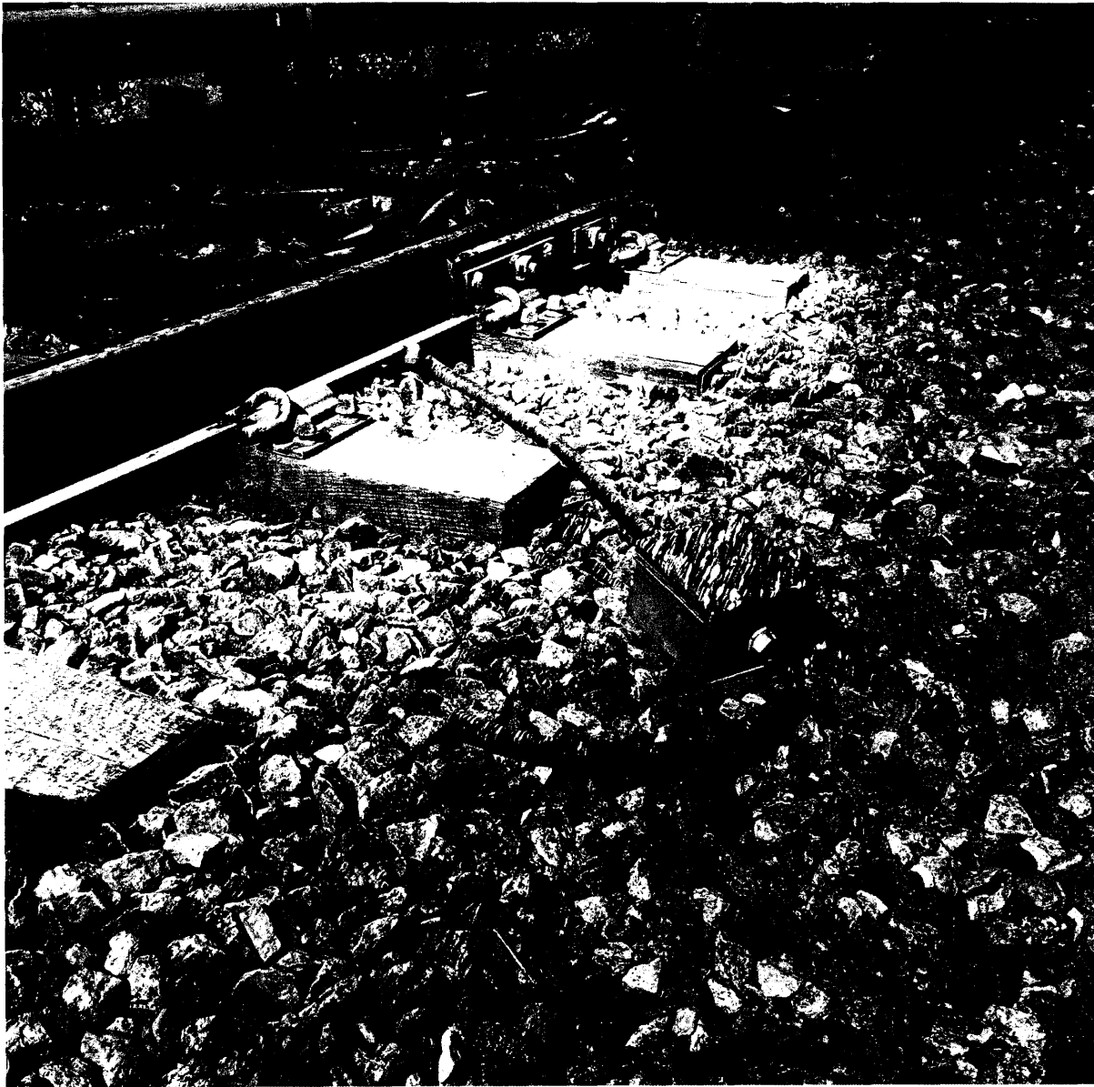
B-06-08 SIGNAL FOWL BALLAST CONDITION AT INSULATED JOINTS
