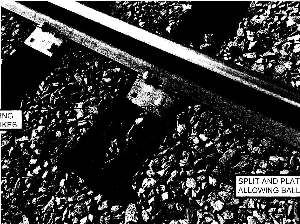
SPLIT CROSSTIE ALLOWING BALLAST TO WORK THROUGH
