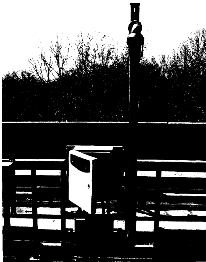
Photo showing broken latch on open cabinet door #ETSF159
