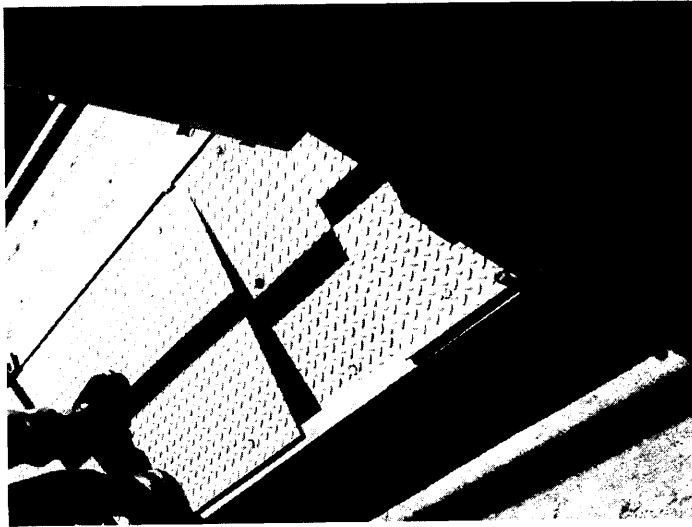
Photo showing Insecure walkway plate at trackside heater control box HCFOE33-2
