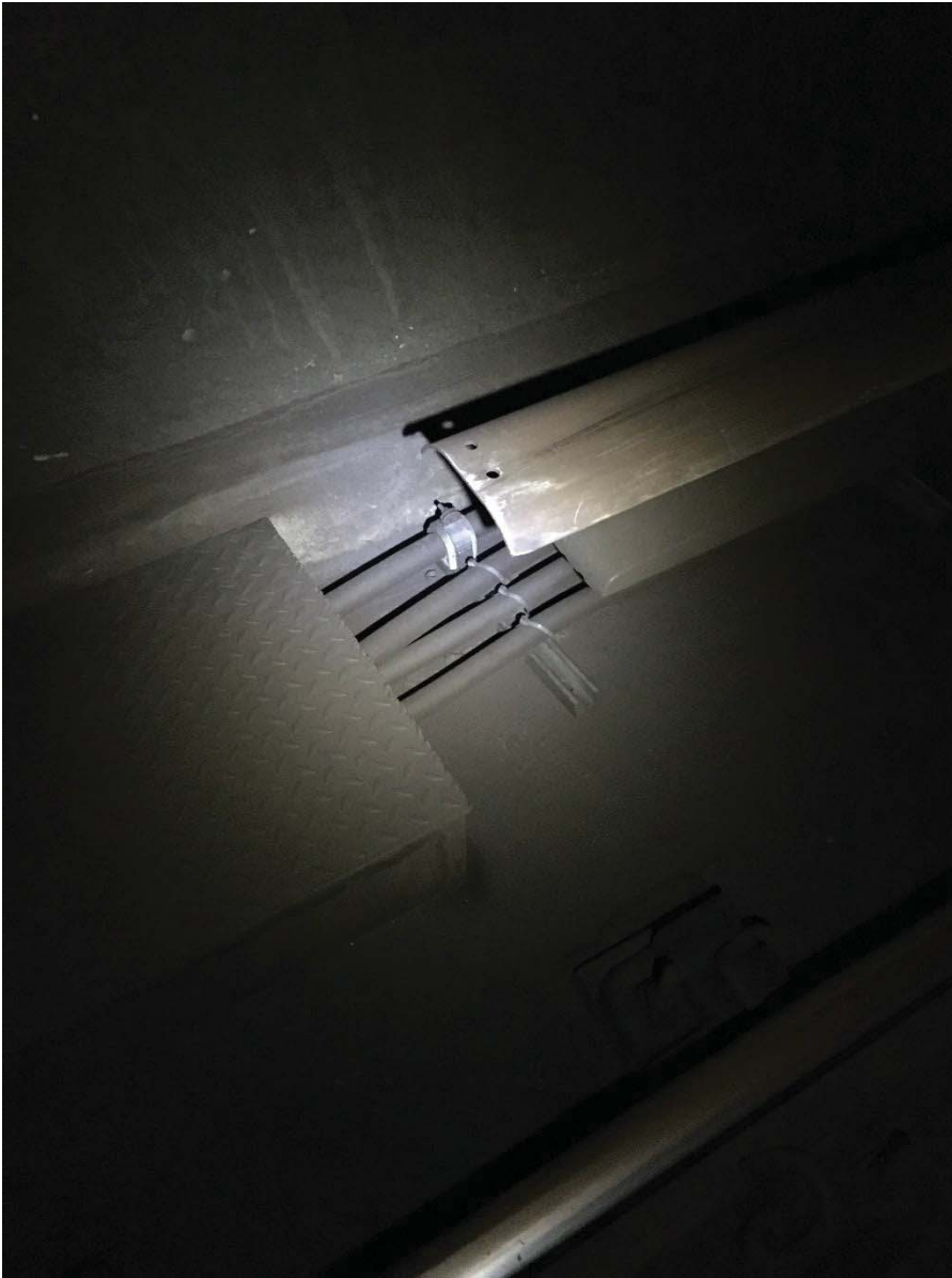
Expansion Cables improperly secured to fiberglass strut
