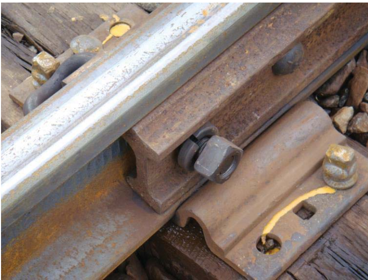
Figure 2 - K1 CM744+00 - Right Rail Joint Bar Bolt Loose
