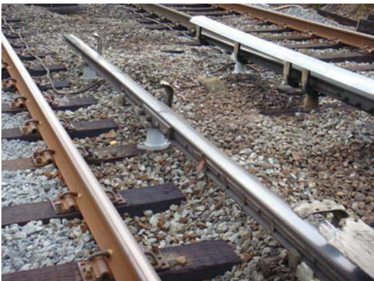
Figure 15 - J1 CM826+20 - End Approach No Coverboard
