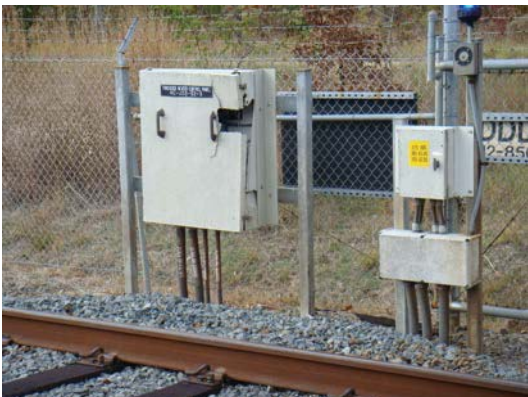
Figure 21 - Heater Control Box - HC-J03-52-3 - still not repaired
