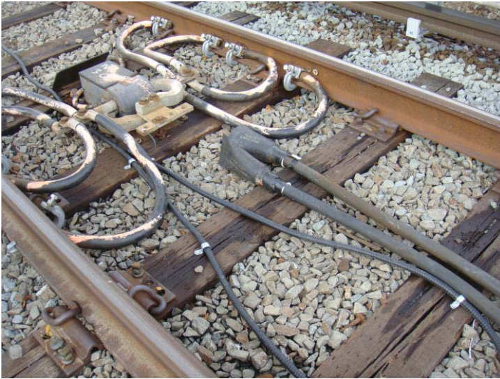
Figure 1 - K1 CM673+80 - Cross Bond not connected
