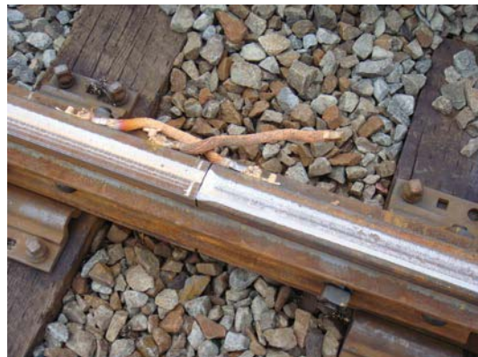
Figure 18 - J1 CM828+00 Left Rail - One C-Bond Detached
