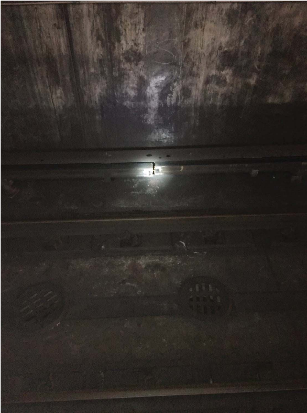
Rail Break noted just outside the Potomac Ave. station
