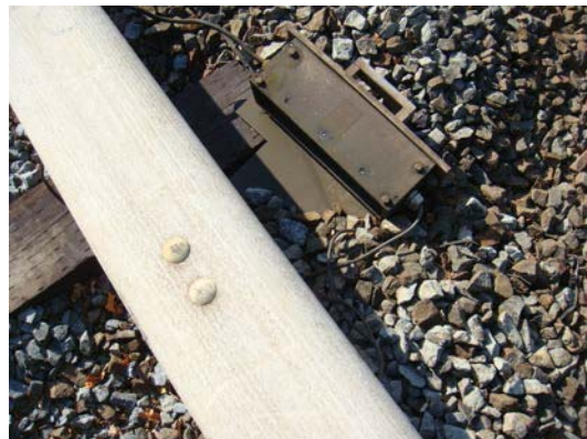
Figure 6 - J1 CM777+40 - Heater Control Fuse Box
