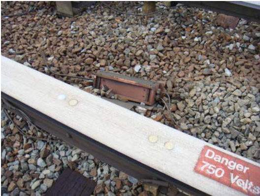
Figure 13 - J1 CM824+80 - Heater Control Fuse Box
