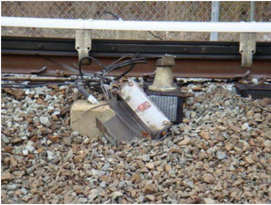
Figure 25 - J2 CM865+60 - Heater Control Fuse Box
