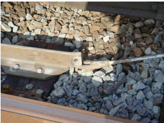
Figure 3 - J1 CM731+60 - 3rd Rail Anchor Arm Off
