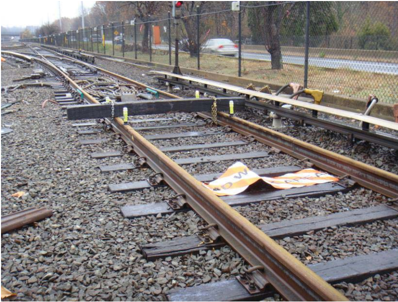
Figure 3 - RWP Work Zone Set-up - East End of Work Zone
