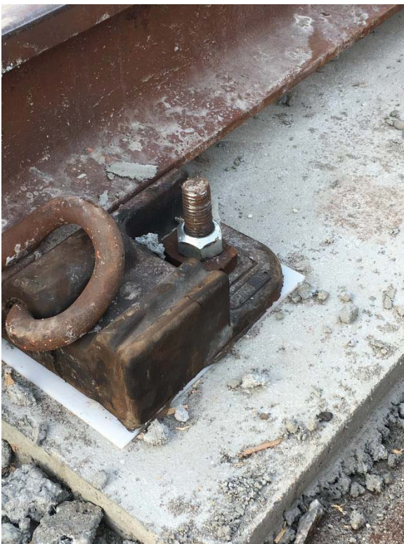
New nut style with more beveled edge
