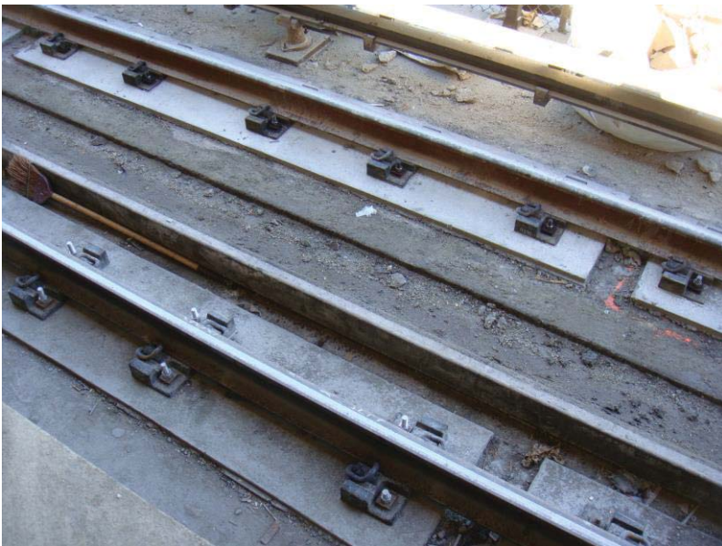
Figure 1 - New Grout Pads at B04
