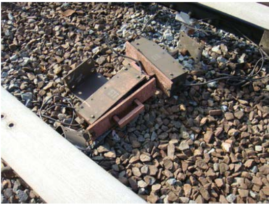
Figure 8 - J1 CM784+00 - Heater Control Fuse Box
