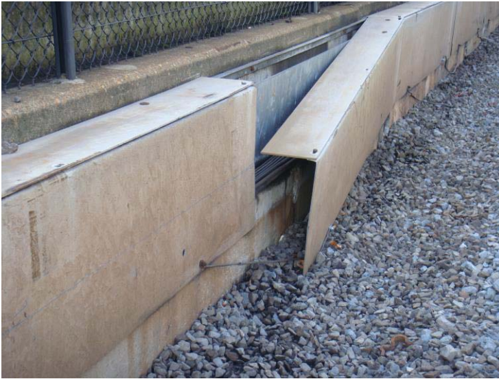
Figure 3 - K1 CM754+00 Cable Trough Cover Dislodged
