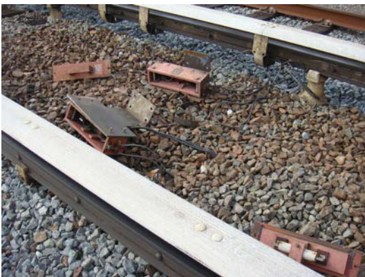
Figure 20 - J1 CM842+70 - Heater Control Fuse Box
