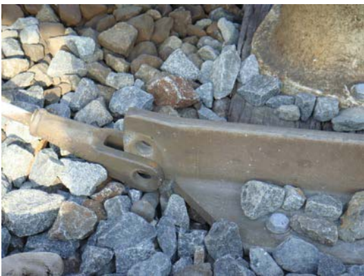
Figure 2 - J1 CM726+50 - 3rd Rail Anchor Arm Off
