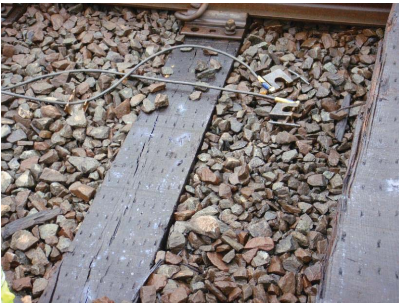
Figure 3 - Shunt Strap not attached at East End of the Work Zone
