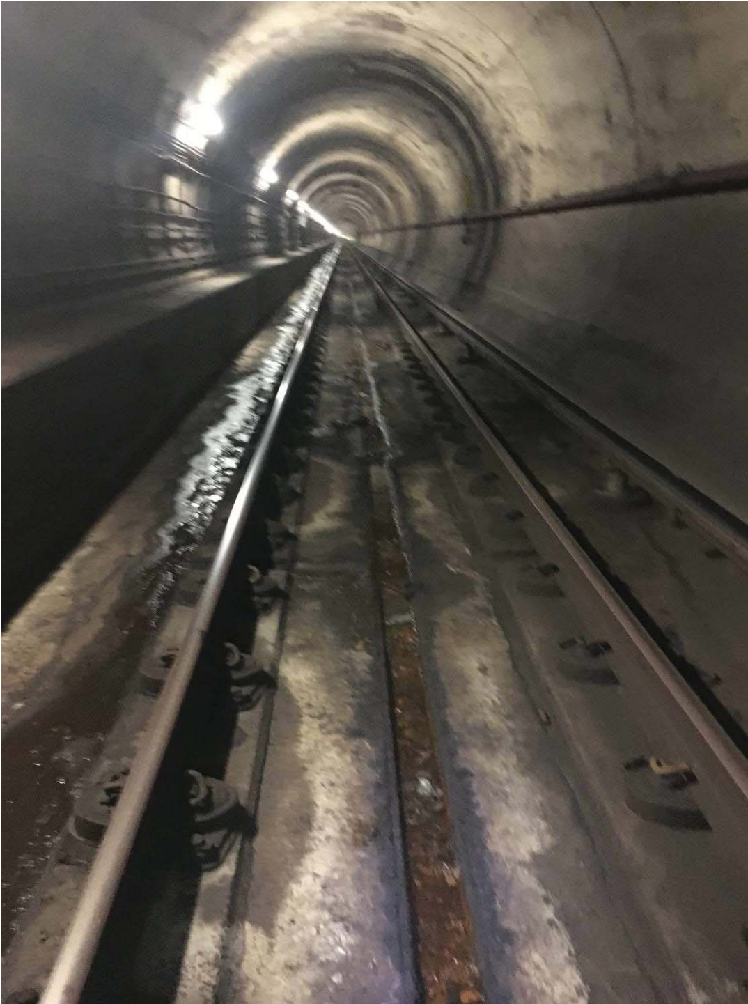
Standing Water due to clogged drains E1 196+00
