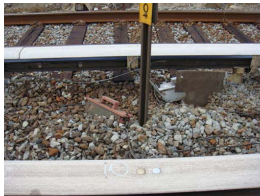
Figure 17 - J1 CM827+00 - Heater Control Fuse Box
