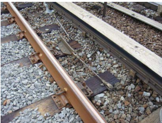
Figure 14 - J1 CM826+00 - 3rd Rail Anchors
