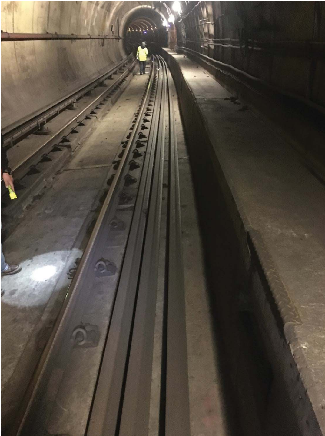
CWR Pieces encumbering access to Safety Walk from the ROW
