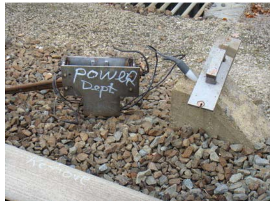
Figure 24 - J1 CM865+60 - Heater Control Fuse Box
