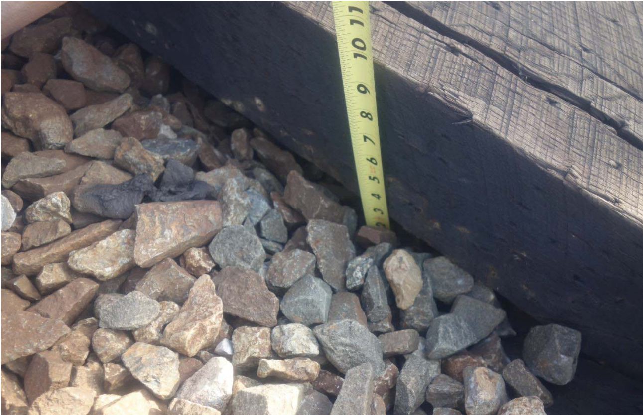
Low Crib Ballast at B2 138+00
