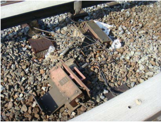
Figure 7 - J1 CM781+50 - Heater Control Fuse Box
