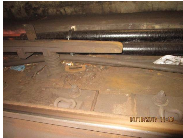
FIGURE 5 - TRK 1 CM 025+00 – TRASH SURROUNDING JUMPER CABLES THAT ARE REPLACING NORMAL FEEDER CABLES DUE TO A TIE BREAKER REHAB. TRASH BY 3 RD RAIL END APPROACH
