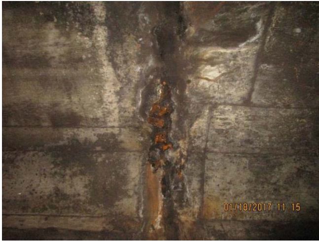
FIGURE 7 - TRK 1 CM 022+00 – WATER INTRUSION IN TUNNEL AND LEAKING ON 3 RD RAIL
