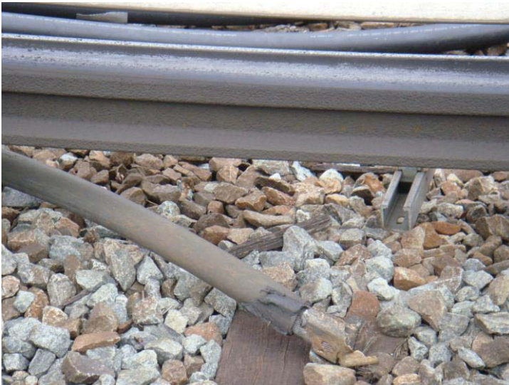
Figure 1 - K1 CM588+80 - Expansion Joint Cable - WMATA repaired immediately
