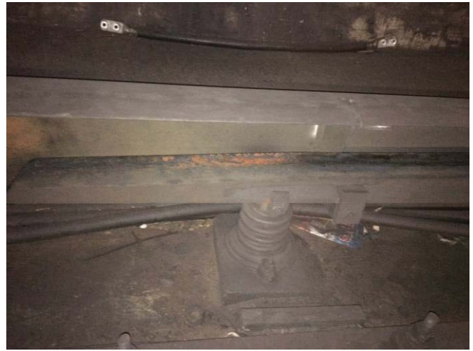
FIGURE 14 - TRK 2 CM 025+00 - 3 RD RAIL END APPROACH SHOULD BE REPLACED.
