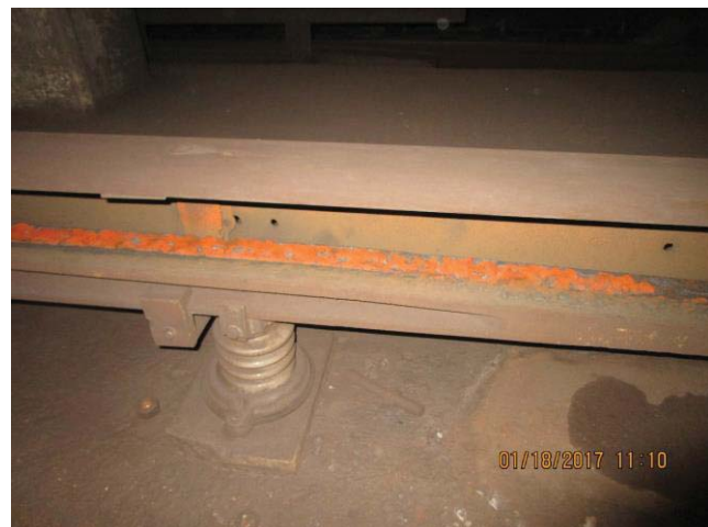
FIGURE 6 - TRK 1 CM 024+00 – 3 RD RAIL COVERBOARD MISSING AND TRASH BY 3 RD RAIL END APPROACH. 3 RD RAIL END APPROACH CORRODED AND NEEDS TO BE REPLACED
