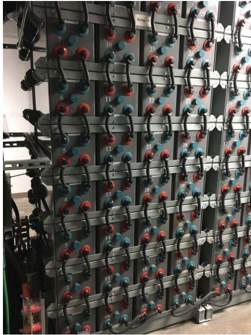
FIGURE 3 – 1 OF 4 BATTERY BANKS (144 BATTERIES PER BANK CONNECTED IN SERIES)
