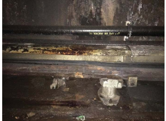
FIGURE 7 - TRK 1 CM 022+00 – WATER INTRUSION IN TUNNEL AND LEAKING ON 3 RD RAIL
