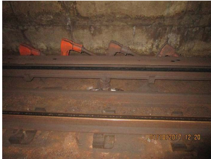
FIGURE 15 - TRK 2 CM 043+00 – DEBRIS SURROUNDING FEEDER CABLES
