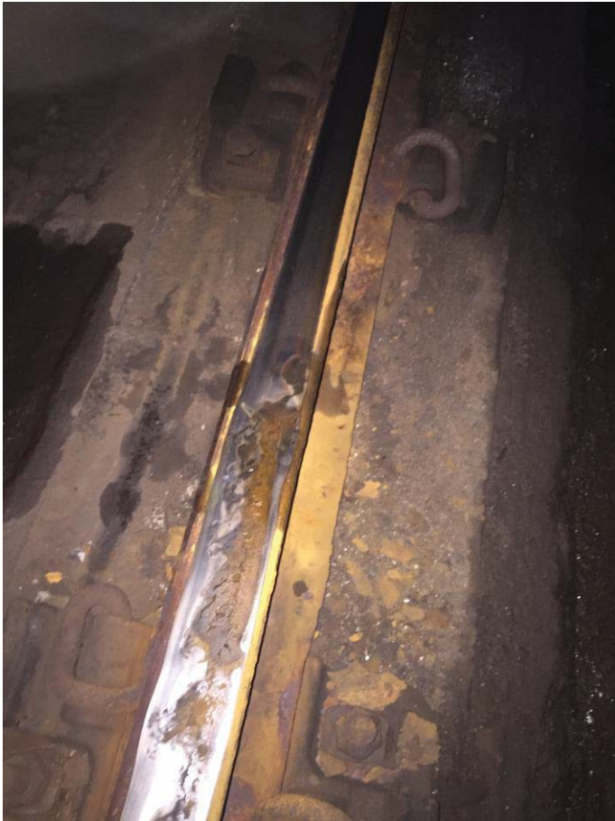
Damage to running surface of rail from water
