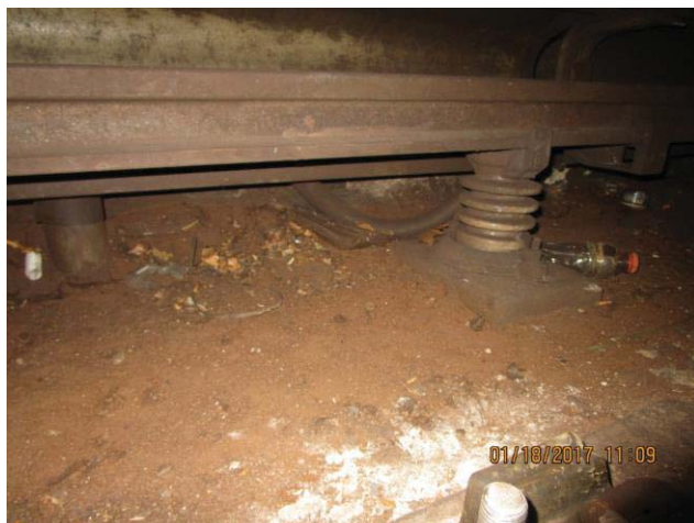
FIGURE 6 - TRK 1 CM 024+00 – 3 RD RAIL COVERBOARD MISSING AND TRASH BY 3 RD RAIL END APPROACH. 3 RD RAIL END APPROACH CORRODED AND NEEDS TO BE REPLACED
