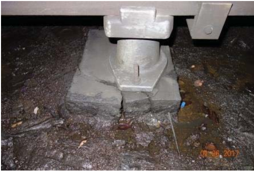
Figure 1: 227+30 cracked third rail grout pad, left rail.
