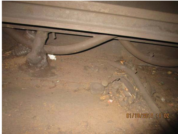
FIGURE 4 - TRK 1 CM 026+00 – TRASH SURROUNDING FEEDER CABLES
