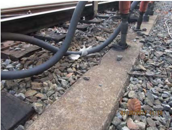
FIGURE 2 - TRK 1 CM 702+00 – OZGEDNEY BUSING NEEDS TO BE REPLACED ON FEEDER CABLE STUB-UP; CABLES LAYING ON THE DECK (BALLAST)
