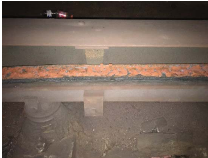
FIGURE 16 - TRK 2 CM 045+00 – 3 RD RAIL END APPROACH NEEDS REPLACEMENT
