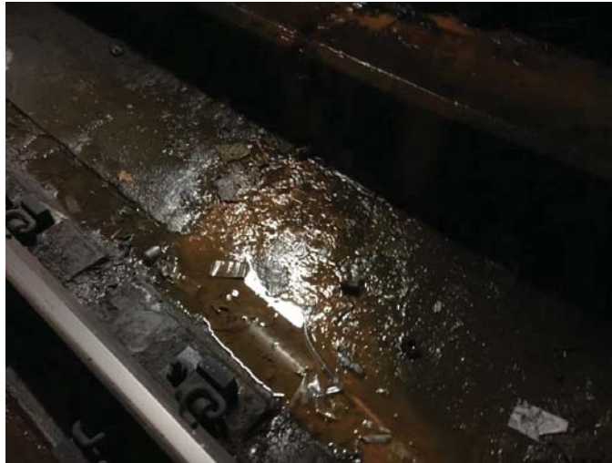
FIGURE 10 - TRK 1 CM 005+00 – WATER INTRUSION IN TUNNEL LEAKING ON SAFETY CATWALK
