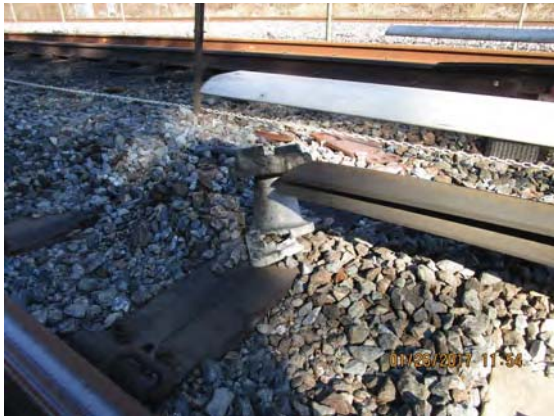
FIGURE 4 - TRK 1 CM 766+00 – 3 RD RAIL POST INSULATOR SUPPORTING THIRD RAIL AS END APPROACH MAY HAVE BEEN SHORTENED; REMOVE UNNECESSARY INSULATOR AS COULD IMPEDE COLLECTOR SHOES OR KNOCK COLLECTOR SHOES OFF TRACK
