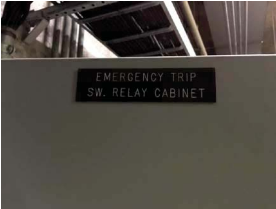
FIGURE 1 – ETS (EMERGENCY TRIP SWITCH) RELAY CABINET AT MEDICAL CENTER TIE BREAKER
