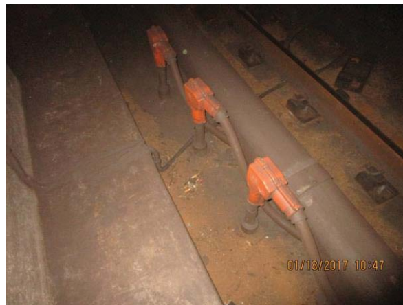
FIGURE 2 – TRK 1 CM 042+00 DEBRIS BY FEEDER CABLES
