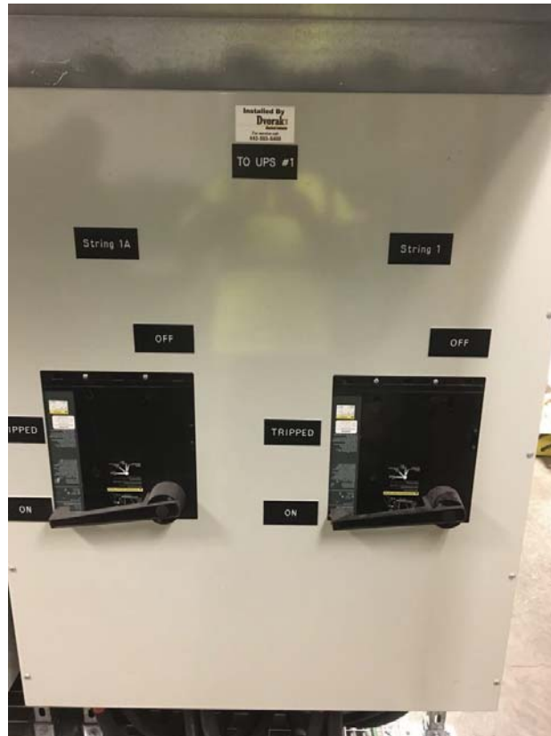
FIGURE 1 – CIRCUIT BREAKERS FOR BATTERY BANK OR STRING 1 AND 1A
