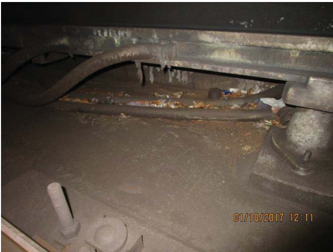
FIGURE 12 - TRK 2 CM 024+00 – DEBRIS SURROUNDING FEEDER CABLES
