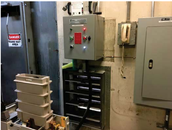
FIGURE 3 – USING TEST CABINET TO TEST OPEN/CLOSE MECHANISM OF CIRCUIT BREAKER
