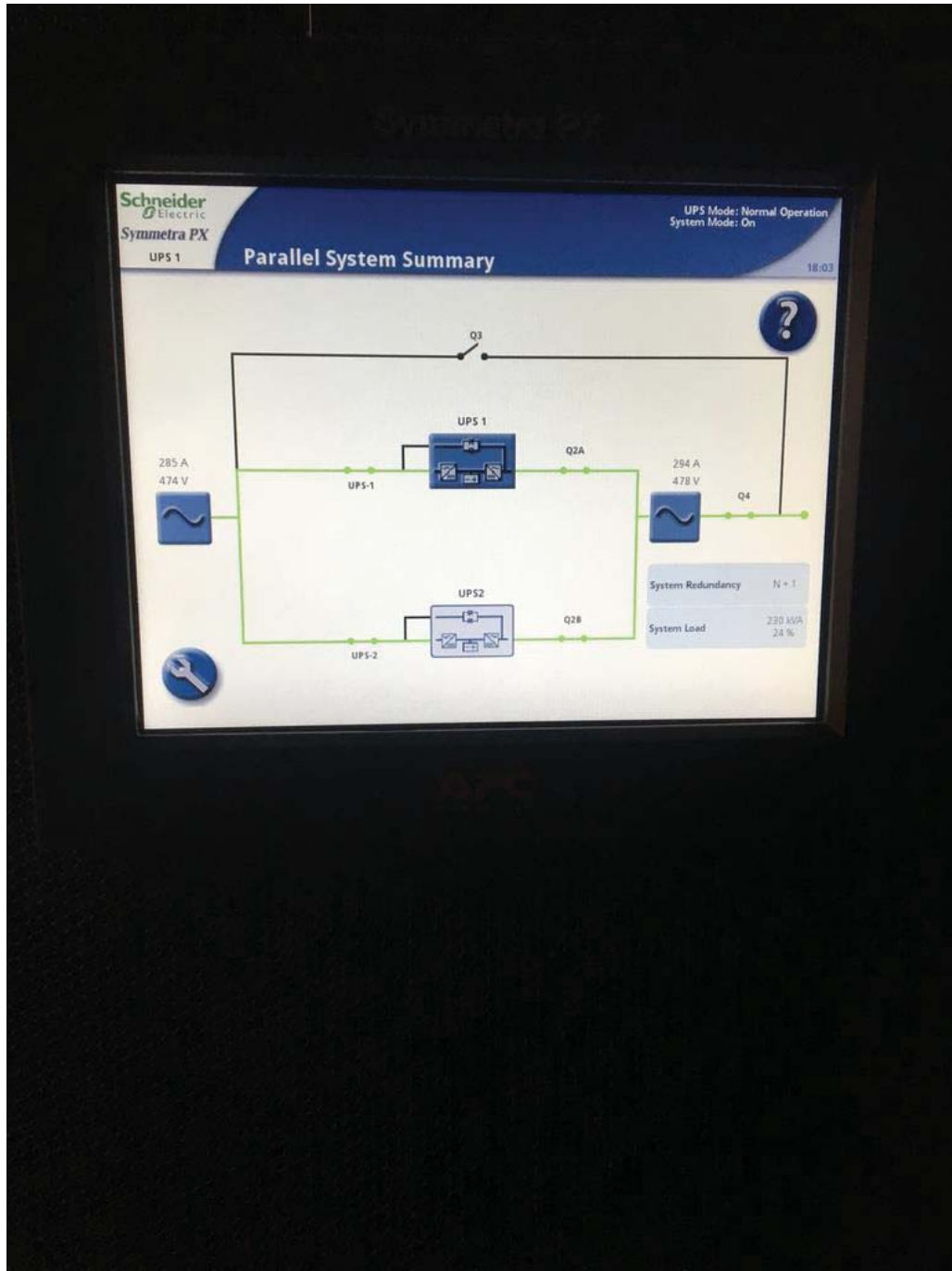
FIGURE 7 – UPS SCHEMA – UPS-1 AND UPS-2 CONNECTED IN PARALLEL
