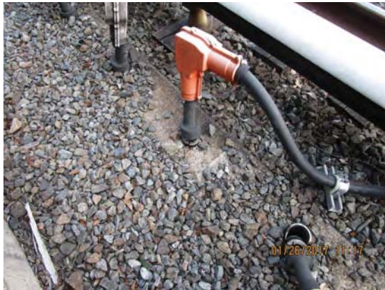
FIGURE 3 - TRK 1 CM 704+00 – HEAT SHRINK NEEDS TO BE REPLACED ON A FEEDER CABLE STUB-UP; GEDNEY BUSHING NEEDS TO BE REPLACED ON ANOTHER FEEDER CABLE STUB-UP
