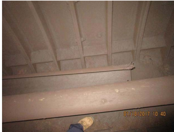
FIGURE 1 - TRK 1 CM 045+00 – 3 RD RAIL COVERBOARD NEEDS TO BE REPLACED
