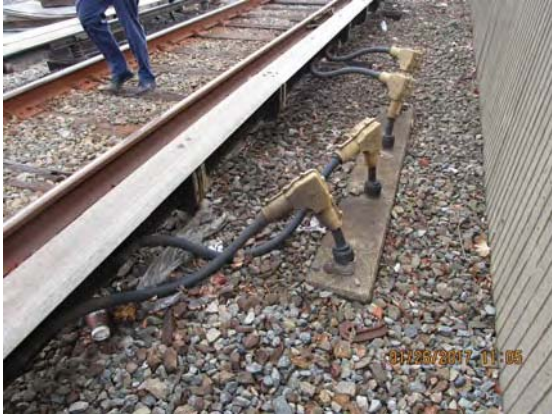
FIGURE 1 - TRK 1 CM 693+00 – FEEDER CABLES LAYING ON THE DECK (BALLAST); HEAT SHRINK AND/OR OZGEDNEY BUSING NEEDS TO BE REPLACED ON FEEDER CABLE STUB-UP
