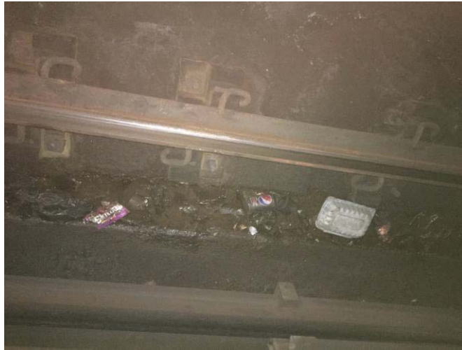
FIGURE 19 - TRK 2 CM 068+00 – TRASH IN DRAIN NEEDS TO BE CLEANED OUT AND 3 RD RAIL COVERBOARD MISSING
