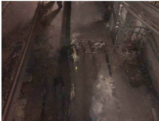
FIGURE 18 - TRK 2 CM 067+00 – WATER INTRUSION IN TUNNEL, LEAKING FROM CEILING
