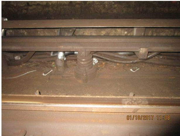
FIGURE 5 - TRK 1 CM 025+00 – TRASH SURROUNDING JUMPER CABLES THAT ARE REPLACING NORMAL FEEDER CABLES DUE TO A TIE BREAKER REHAB. TRASH BY 3 RD RAIL END APPROACH
