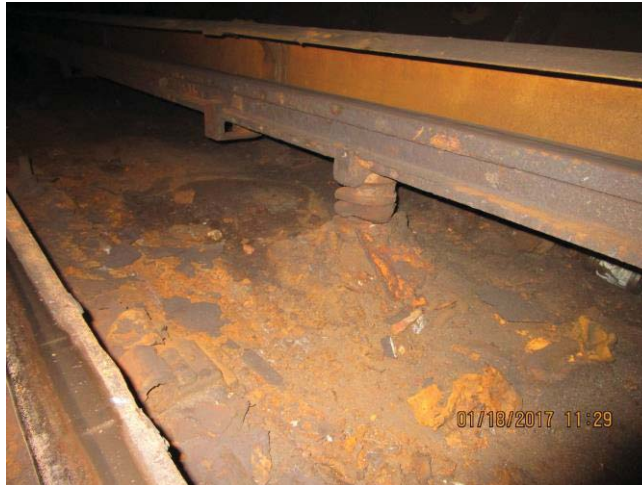
FIGURE 8 - TRK 1 CM 008+00 – 3 RD RAIL POST INSULATOR NEEDS REPLACEMENT
