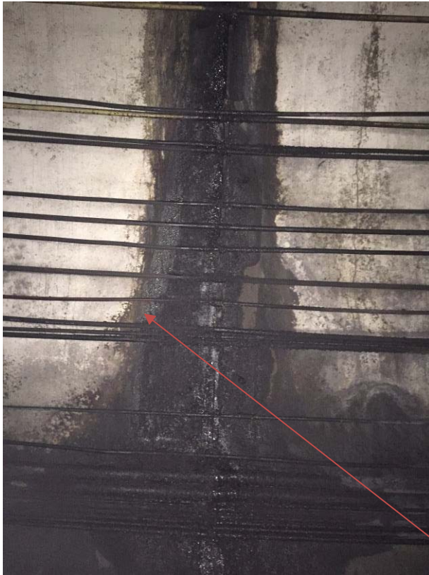
Crack in the side of tunnel allowing
