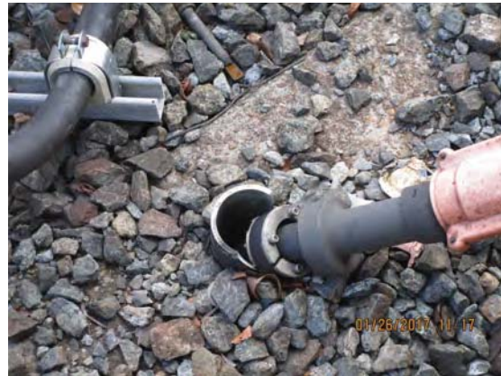
FIGURE 3 - TRK 1 CM 704+00 – HEAT SHRINK NEEDS TO BE REPLACED ON A FEEDER CABLE STUB-UP; GEDNEY BUSHING NEEDS TO BE REPLACED ON ANOTHER FEEDER CABLE STUB-UP
