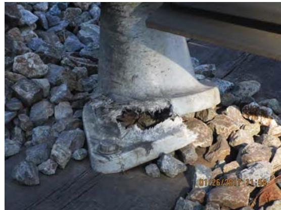
FIGURE 4 - TRK 1 CM 766+00 – 3 RD RAIL POST INSULATOR SUPPORTING THIRD RAIL AS END APPROACH MAY HAVE BEEN SHORTENED; REMOVE UNNECESSARY INSULATOR AS COULD IMPEDE COLLECTOR SHOES OR KNOCK COLLECTOR SHOES OFF TRACK
