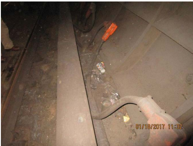
FIGURE 9 - TRK 1 CM 007+00 – DEBRIS SURROUNDING FEEDER CABLES; FEEDER CABLE ORANGE BOOT IN CONTACT WITH METAL TUNNEL STRUCTURE
