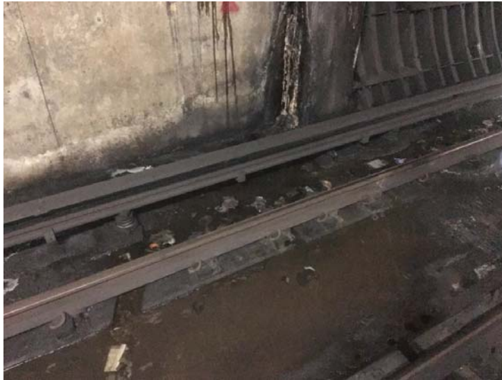
FIGURE 17 - TRK 2 CM 054+00 – TRASH AND WATER IN TUNNEL AREA BY 3 RD RAIL
