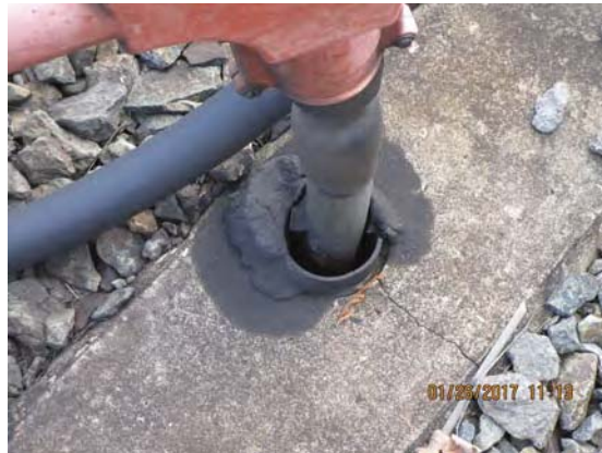
FIGURE 2 - TRK 1 CM 702+00 – OZGEDNEY BUSING NEEDS TO BE REPLACED ON FEEDER CABLE STUB-UP; CABLES LAYING ON THE DECK (BALLAST)
