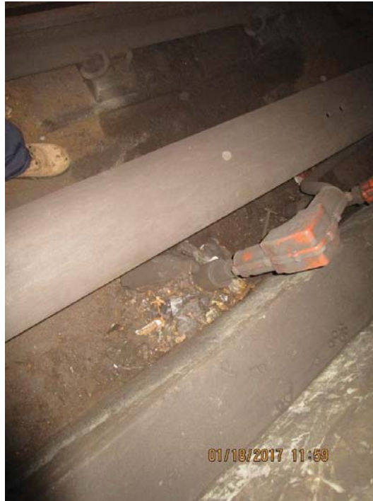
FIGURE 12 - TRK 2 CM 024+00 – DEBRIS SURROUNDING FEEDER CABLES
