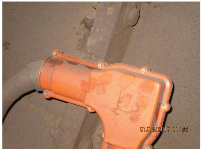
FIGURE 9 - TRK 1 CM 007+00 – DEBRIS SURROUNDING FEEDER CABLES; FEEDER CABLE ORANGE BOOT IN CONTACT WITH METAL TUNNEL STRUCTURE
