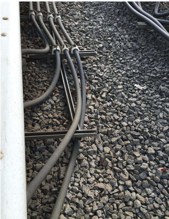
FIGURE 4 – CABLES LYING ON DECK AND MISSING FIBERGLASS STANDOFF(S) WITH KINDORF STRAP(S); LOOSE NUT/BOLT ASSEMBLY ON KINDORF STRAP
