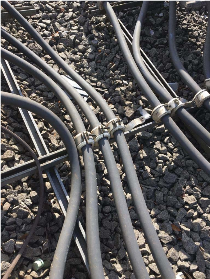
FIGURE 6 – CABLES LYING ON DECK AND MISSING FIBERGLASS STANDOFF(S) WITH KINDORF STRAP(S); LOOSE NUT/BOLT ASSEMBLY ON KINDORF STRAP
