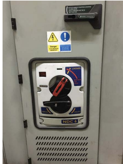
Figure 2 – INDIVIDUAL 750V DC TYPE NDC HIGH SPEED BREAKER
