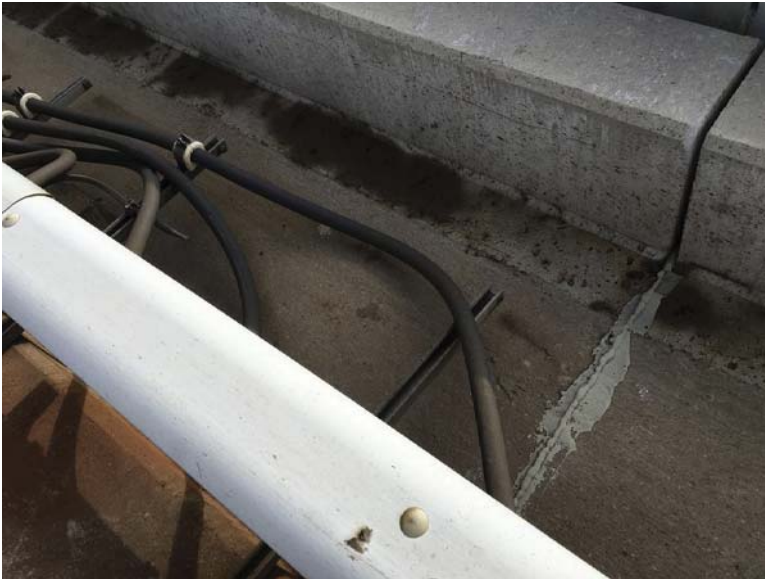
FIGURE 1 – CABLE LYING ON DECK AND MISSING FIBERGLASS STANDOFF WITH KINDORF STRAP
