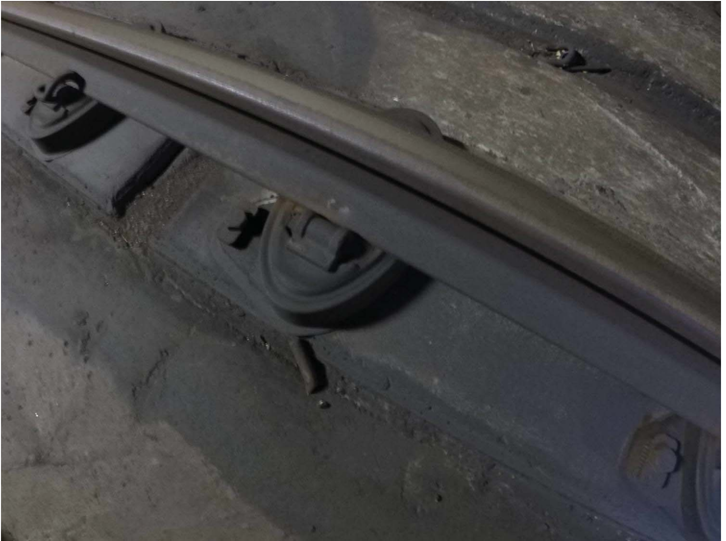
Cologne Egg Fastener with broken e-clip
