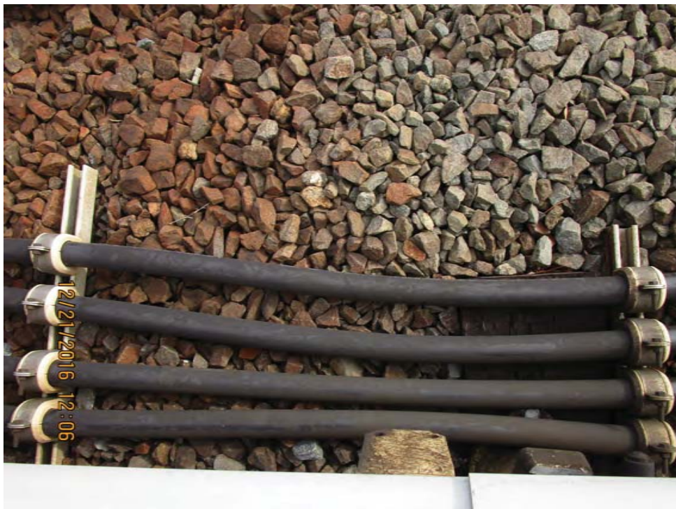
FIGURE 3 - CABLES LAYING ON DECK (BALLAST) f
