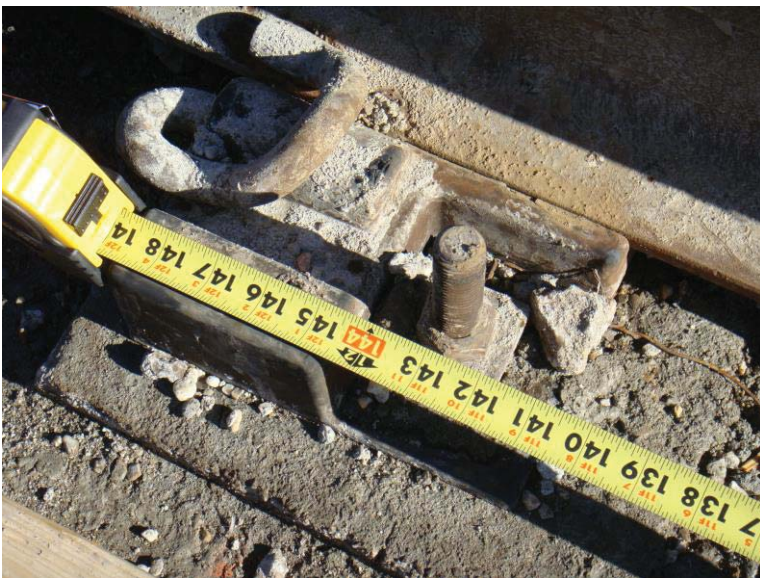
Figure 6 - 144" between effective fasteners at B1 CM174+00
