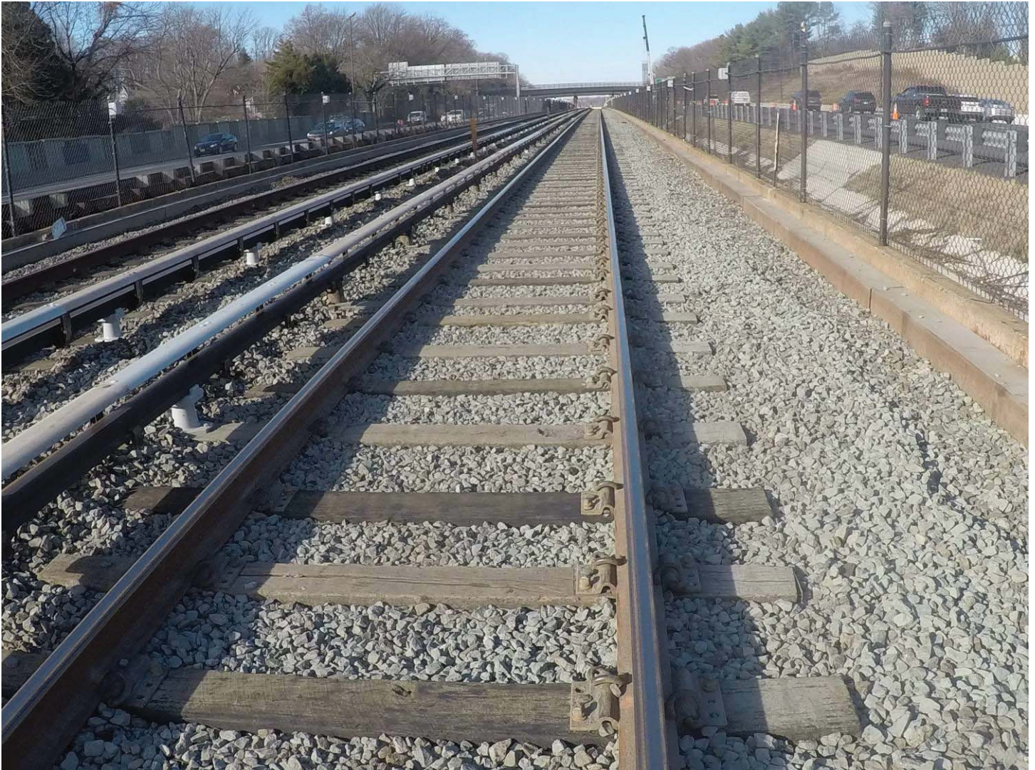
Recently Completed Tie Replacement and Ballast addition and regulation
