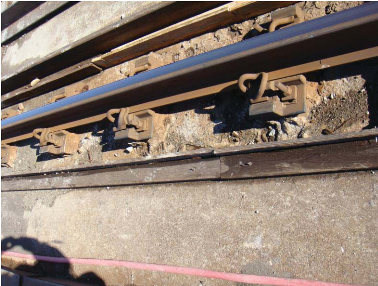
Figure 5 - Grout Pad at B1 CM174+00 left rail scheduled for completion 12/10/16
