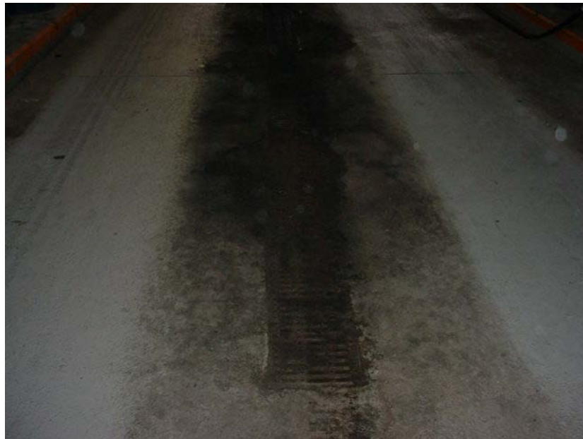
Fuel Alley Trench Drain – Before
