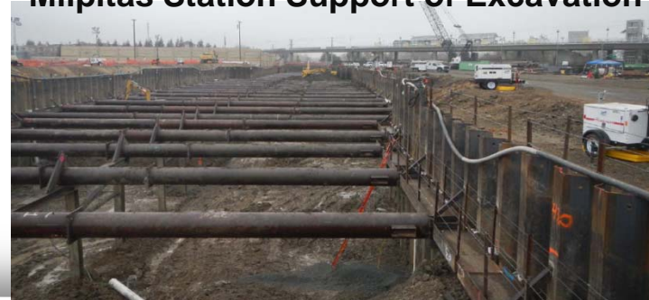
Milpitas Station Support of Excavation
