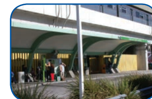
Intermodal Station along Miami-Dade Busway
