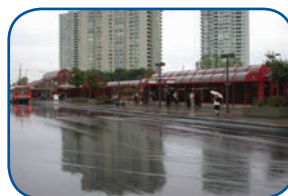
Ottawa Transitway Intermodal Station
