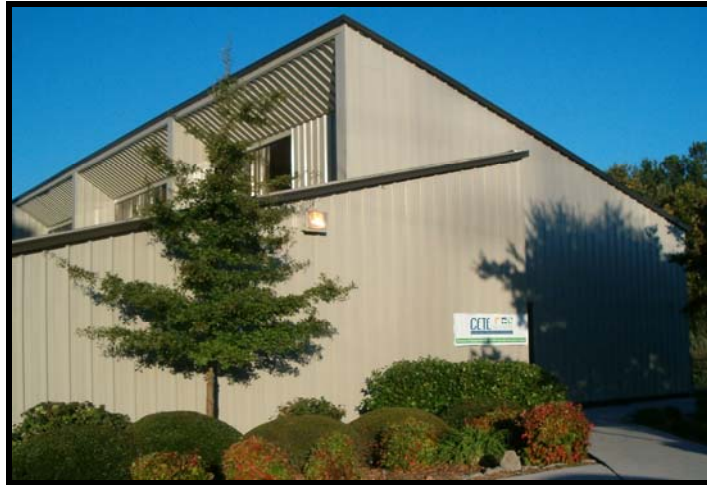
Figure 3. 9,452 Sq. Ft. AVTF Building
