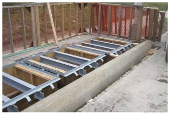
At left: Subway vent wells required covers for Hurricane Irene (August 2011). At right: Vent well and curb rehabilitation project (March 2012) performed to prevent water infiltration into the subway.
