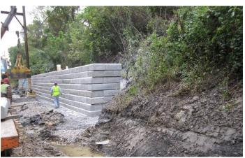
In response to track washouts during Tropical Storm Lee in September 2011 (left), SEPTA constructed a retaining wall (right) to prevent debris from washing onto the West Trenton Line during future storms.
