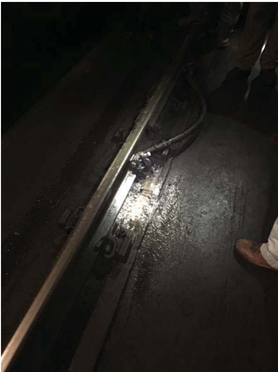
Leak on negative return cables at 360+50
