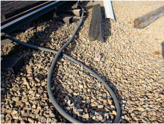
Figure 6 - Jumper Cable on ground CM 540+30 to CM 540+40
