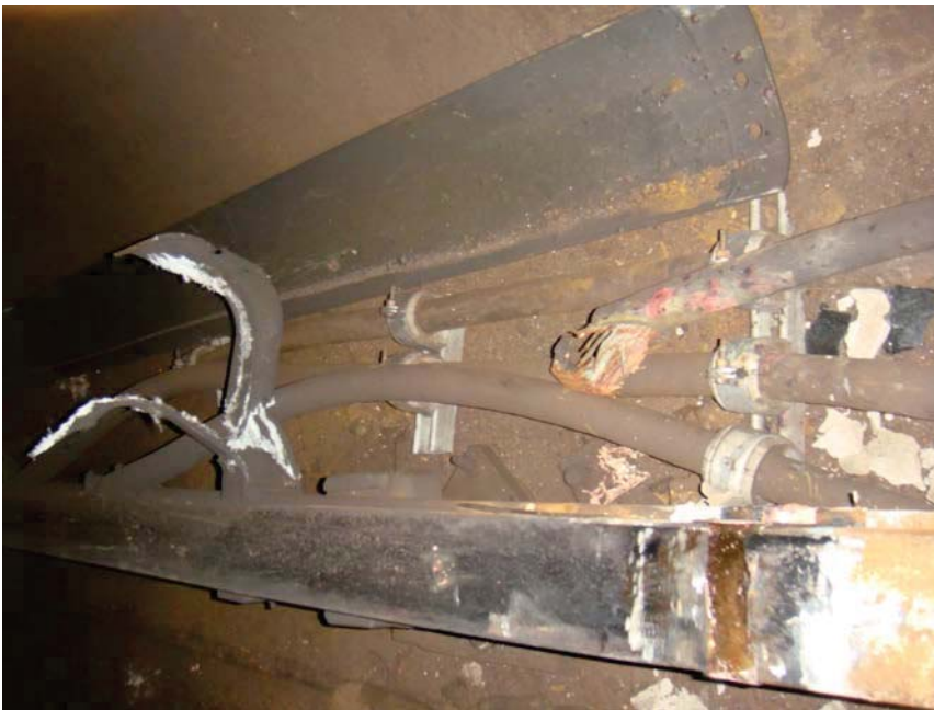
Figure 1 - A1 CM 243+50 - expansion joint elimination. Note the cables still connected and lying on the ground exposed conductors.
