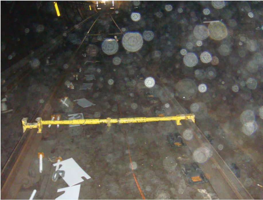
Figure 2 - Ongoing fastener replacement between Friendship Heights (A08) and Bethesda (A09) - Note: White specks are airborne dust from work effort
