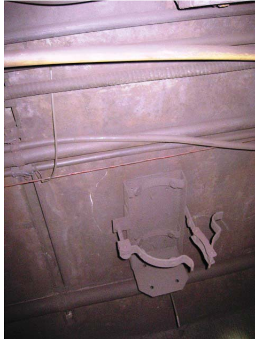
Missing Fire Extinguisher at 342+70
