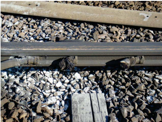
Figure 7 - Jumper cables cut, evidence of fire - CM 579+00 at 3rd rail expansion joint
