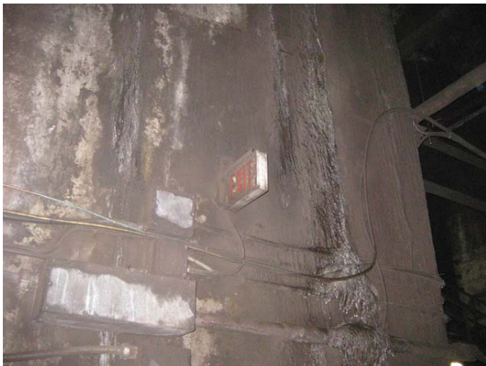
Illegible illuminated EXIT sign at 388+40
