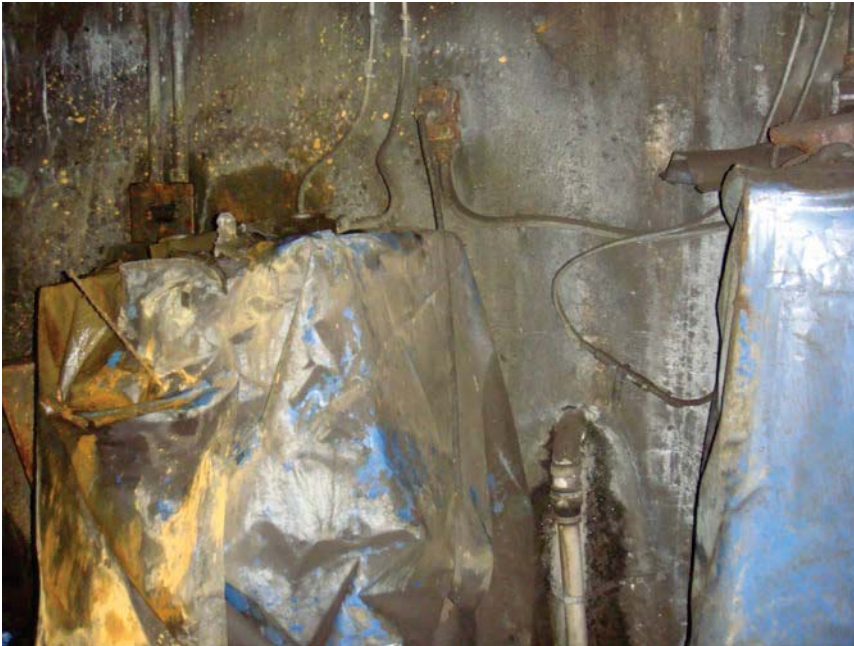
Figure 2 - ANCOM Equipment - note the tarps and water intrusion. These were deactivated in 2015 and scheduled for removal
