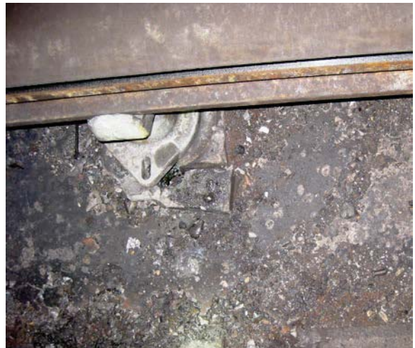
Damaged Invert at CM 79+50
