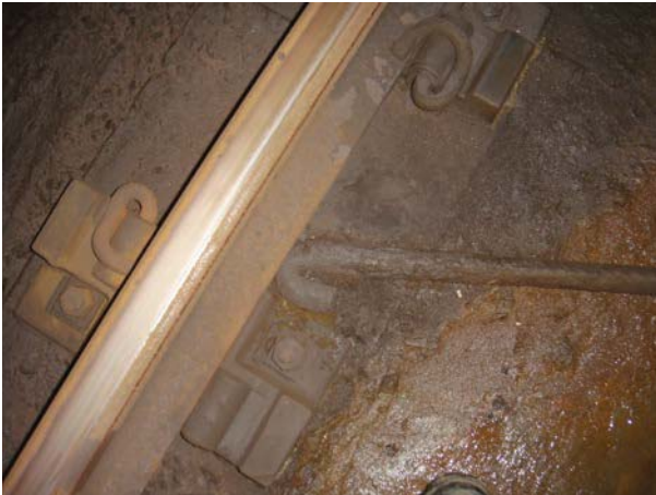
Figure 4 - Gage Rod laying on ground
