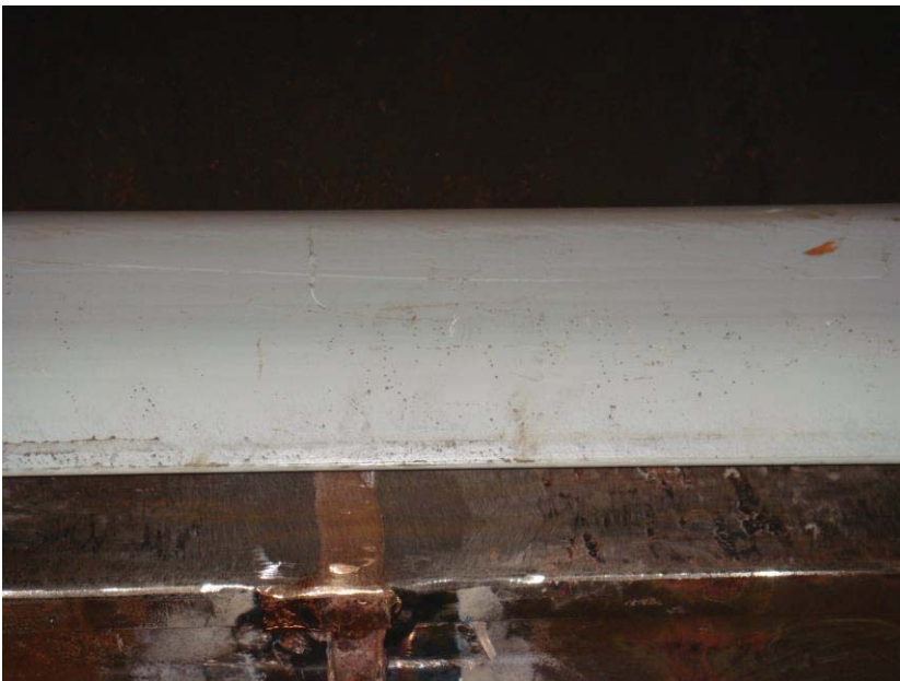
Figure 1 - example of third rail weld where expansion joint was eliminated
