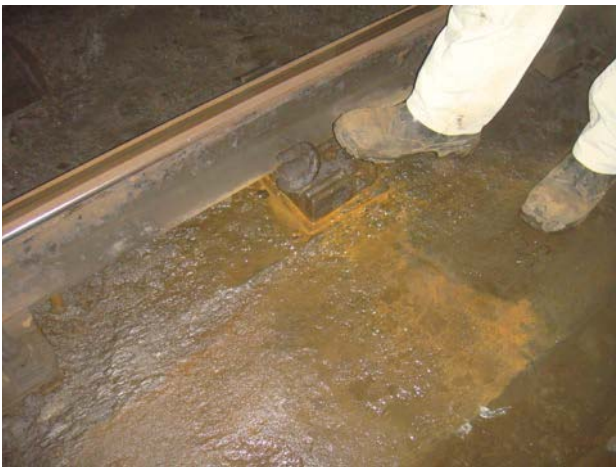
Figure 5 - Example of pumping tie plate with wet conditions
