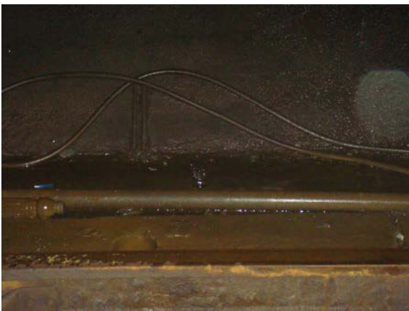
Figure 2 - Switch 1A Standing Water
