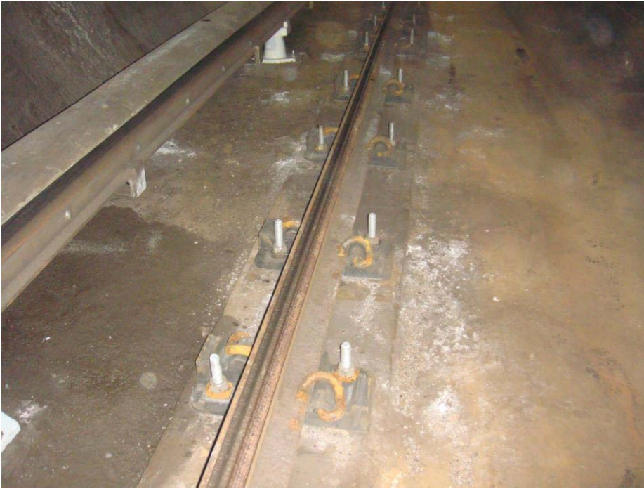
Figure 1 - Fastener Replacement between A1 CM 434+00 and A1 CM 435+00
