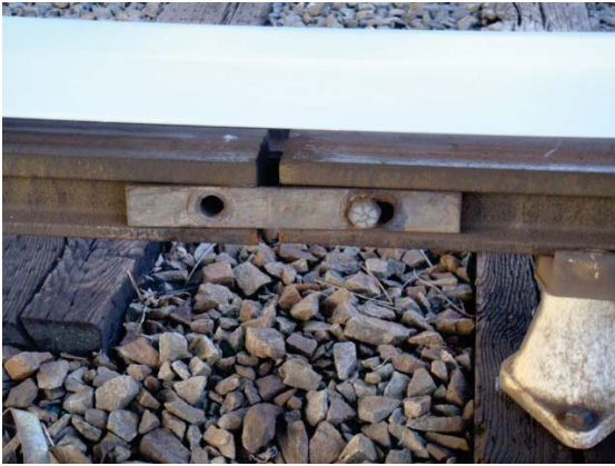
Figure 3 - Missing Bolt - 3rd Rail Joint Bar - CM 518+00
