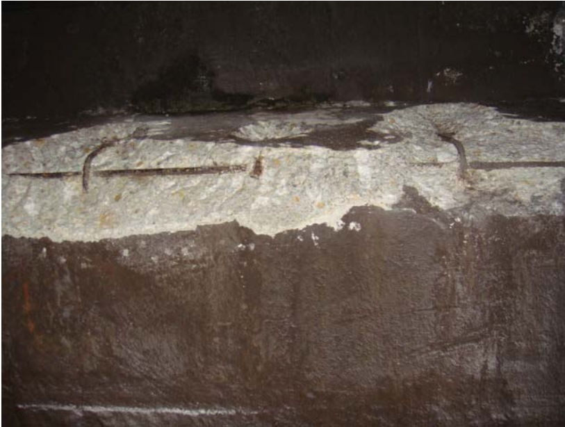
Figure 1 - Catwalk Repairs - prior to completion
