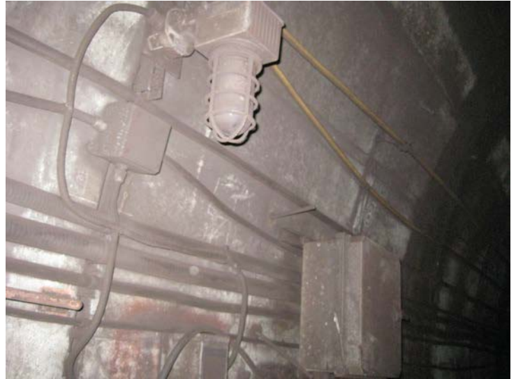
ETS Box Missing Blue Light and Fire Extinguisher 342+80
