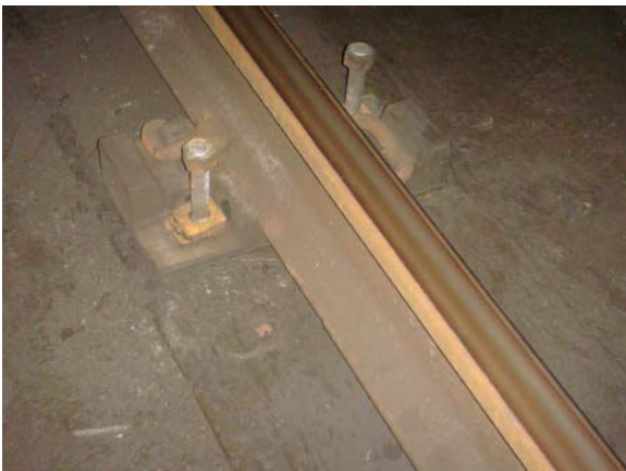
Figure 1 - Switch 1A loose bolts x3
