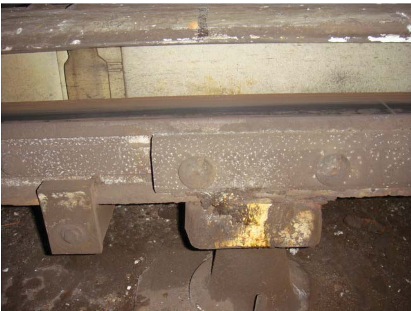
Figure 4 - Insulator at A1 CM 422+30 - appears to be arcing
