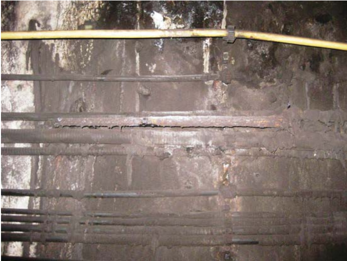
Decayed/Rusted Grab Bar 343+20
