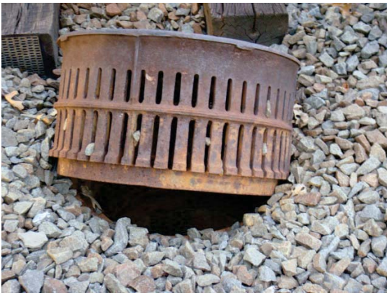
Figure 4 - Manhole Drain Cover Dislodged - CM 518+00
