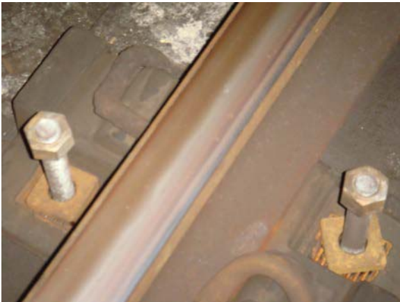
Figure 1 - Switch 1A loose bolts x3
