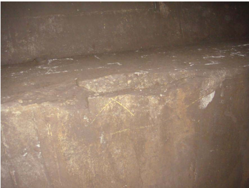
Figure 2 - Concrete Spalling - A1 413+60
