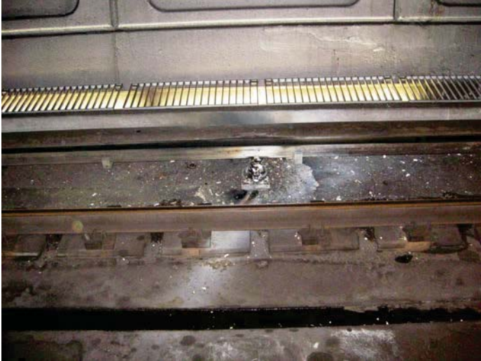
Repaired incident insulator (far left)
