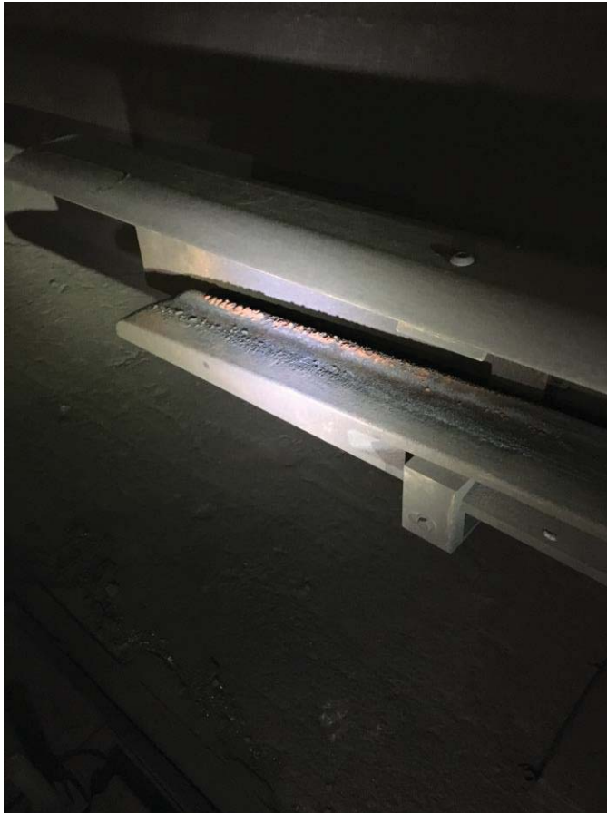
Removed 3 rd rail expansion
