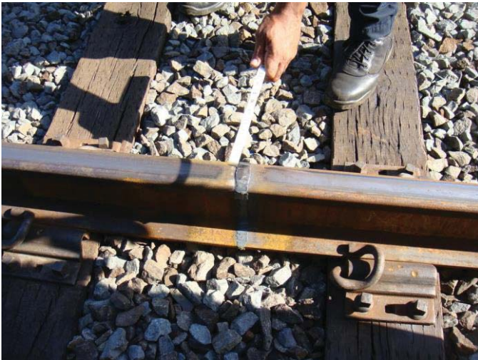
Figure 5 - K1 CM 329+00 - Mismatched rail ends - unfinished weld
