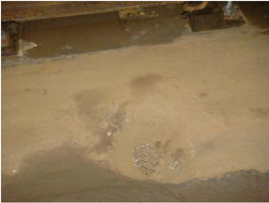
Figure 1 - New Screen but down approximately 4-inches below grade - multiple locations
