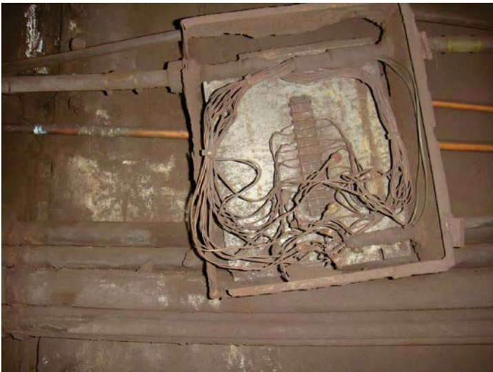
Figure 2 - A2 CM381+50 - communication splice box rotted with exposed wires
