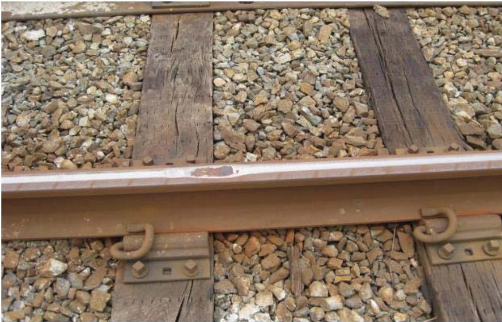
A2-515+80- Severe rail surface defects (spalling) from vertical track deflection (Location- wood tie transition to DF aerial transition)
