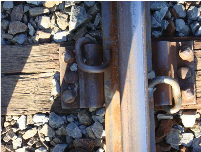
Figure 7 - Tie plate configuration on existing ties - note 4 screw spikes and 2 cuts spikes
