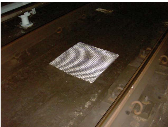
Figure 2 - Example of Drain cover that protects from trip and falls
