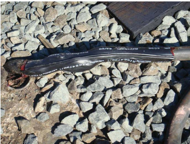
Figure 3 - K1 CM 336+90 - third rail return cable with shrink wrap - requesting engineering check
