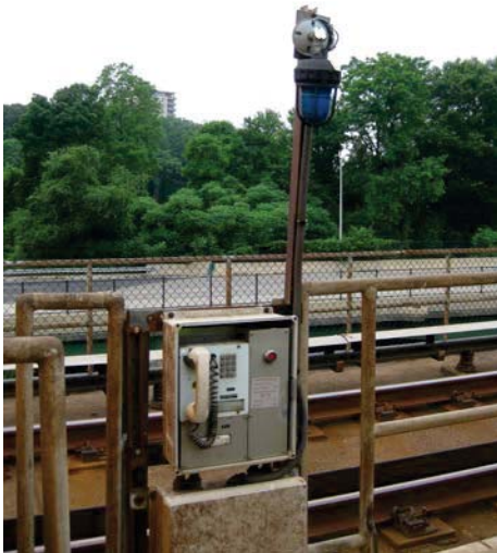
Non-functional ETS box @ CM A2 523+40 No blue lantern.
