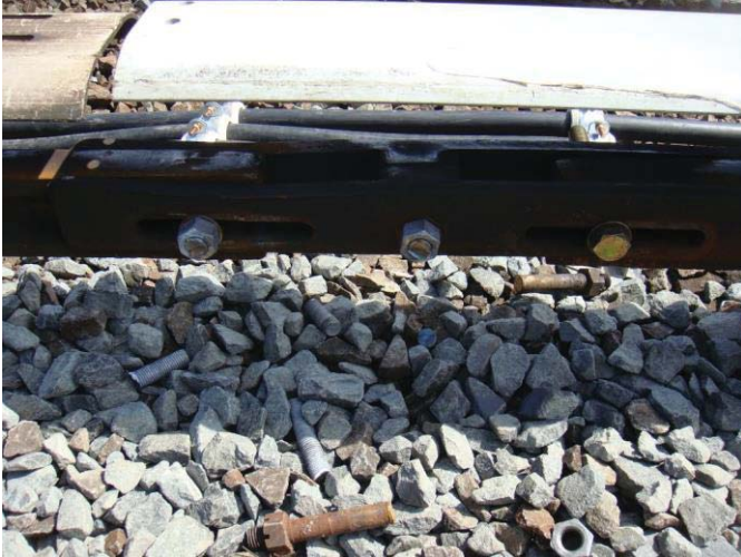
Figure 2 - K1 CM 392+10 - incorrect bolts in the third rail expansion joint
