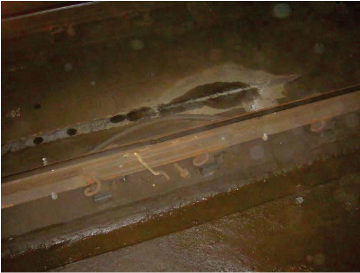
Figure 3 - A2 CM361+35 - Broken bolt in joint bar
