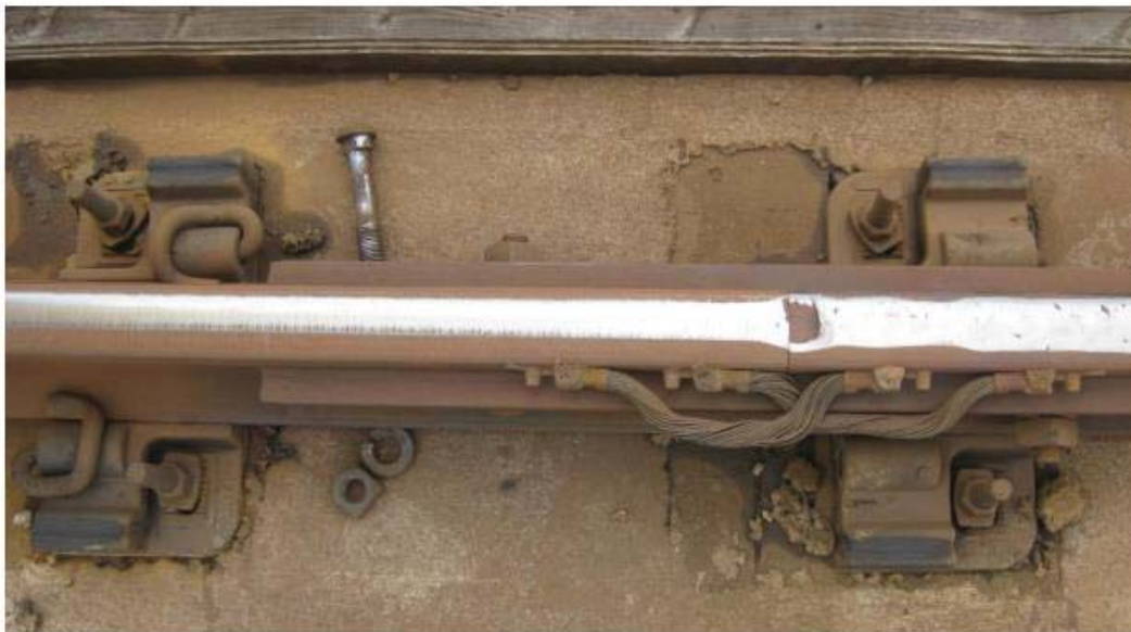
A2-537+50 LR- Suspended rail joint with missing bolt in rail end (this is a 4- bolted suspended joint, where 1- bolt is only holding at one rail end- there is also a rail head surface defect at the joint causing severe pounding to the DF aerial structure)
