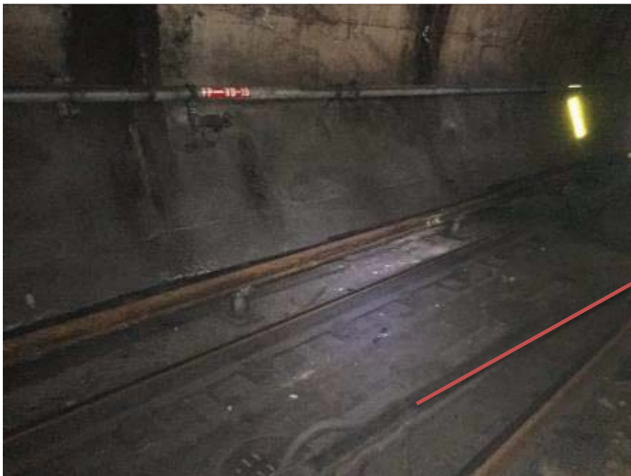
Removed 3 rd rail expansion
