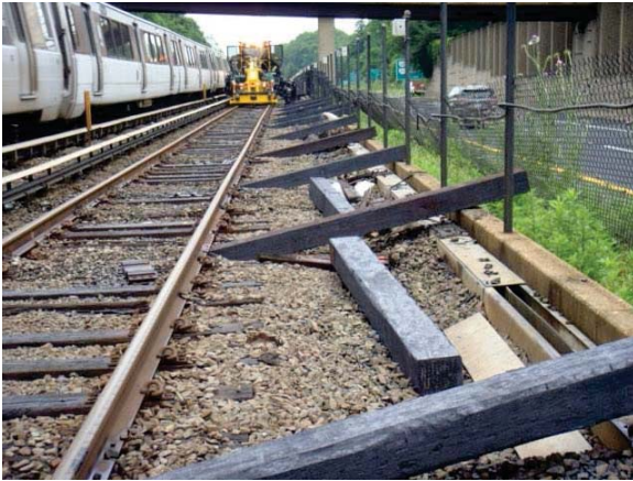
Figure 1 - Ties ready for insertion
