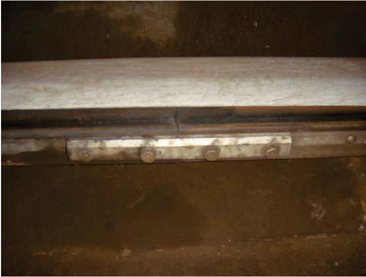
Figure 1 - A2 CM384+70 - eliminated third rail expansion joint - incorrect hardware
