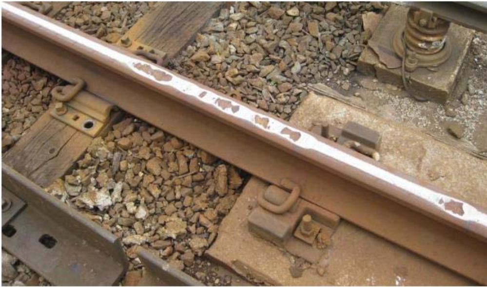
A2-516+00 LR- Severe rail surface defects (spalling) from vertical track deflection (Location-wood tie transition to DF aerial transition)
