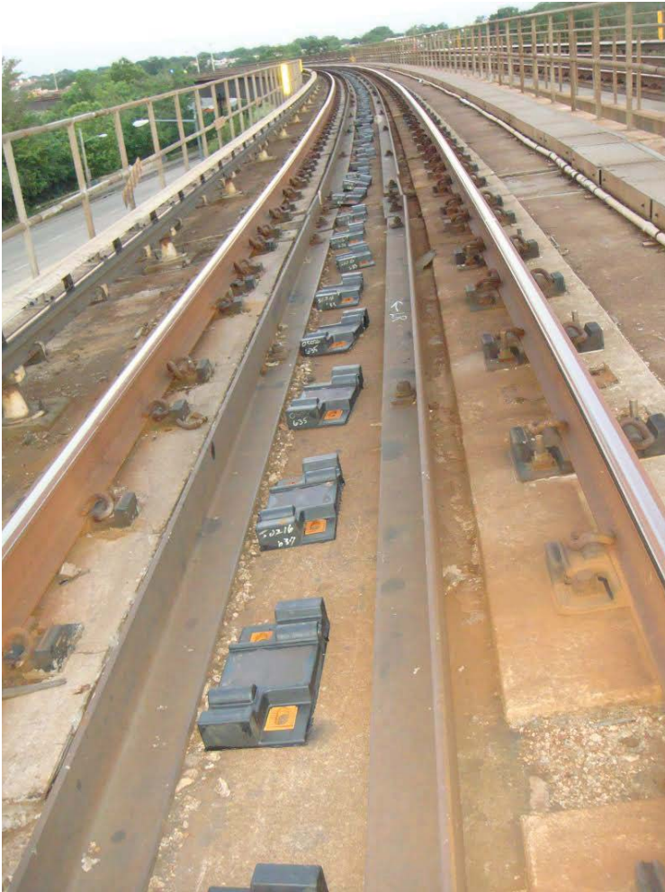
Figure 2 - New Fasteners ready for installation - track 1
