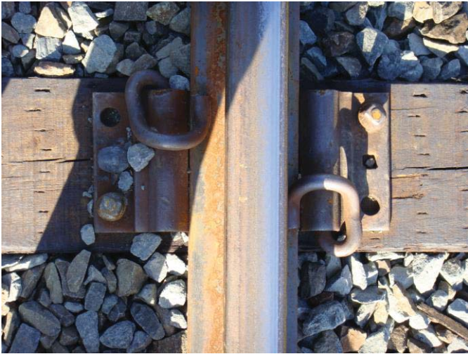
Figure 6 - Tie Plate Configuration - note two screw spikes and one cut spike
