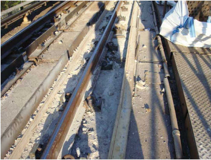
Figure 2 - New Grout Pads formed and awaiting concrete pour
