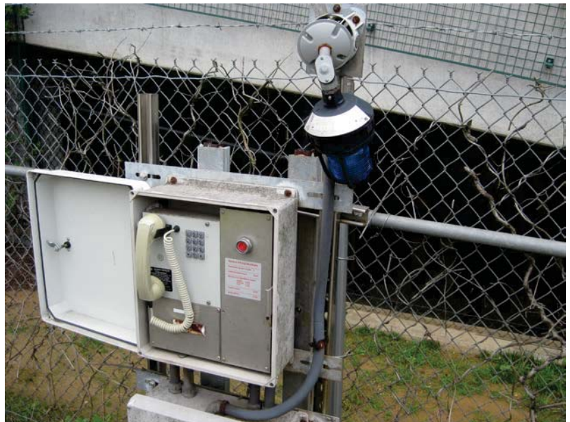
Although ETS is functional, lantern is OOS & full of water @ CM A2 558+80 (adjacent to the Parking Structure)
