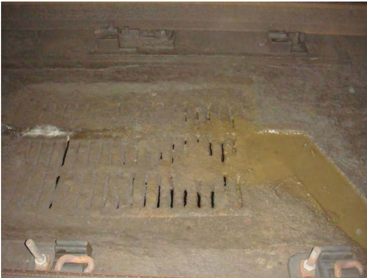
Figure 1 - A1 CM 381+00 - drain cover fouled with mud - similar conditions at other noted drains covers
