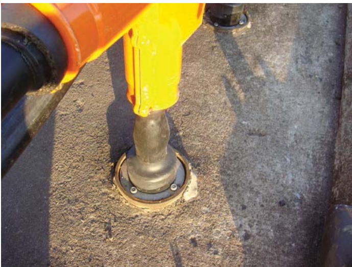
Figure 1 - New Third Rail Stub-up cables - note the shrink sleeves covering the ducts
