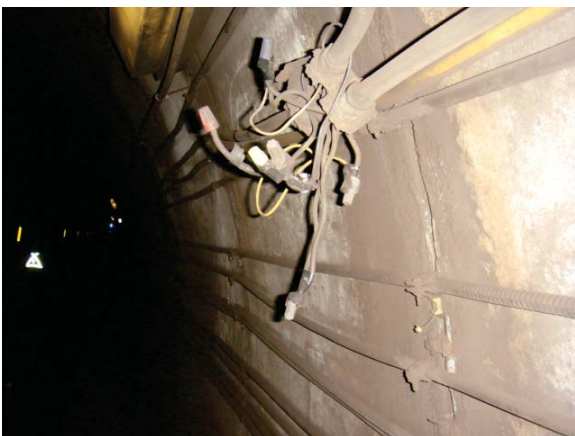
Figure 3 - Exposed wiring feed to florescent fixture
