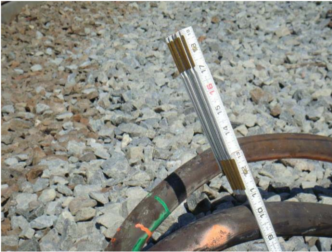
Figure 4 - K1 CM 371+00 - 10" high return cables on field side of rail
