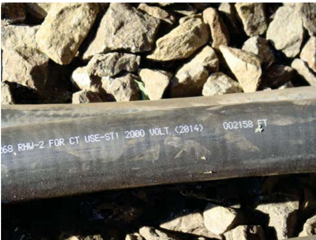
Figure 3 - Cable used to replace expansion joint jumpers - #2
