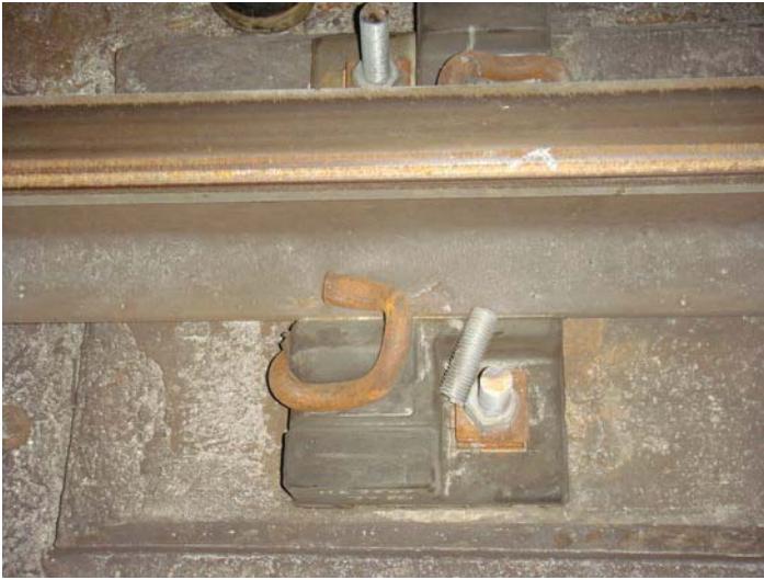
Figure 4 - Long Stud Bolts – evidence of cut bolts, both sides of fastener
