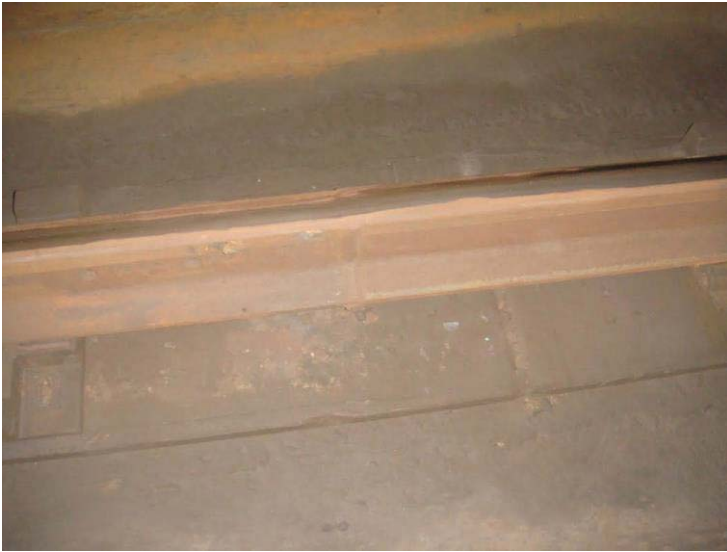
Figure 2 - A1 CM 349+00 - unsupported joint
