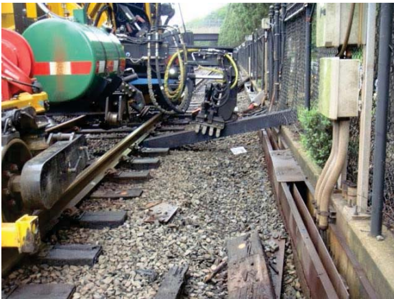
Figure 2 - Ties being inserted
