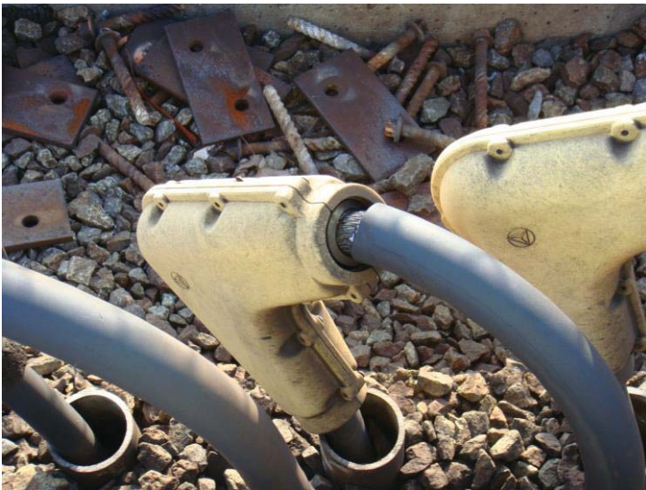
Figure 3 - C1 CM354+80 exposed third rail boot, no sleeves
