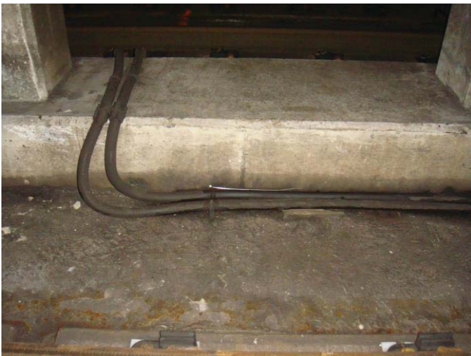
Figure 1 - Unsupported third rail return cable
