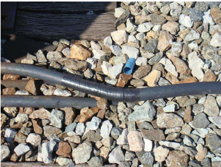
Figure 1 - Taped 3rd rail return cable at D1 CM313+20
