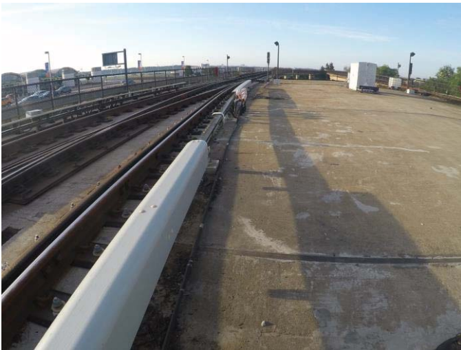
Figure 4 - Missing cover boards CM371+00 track 1 & 2
