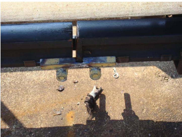
Figure 2 - CM308+00 and CM307+75 Track 1&2 - 3rd rail incomplete weld
