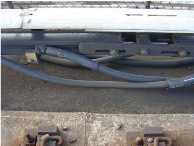
Figure 4 - C1 CM391+60 - 3rd Rail expansion joint cable with electrical tape
