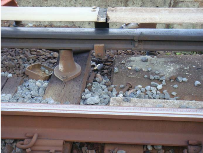
Figure 1 - C2 CM407+90 - Broken insulator - 3rd rail joint
