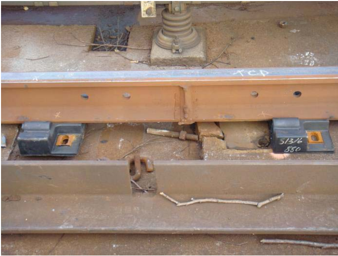
Figure 3 - C2 CM376+30 - Right Rail Support - deteriorated grout pad
