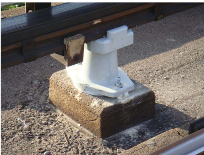
Figure 2 - Incorrect shim - C1 CM377+00 (Noted in other areas as well)
