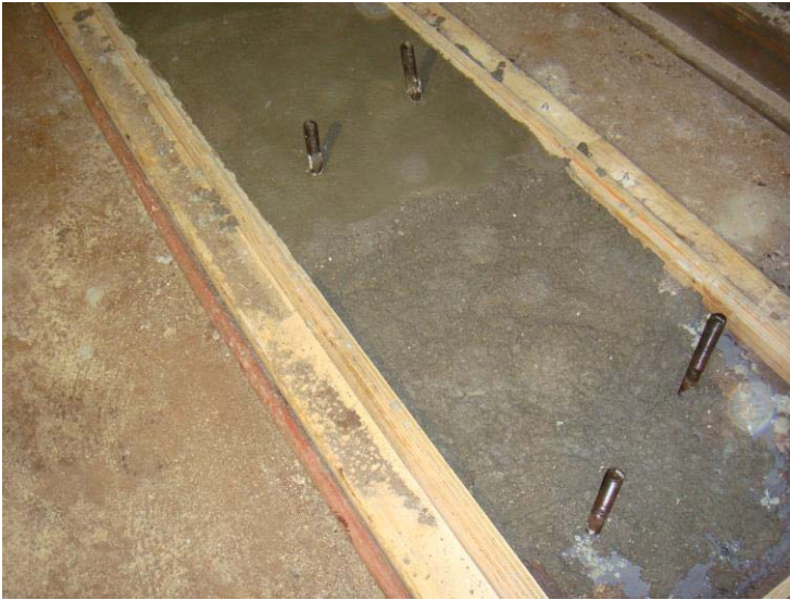
Figure 2 - New grout pad
