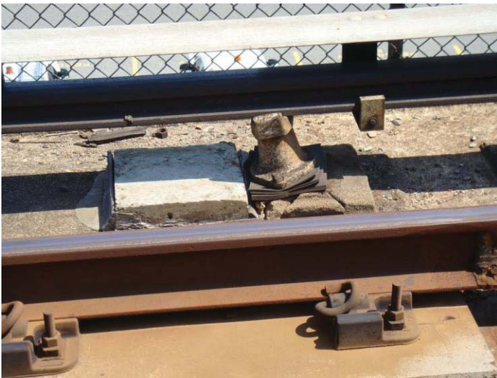
Figure 4 - D2 CM296+40 - New grout pad adjacent to crumbled one
