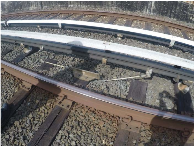
Figure 6 - Third rail anchor not attached - C1 CM417+00 and C1 CM475+00
