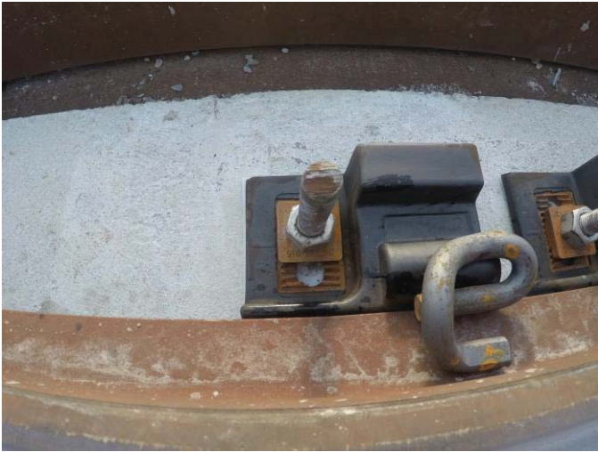
Figure 5 - Stud bolt in excess of 3" above base of rail - signs of having been cut
