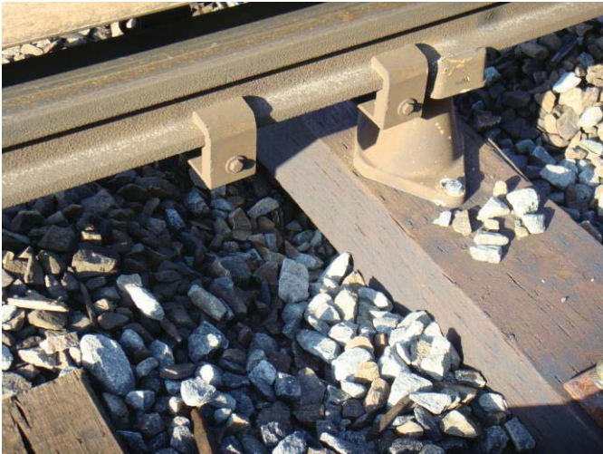
Figure 3 - No ballast support under third rail ties
