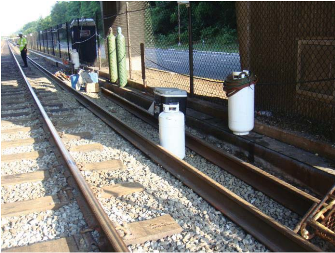
Figure 4 - Un-secure CGC Cylinders adjacent to Rt. 66
