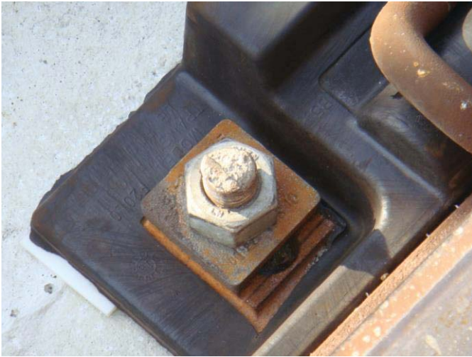
Figure 3 - Ground off stud bolts - observed throughout the new grout pad area from CM376+00 - CM379+00
