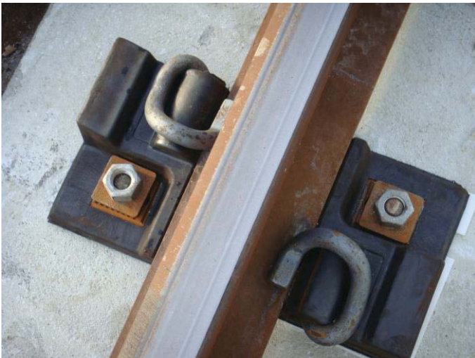
Figure 1 - short stud bolts securing fastener. Also noted stud bolts in excess of 3-inches above base of rail. CM376+00 through CM379+00
