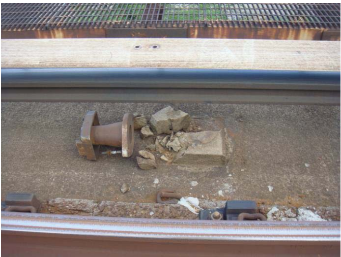
Figure 2 - C2 CM406+60 - broken insulator grout pad
