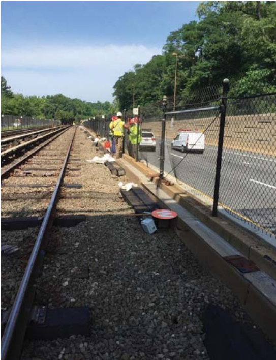
Figure 1 - TRST personnel working on exterior wayside fence adjacent to travel lane of route 66
