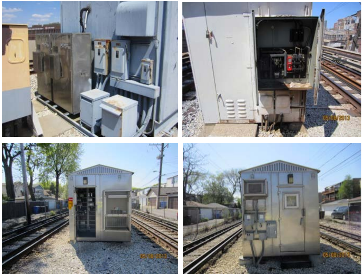
Figure 2-8 Examples of Signal Houses: Orange Line Pulaski Station (top left), Red Line Bryn Mawr Station (top right), Brown Line Rockwell Station (bottom left), Brown Line Sacramento Station (bottom right)
