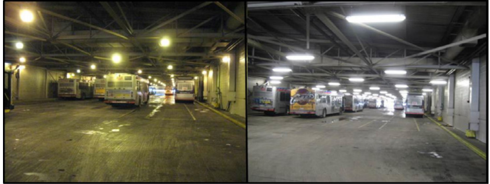
Figure 8-7 Lighting in Hayden Bus Garage Before (left) and After (right) Retrofit
