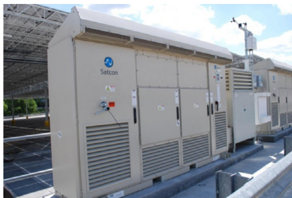
Figure 8-15 MARTA Solar Canopy Feeds Power Into Two Inverters
