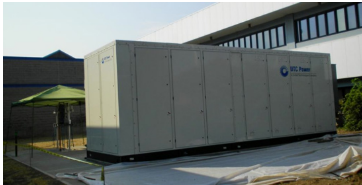
Figure 7-2 Stationary Fuel Cell during Installation at CTTRANSIT
