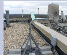
Rooftop wireless cameras in Rockville, MD, focus on track and metro stations to detect safety and security incidents.
