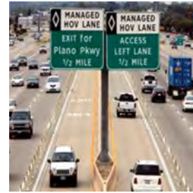
C. Roadway lanes for exclusive use by high occupancy vehicles (HOV) and separated from traffic by physical barriers
