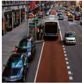
B. Exclusive busway separated from traffic by painted line
