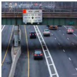
D. Roadway lanes for exclusive use by HOV and separated from traffic by painted lines
