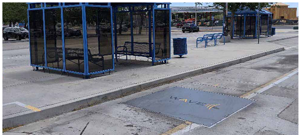
Figure 2-1. WAVE Inductive Charging System, Source: Bryan Lee, CALSTART
