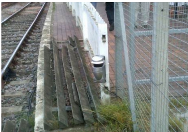
Figure 2-4 Trespasser Detection – Track Surveillance with Laser Beam in UK
